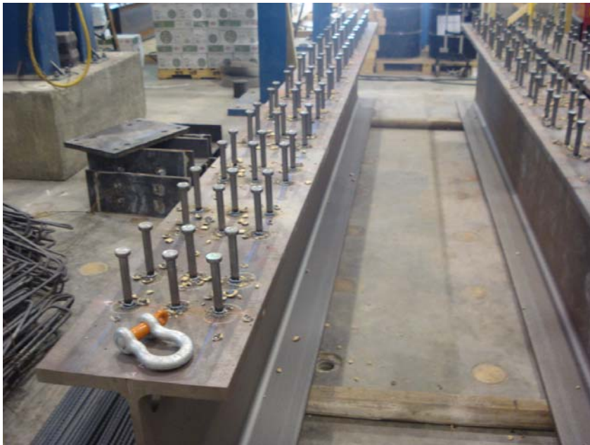
Figure 4-8b: Completed Shear Connector Configuration before Cleanup
