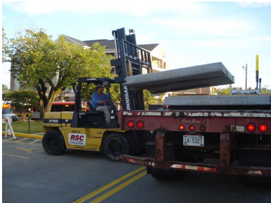
Figure 4-21: Deck Panel Offloading Using Forklift
