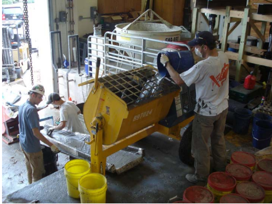
Figure 4-30: Grout Mixing Station
