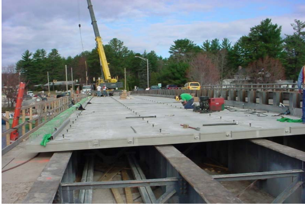
Figure 2-3: Full-Depth Deck Panel System (Culmo 2011)
