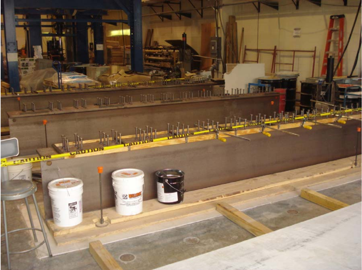
Figure 4-20: Girder Configuration Prior to Deck Panel Placement
