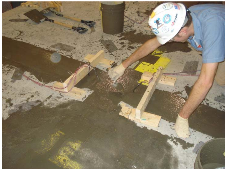
Figure 4-35: Final Leveling and Finishing of Grout Installation
