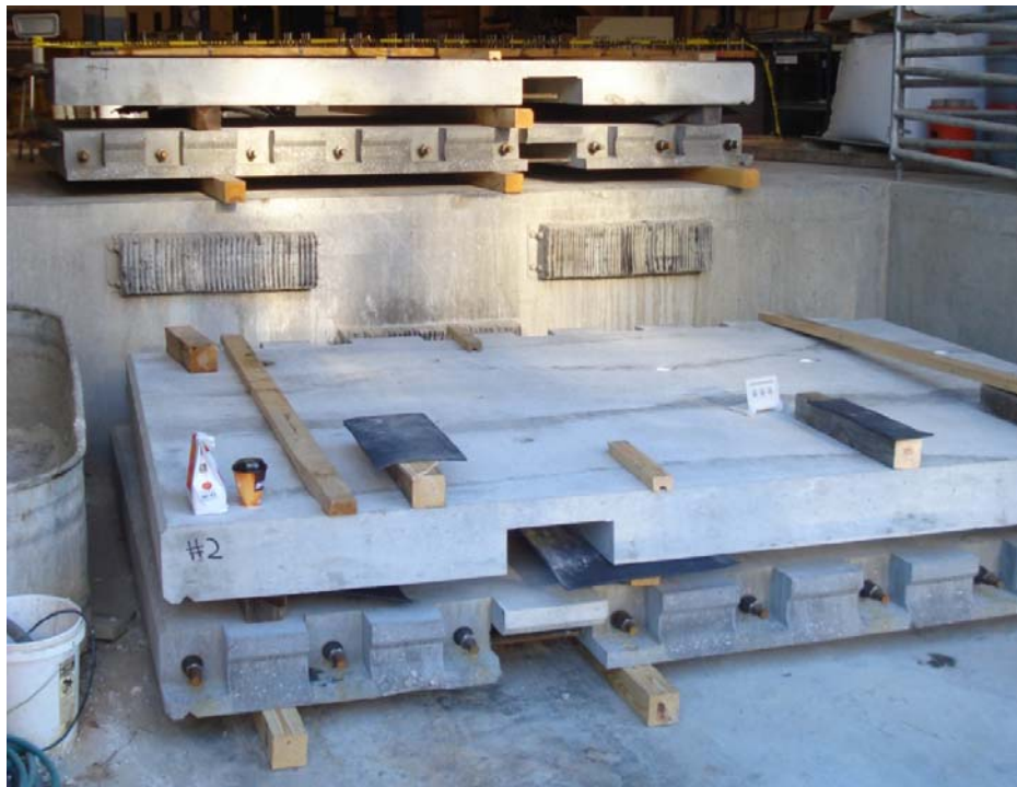
Figure 4-22: Offloaded Deck Panels
