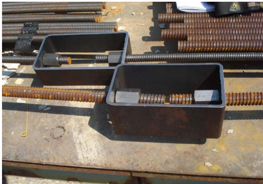
Figure 4-3: Test Fit of HSS Coupler: Staged Construction (left) and Transverse (right) Side Elevation
