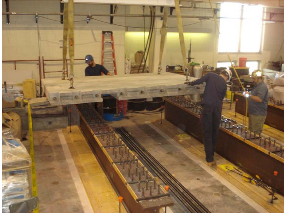
Figure 4-24: Positioning of Typical Deck Panel
