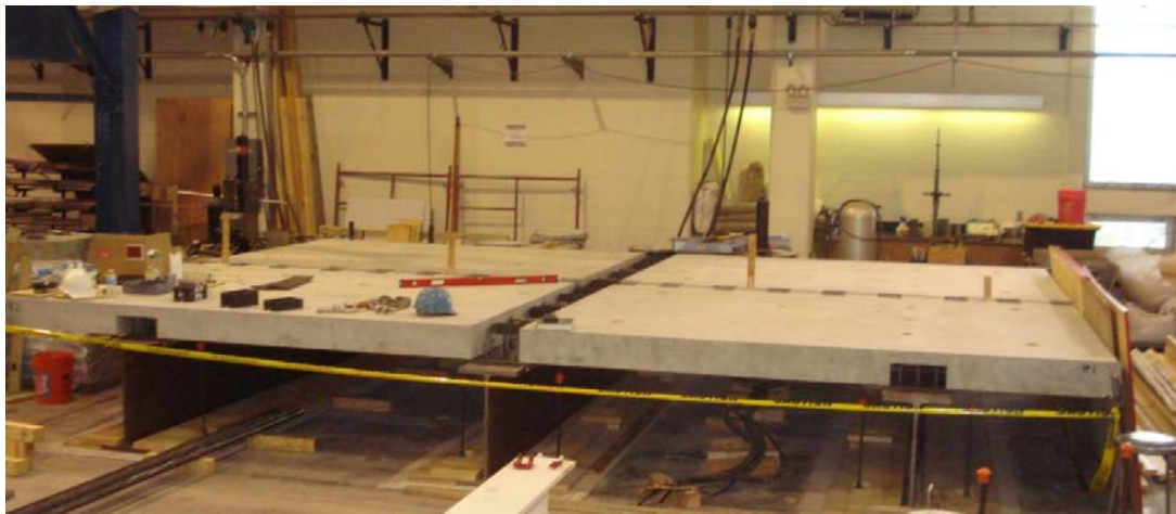
Figure 4-25: Test Deck Specimen after Panel Placement
