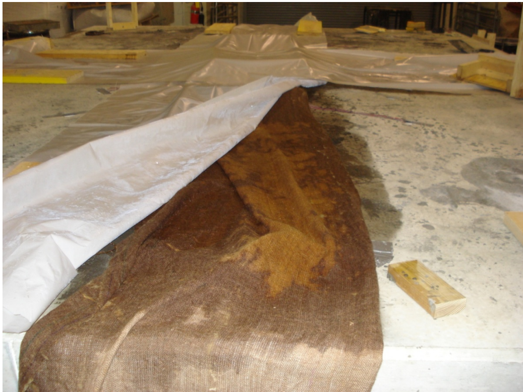
Figure 4-36: Moist Curing of Grouted Joints
