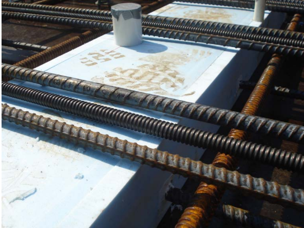
Figure 4-13: Continuous Shear Pocket Formwork
