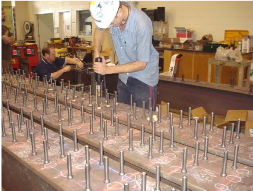
Figure 4-8a: Shear Connector Welding Process
