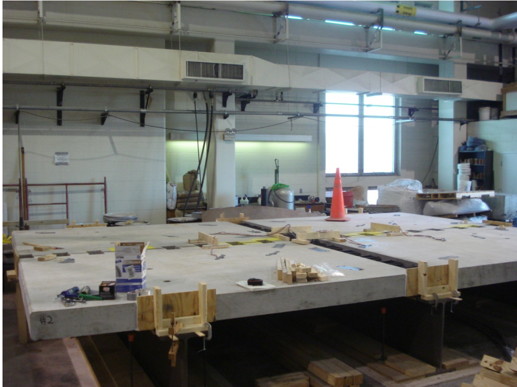
Figure 4-29: Formwork Prior to Grout Installation
