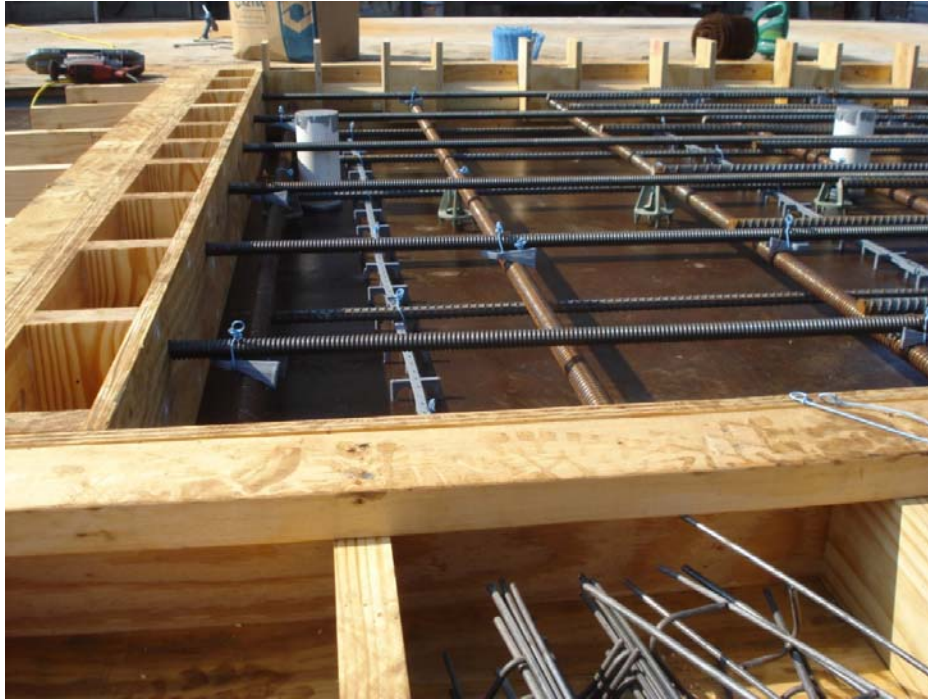
Figure 4-11: Formwork for Staged Construction Joint
