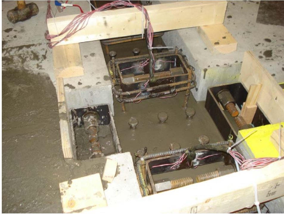
Figure 4-34: Grout Installation at the Panel-to-Panel Joint Intersection
