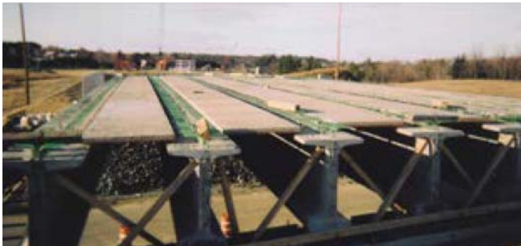
Figure 2-2: Partial-Depth Deck System (Culmo 2011)
