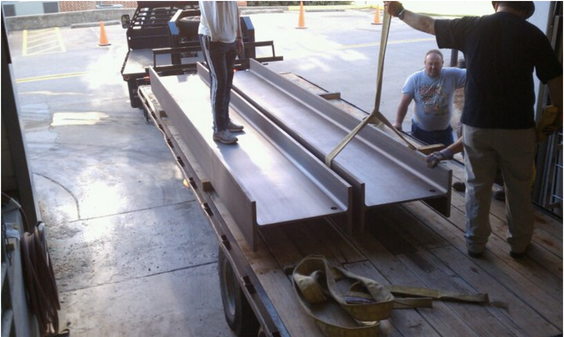
Figure 4-1: Delivery of Steel Girders
