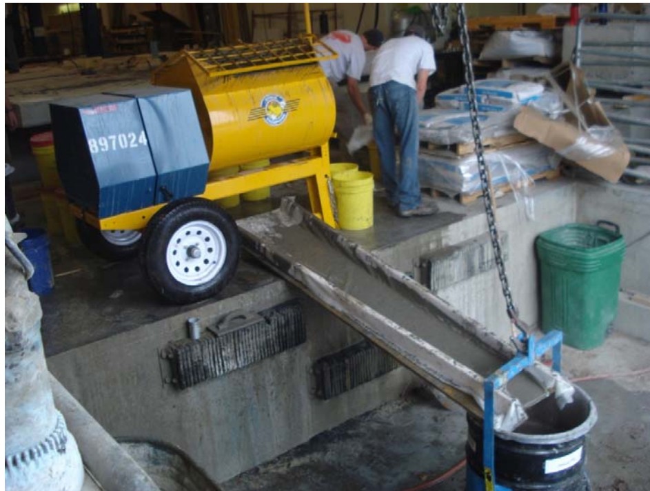
Figure 4-31: Dispensing Grout into Overhead Bucket
