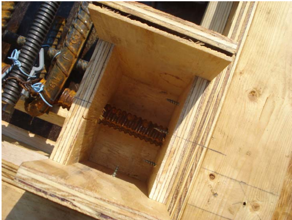
Figure 4-12: Formwork for Transverse Joint
