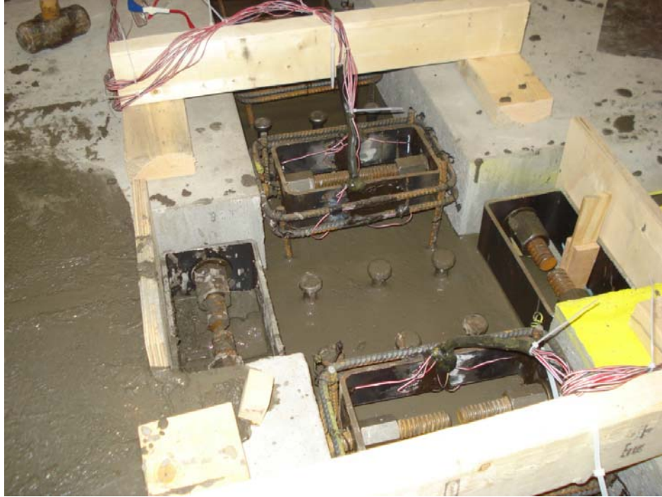
Figure 5-8: HSS Coupler Instrumentation at Staged Construction Joint
