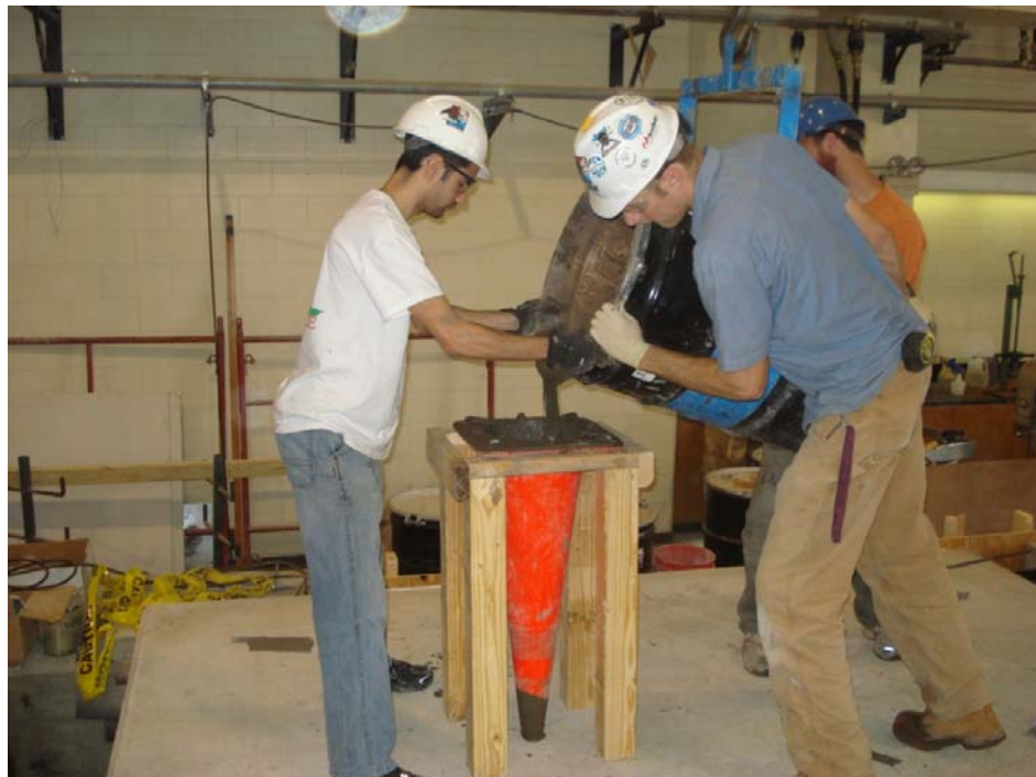
Figure 4-33: Grout Installation into Longitudinal Joint through Injection Port
