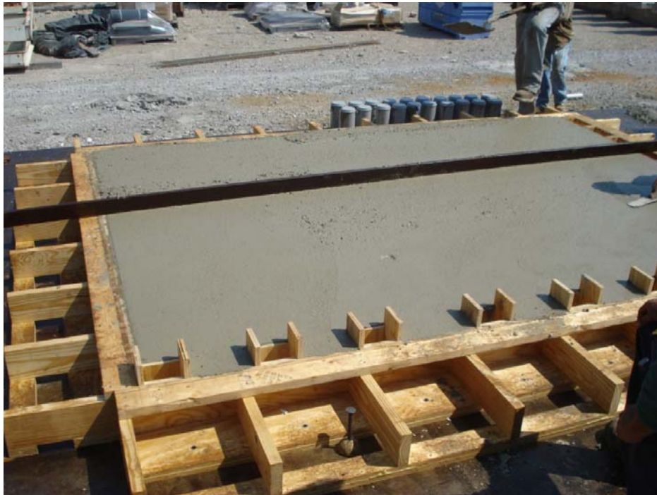
Figure 4-15: Finishing of Panel Surface
