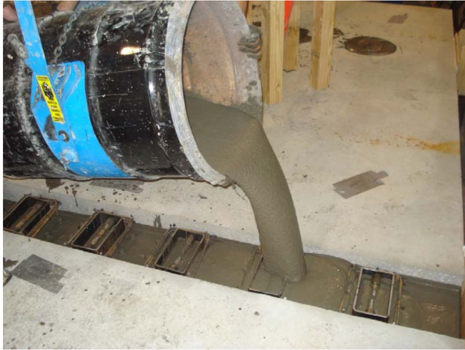
Figure 4-32: Grout Installation into Staged Construction Joint
