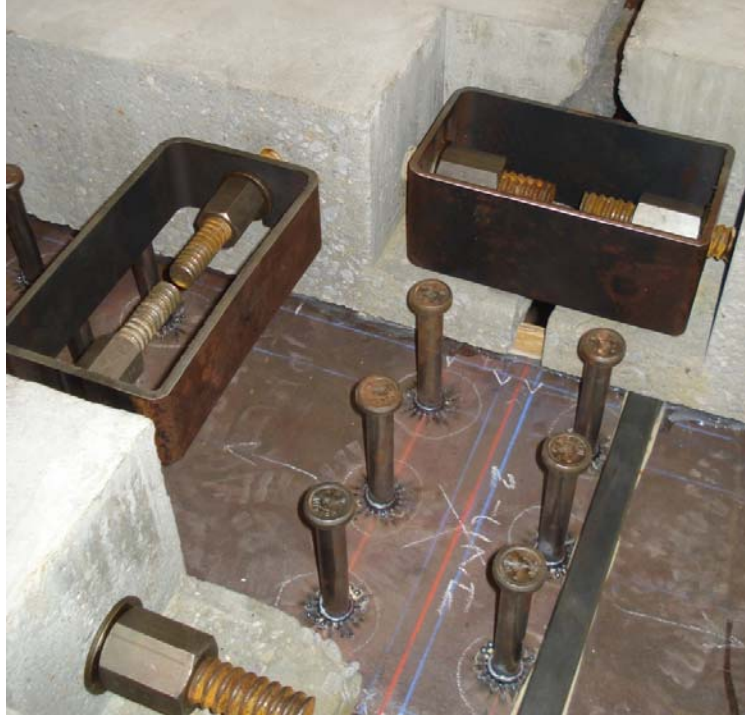
Figure 4-26: Initial Panel-to-Panel Connections
