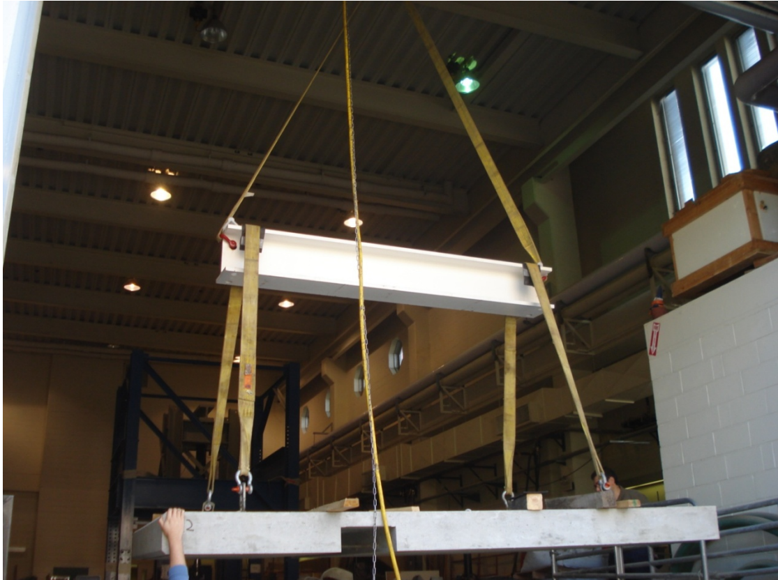
Figure 4-23: Deck Panel Lifting Configuration Including Spreader Beam
