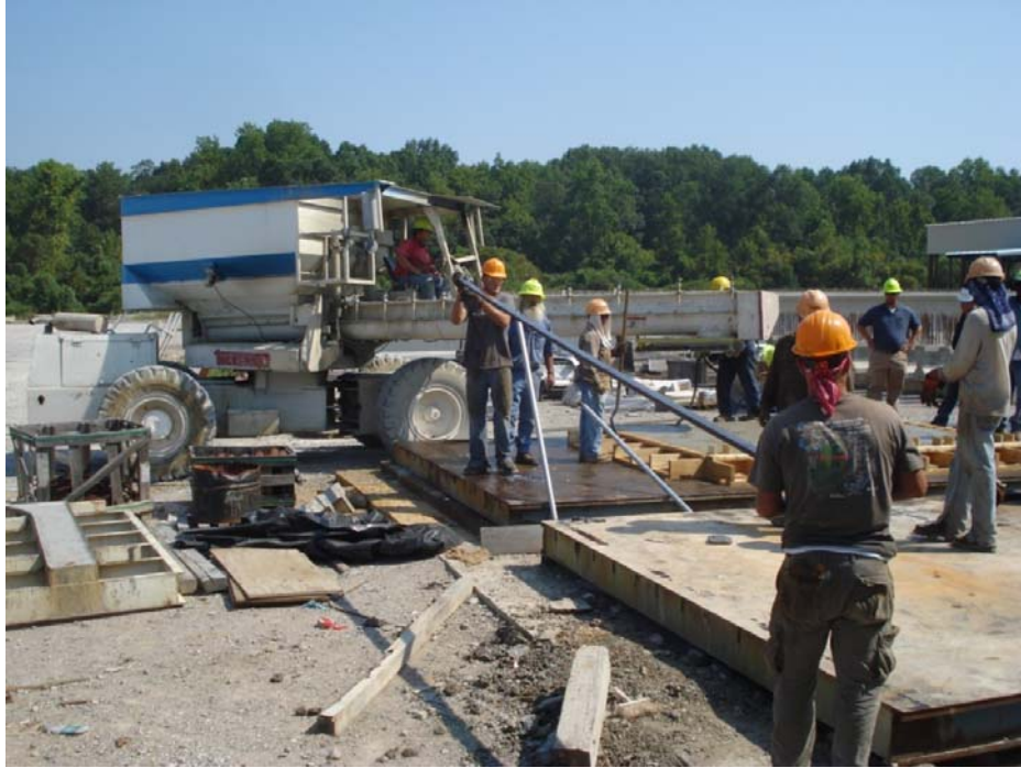
Figure 4-14: Placement of Concrete for Typical Deck Panel
