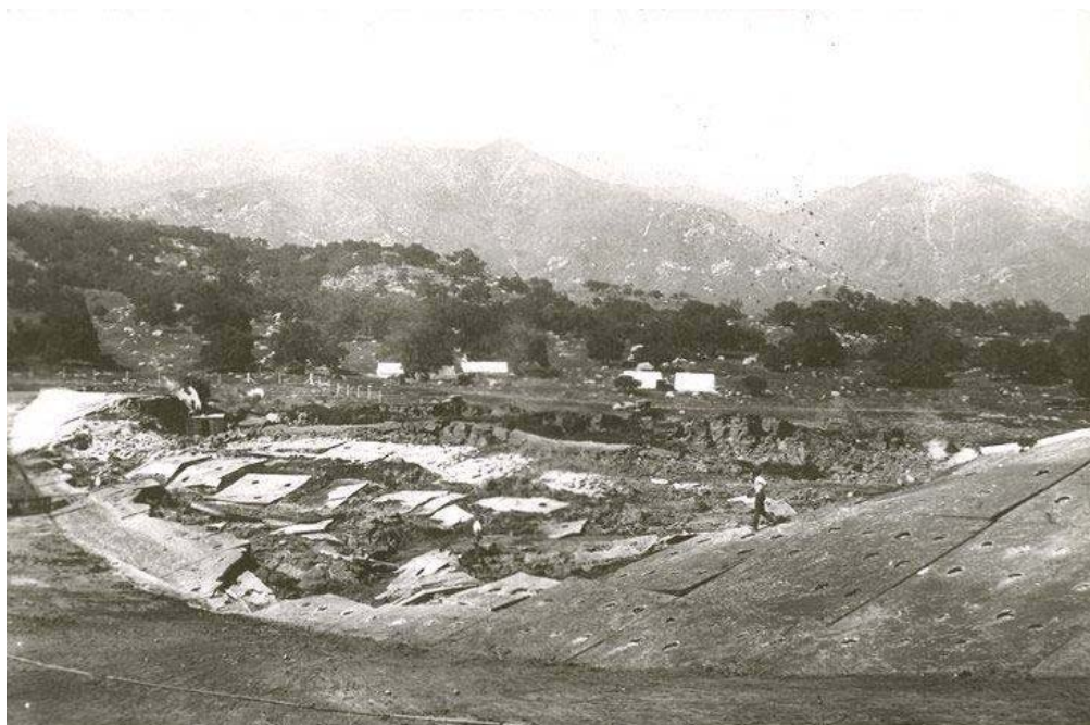
Figure 2.10: Flow failure at Sheffield Dam after 1925 Santa Barbara earthquake
