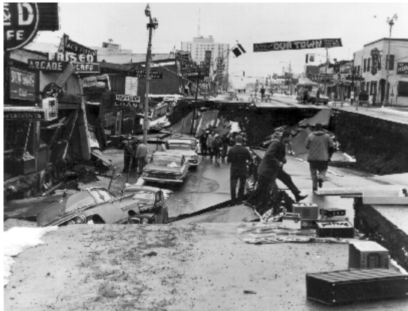
Figure 2.4: Ground deformation due to lateral spreading after the 1964 “Good Friday” earthquake ( http://neic.usgs.gov/neis/eq_depot/usa/1964_03_28.html ).
