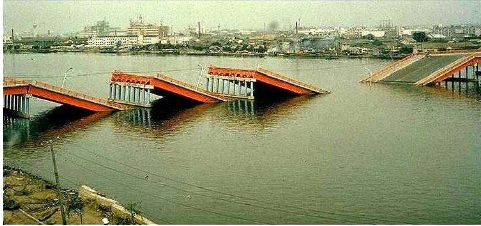
Figure 2.2: Collapse of the Showa Bridge due to liquefaction-induced lateral spreading after the 1964 Niigata earthquake ( http://www.ce.washington.edu/~liquefaction/ ).
