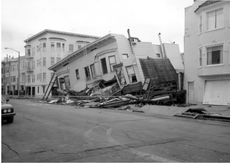
Figure 2.6: Structures damaged in the Marina District of San Francisco. The first story of this three-story building was damaged because of liquefaction; the second story collapsed. What is seen is the third story. Loma Prieta earthquake 1989 ( http://libraryphoto.er.usgs.gov/earth1.htm ).
