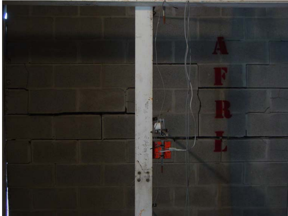
Fig. 3.52. Interior view of Wall 2 after Detonation 3
