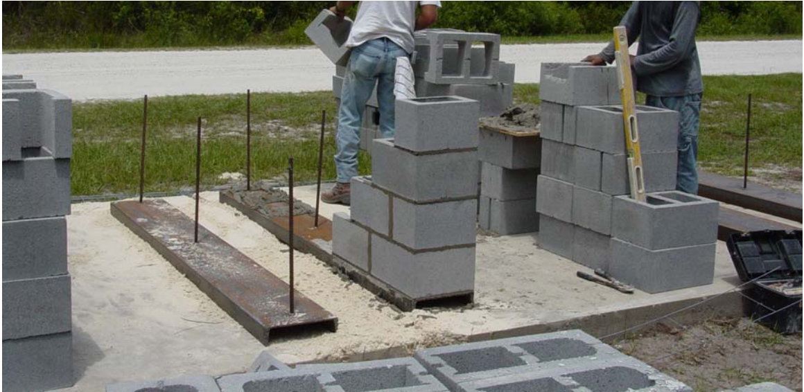
Fig. 3.14. Beginning of Wall 1 construction
