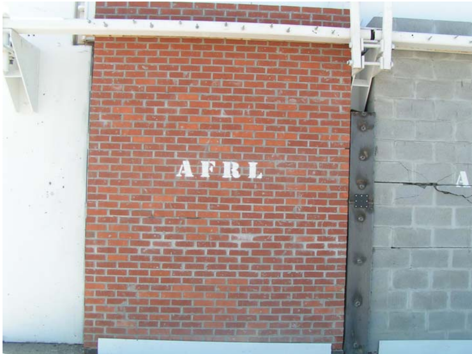
Fig. 3.36. Exterior view of Wall 2 after Detonation 1
