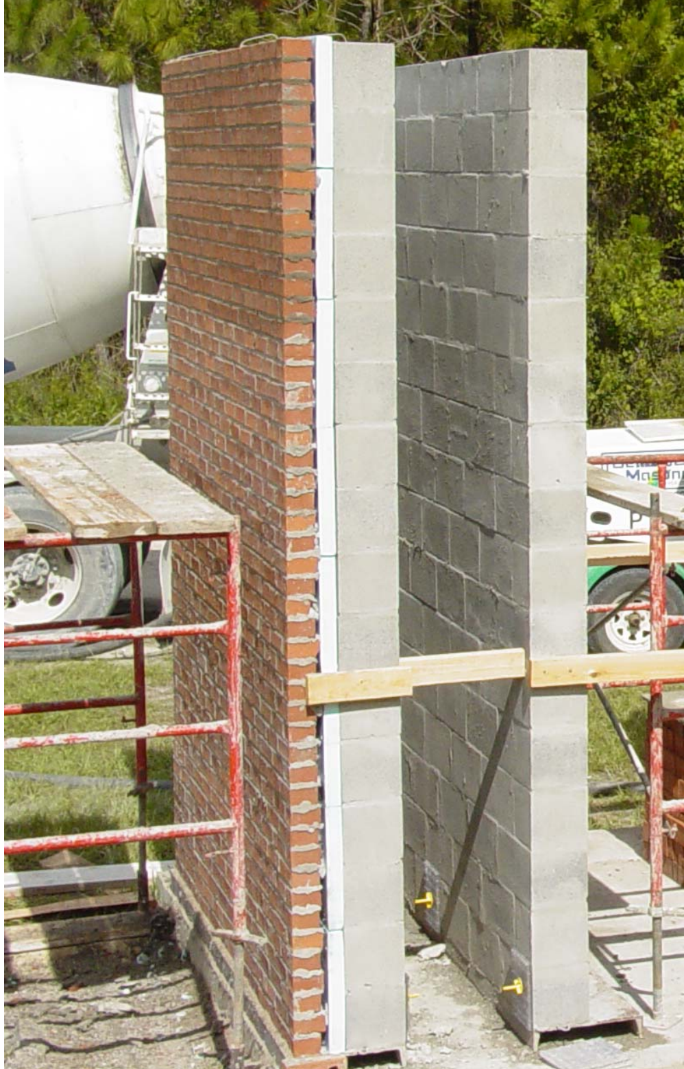
Fig. 3.18. Wall 2 nearing completion
