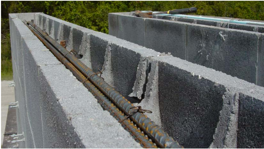
Fig. 3.16. Bond beam before grouting
