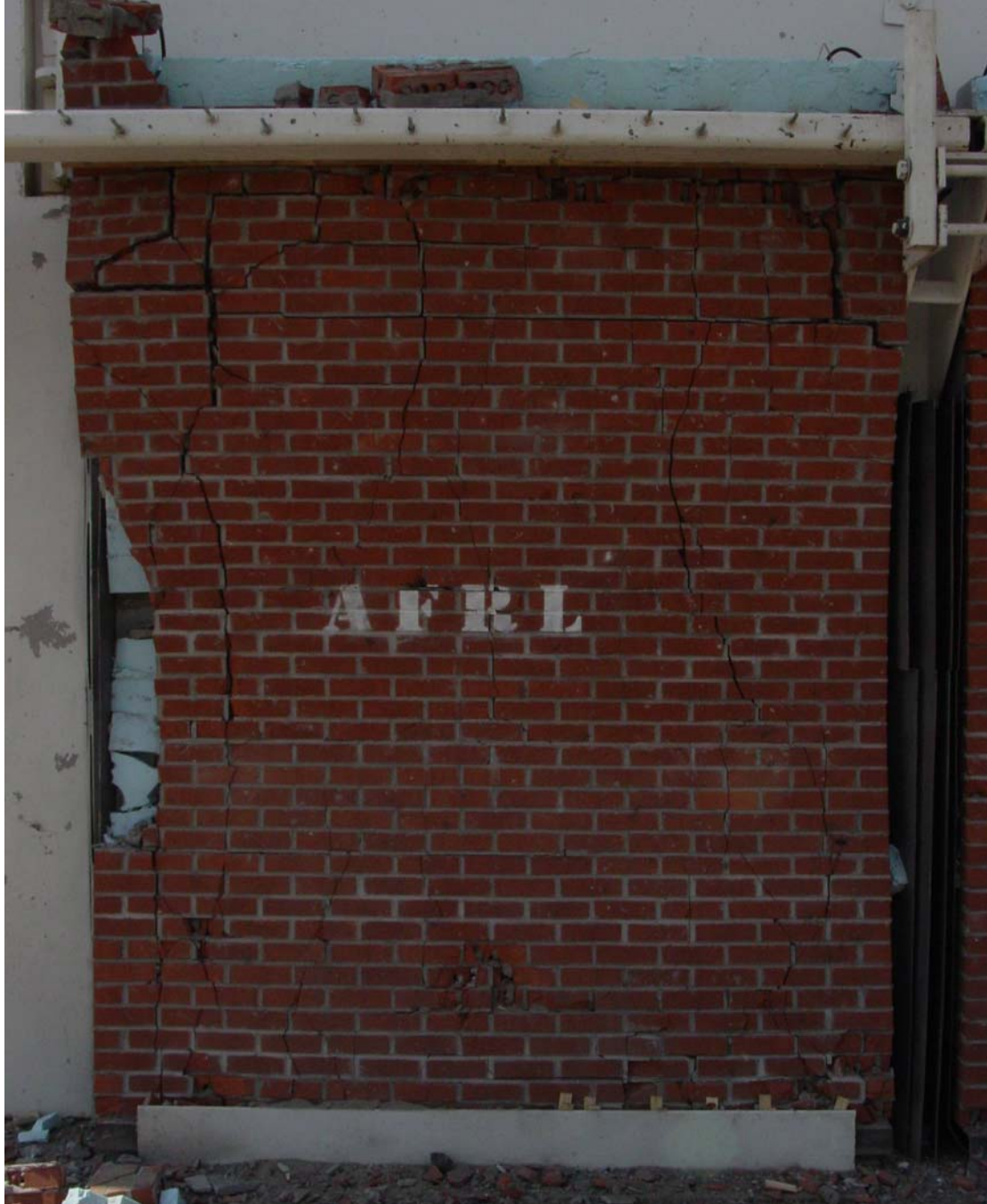
Fig. 3.49. Exterior view of Wall 2 after Detonation 3
