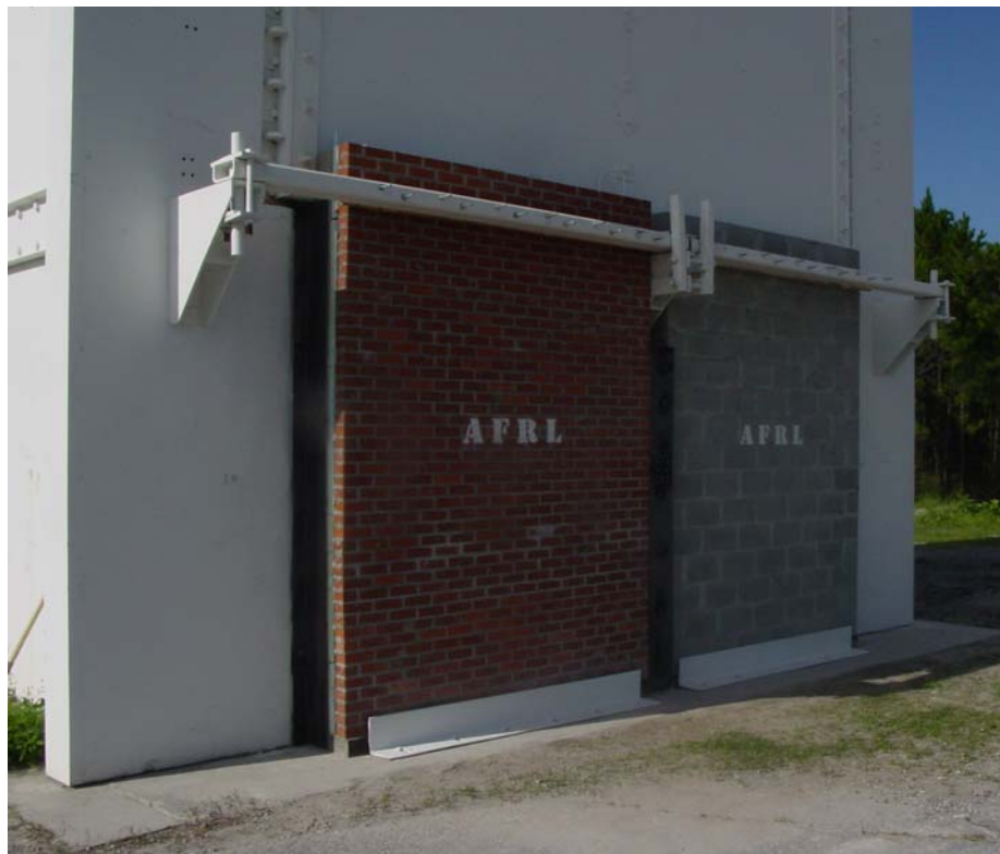
Fig. 3.31. Oblique view of walls prior to detonation
