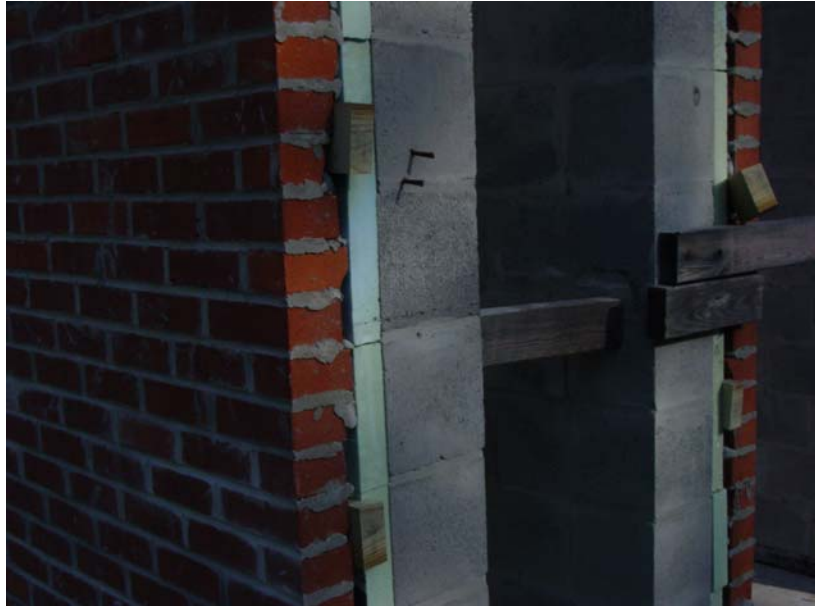
Fig. 3.21. Wooden wedges driven between foam and brick veneer
