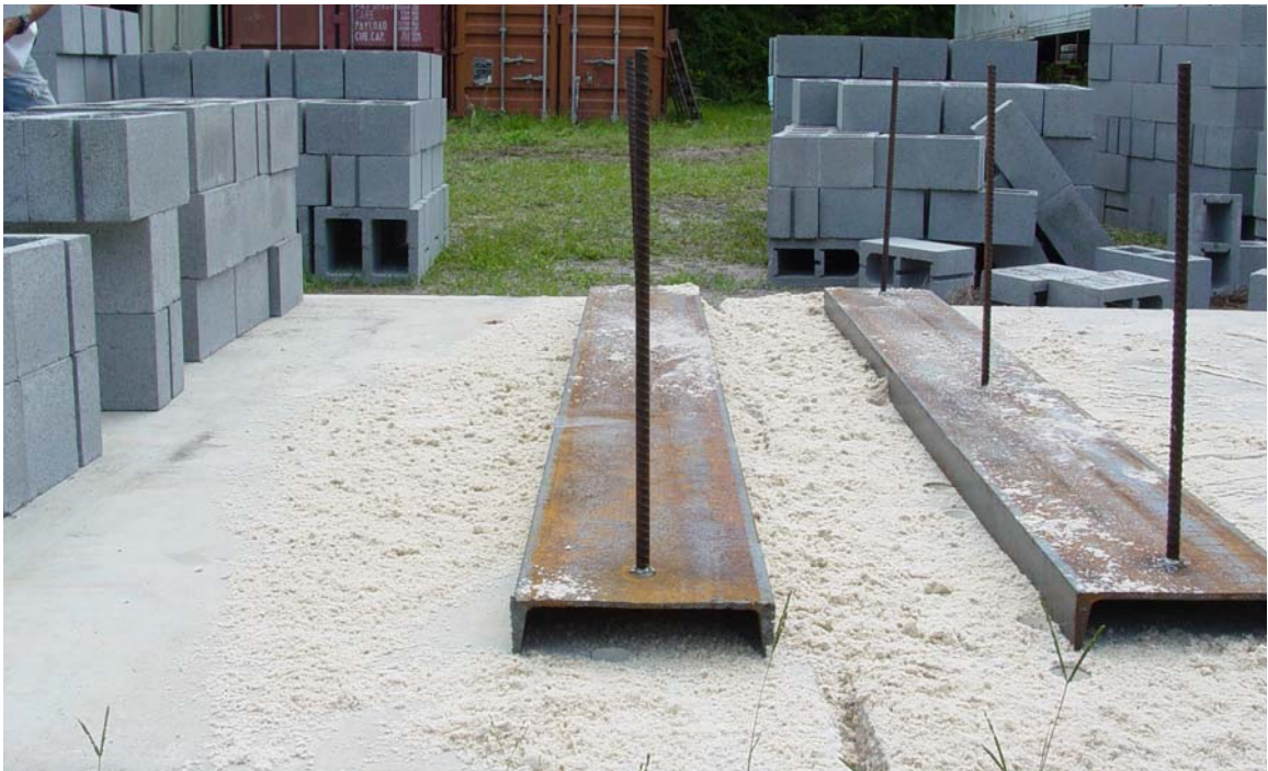
Fig. 3.13. Support channels for walls
