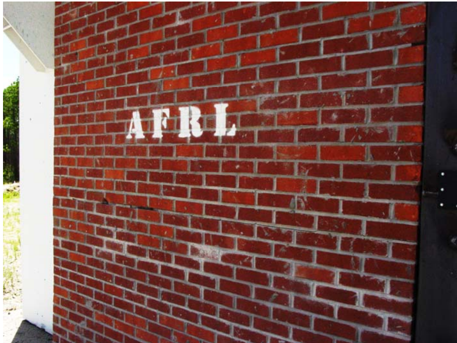
Fig. 3.39. Close-up exterior view of Wall 2 after Detonation 1
