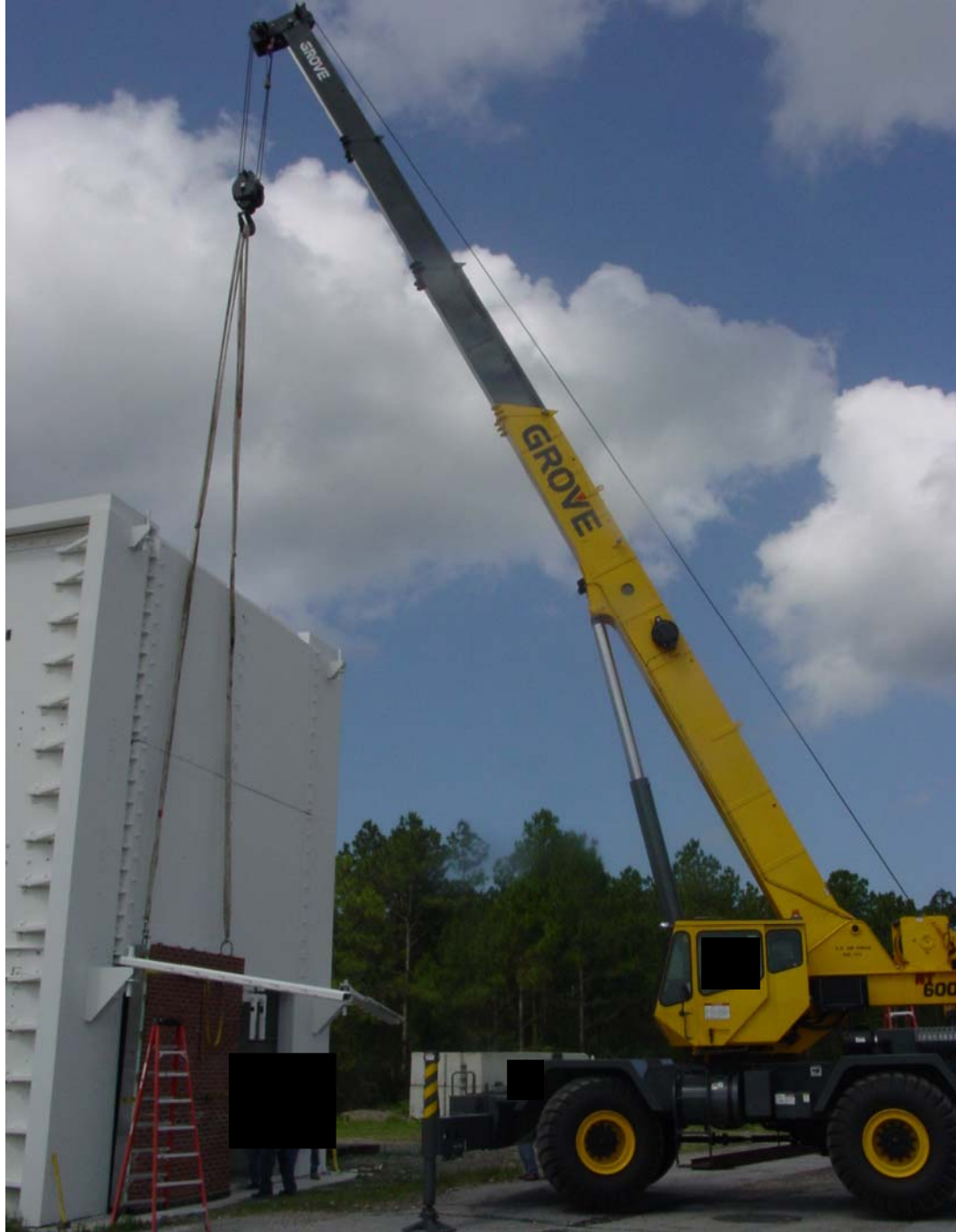
Fig. 3.24. Placing Wall 2 in reaction structure
