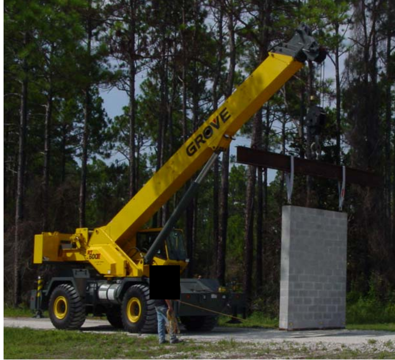
Fig. 3.19. Transporting Wall 1 to test range
