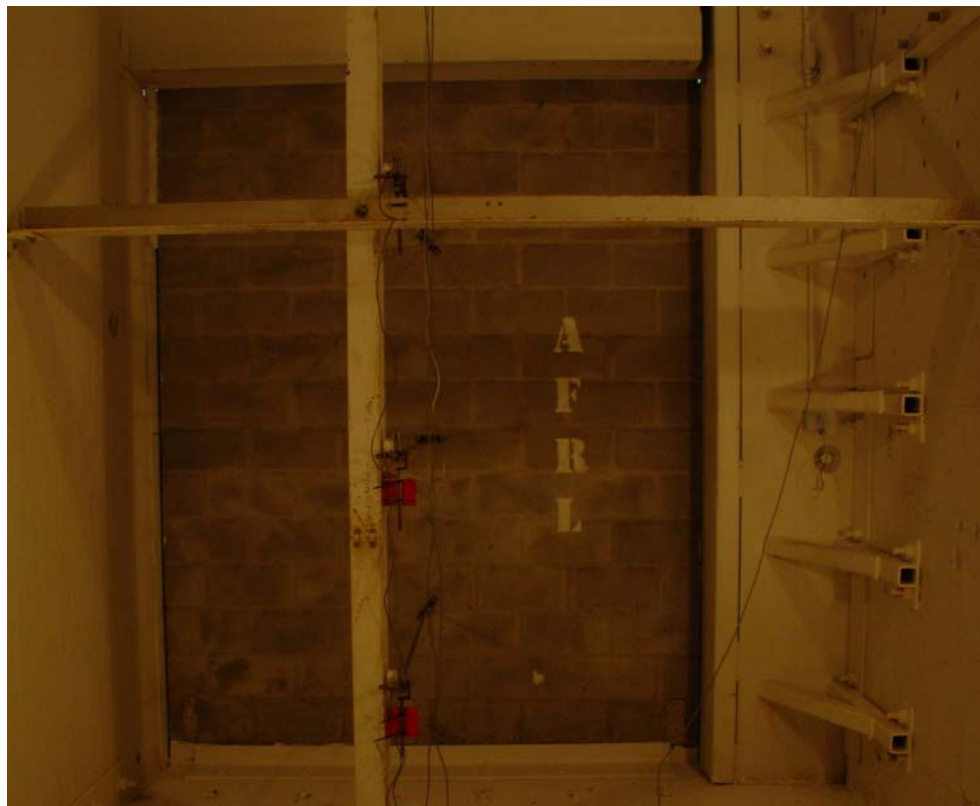
Fig. 3.28. Deflection gauges on Wall 2
