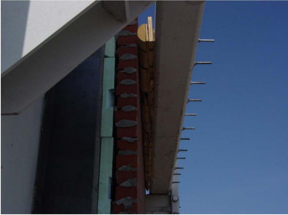
Fig. 3.26. Top exterior support for Wall 2
