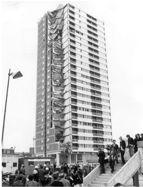
Figure 1-1 Ronan Point Apartments collapse (Copyright Daily Telegraph 1968:
