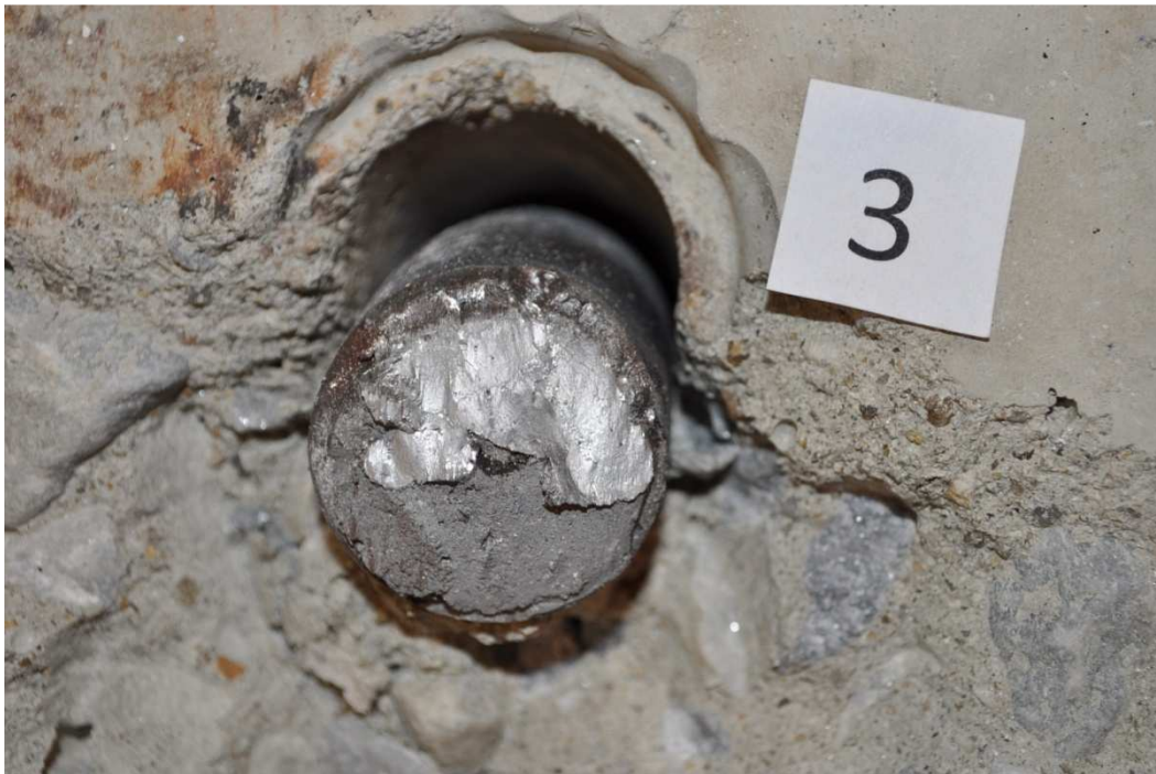
Figure 4-11 Failure Surface for S-1.25-22-B (3)
