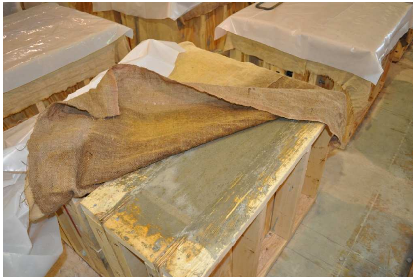
Figure 3-11 Concrete Curing Under Wet Burlap
