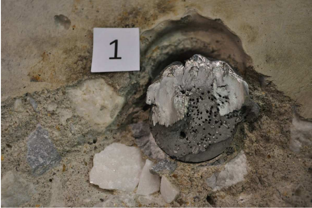
Figure 4-14 Failure Surface for S-1.25-22-C (1)
