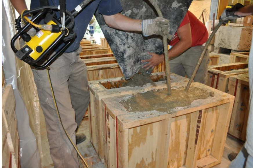
Figure 3-10 Vibrating Concrete to Achieve Proper Consolidation
