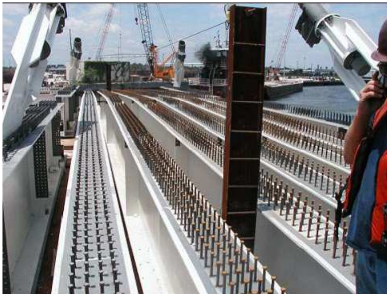
Figure 1-1 Welded Shear Studs on Cooper River Bridge (Champney and Hsu 2009)
