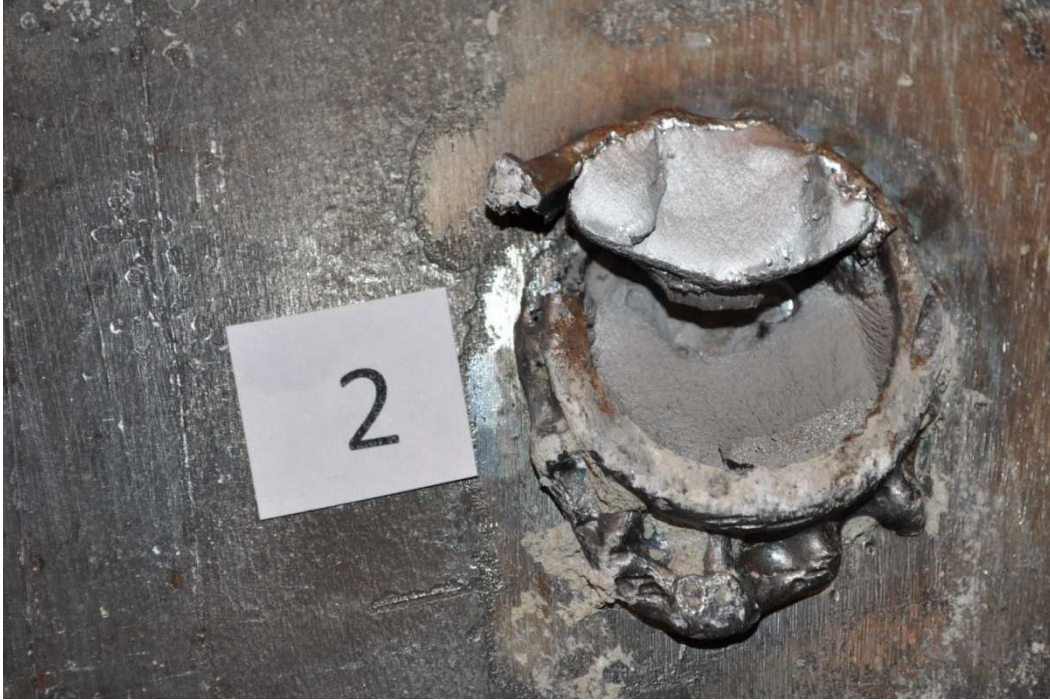
Figure 4-30 Failure Surface for S-1.25-26-D (2)
