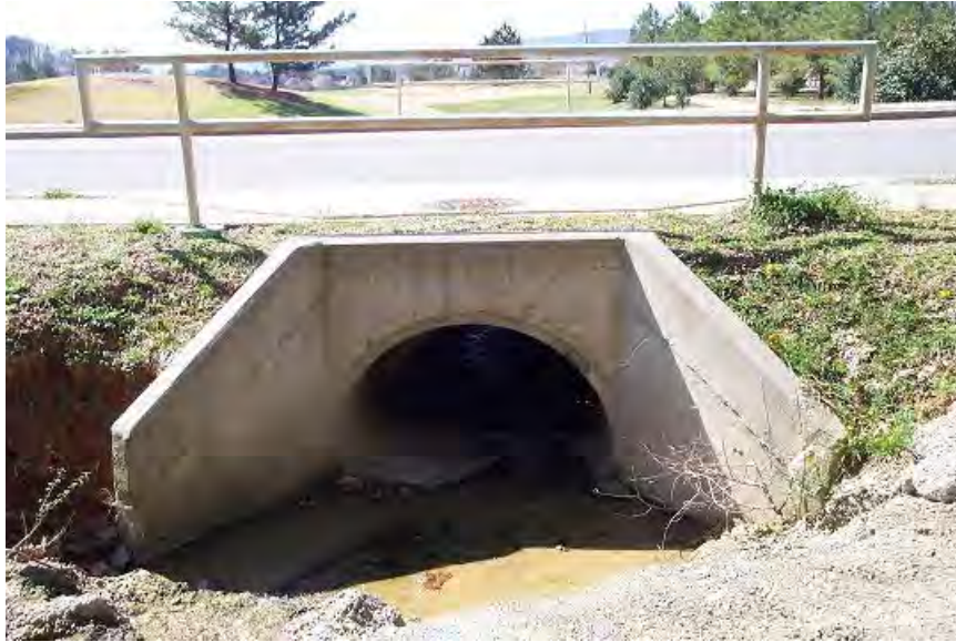
Figure 2.20: Underground roadway drainage culvert (COH 2011)
