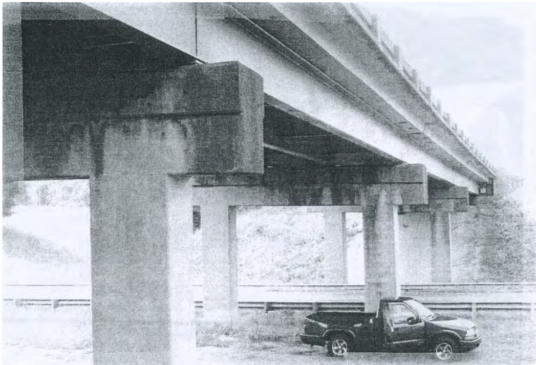
Figure 3.10 I-59 (SBR) Bridge Over SR68 at Collinsville
