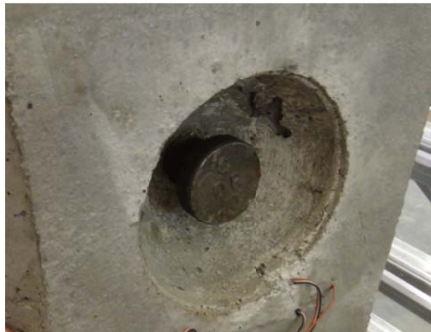
Figure 5-23 Lifter at Concrete Surface
