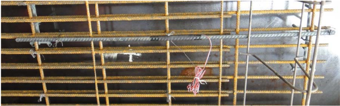
Figure 4-4 Sister Bar Installed in Reinforcement Cage
