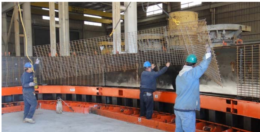
Figure 2-5 Steel Mat Bowing to Fit Arch Radius
