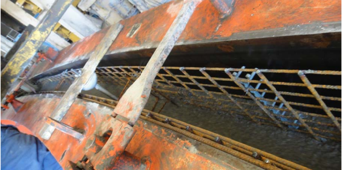
Figure 2-6 Casting of Bridge Unit
