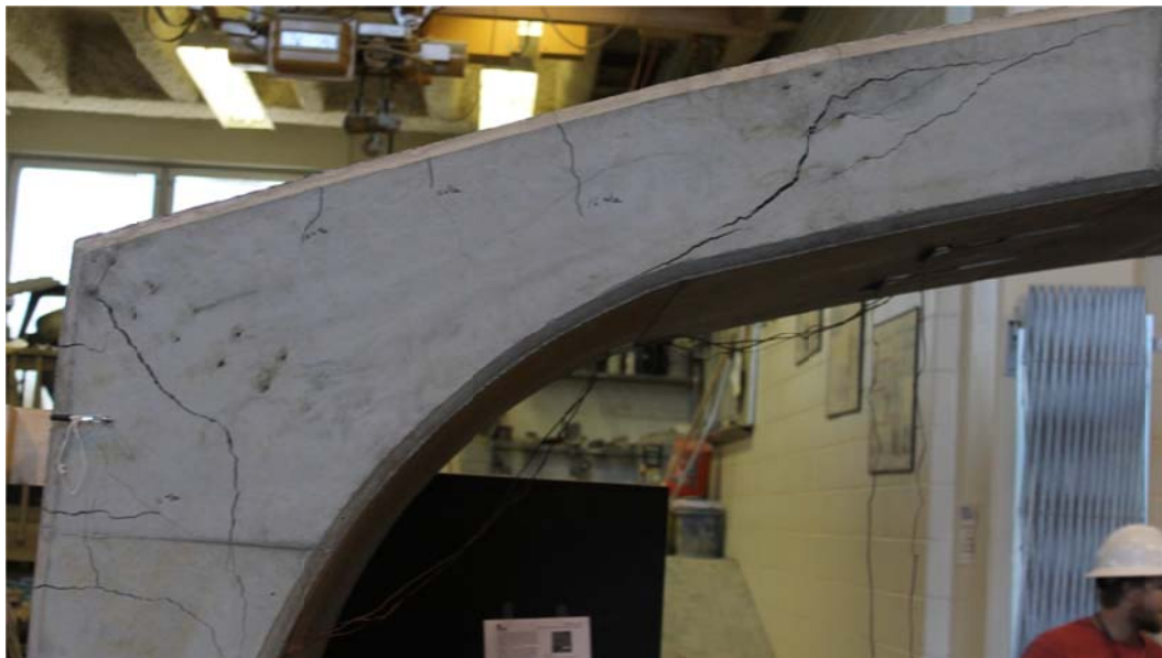
Figure 4-38 Immediately Prior to Failure
