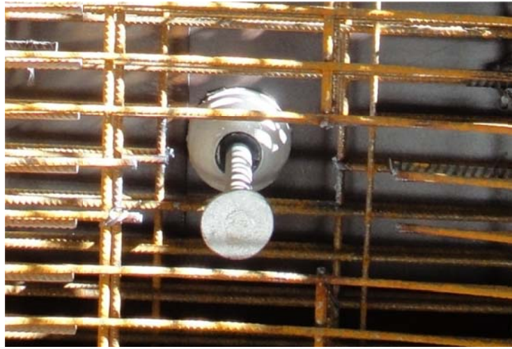
Figure 5-25 Reinforcement Cut at Lifter Location
