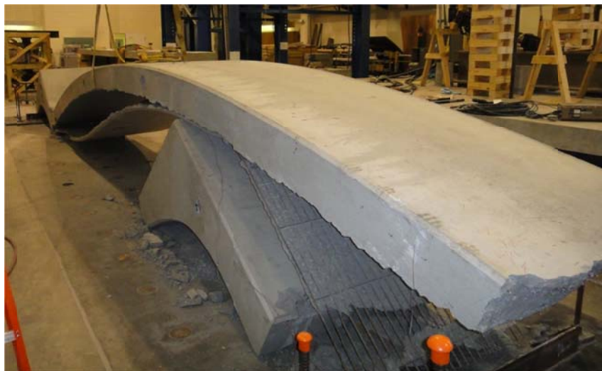
Figure 5-27 Demolished Bridge Unit
