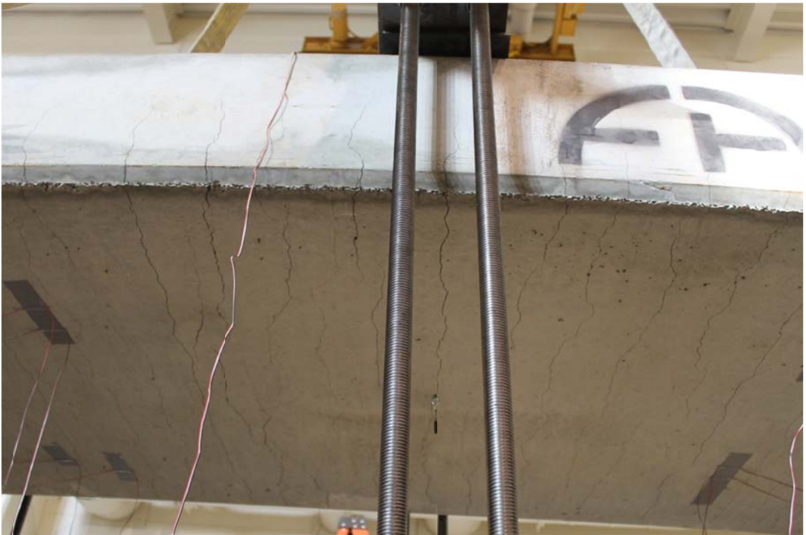
Figure 5-15 Midspan Cracking – After Failure
