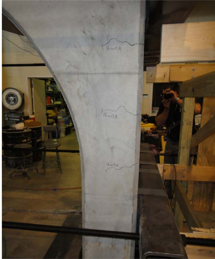
Figure 4-32 Initial Cracks in Leg
