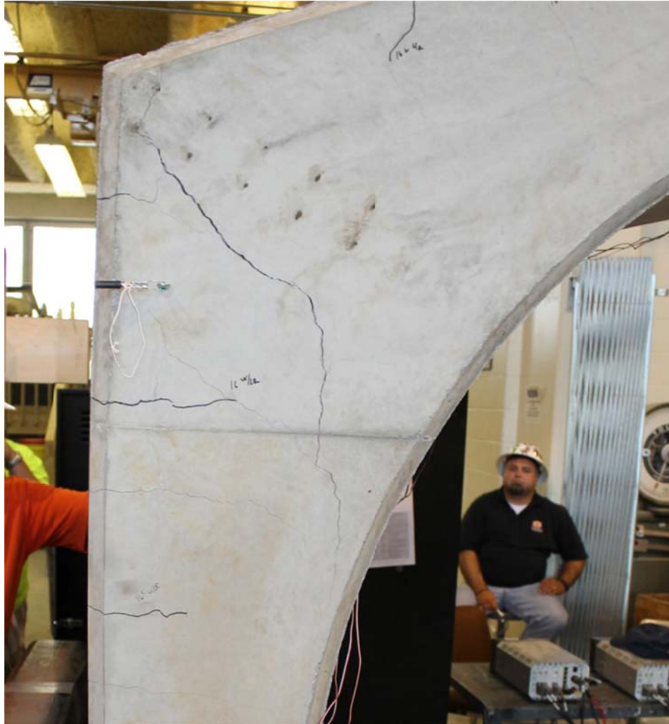
Figure 4-36 Corner Crack at 156 kip Total Load
