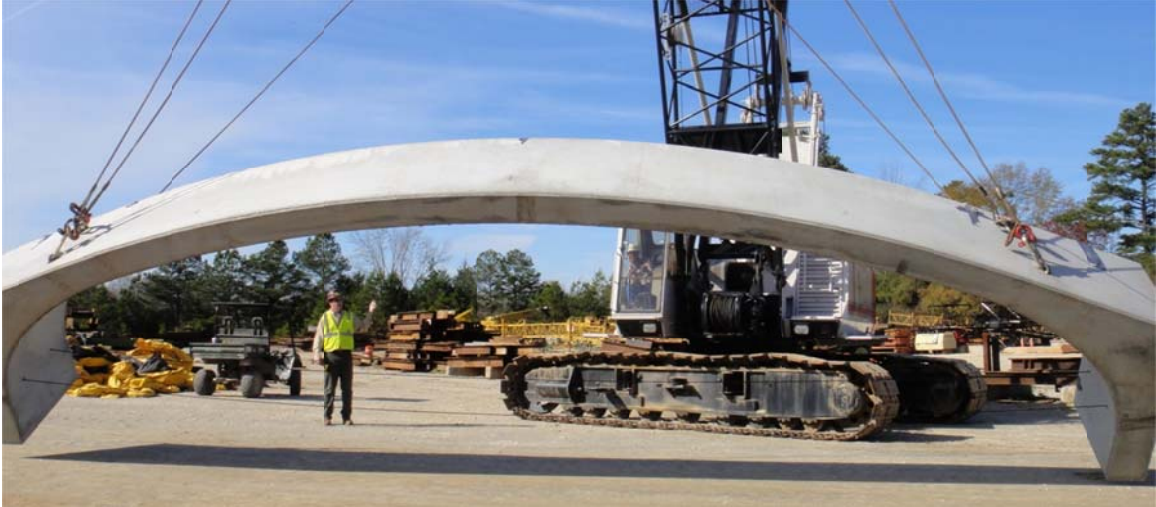
Figure 2-8 Arch Culvert Unit Being Rotated
