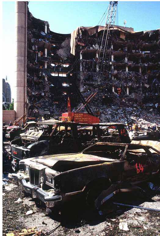
Figure 1-1 Alfred P. Murrah Collapse (accessed from: DefenseImagery.mil )
