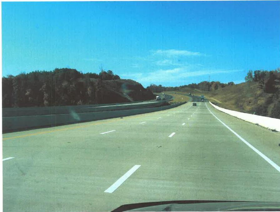
Figure 39: Station 155+00, Corridor X project (Photo courtesy of HMB).
