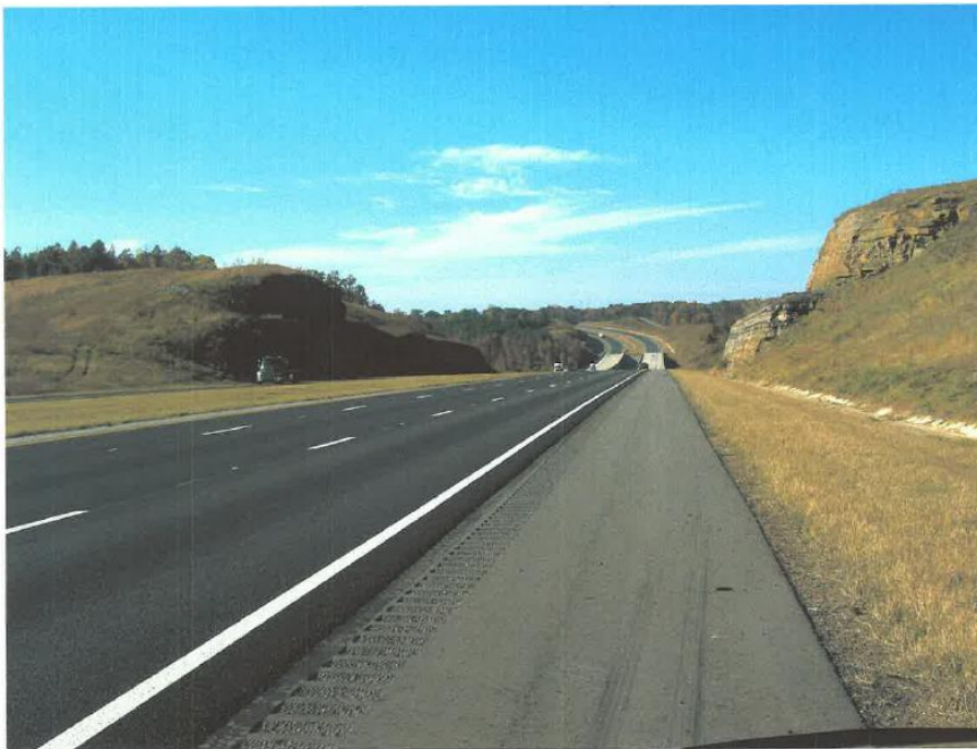
Figure 40: Station 185+00, Corridor X project (Photo courtesy of HMB).
