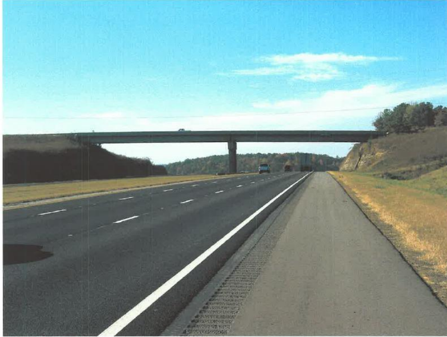
Figure 41: Station 250+00, Corridor X project (Photo courtesy of HMB).
