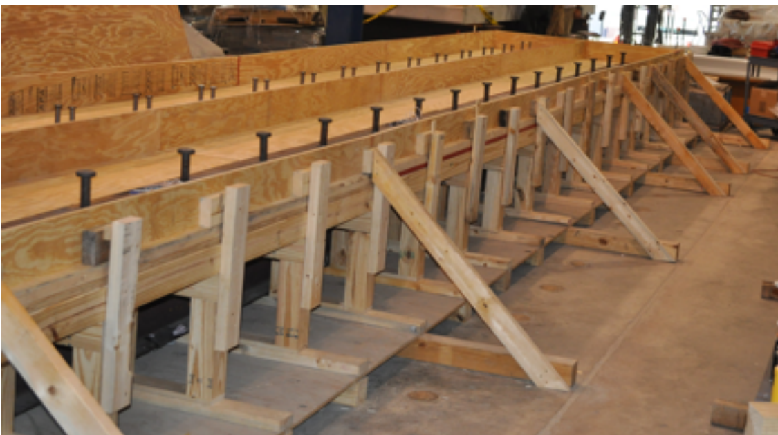
Figure 3.4-3: Fully assembled concrete formwork
