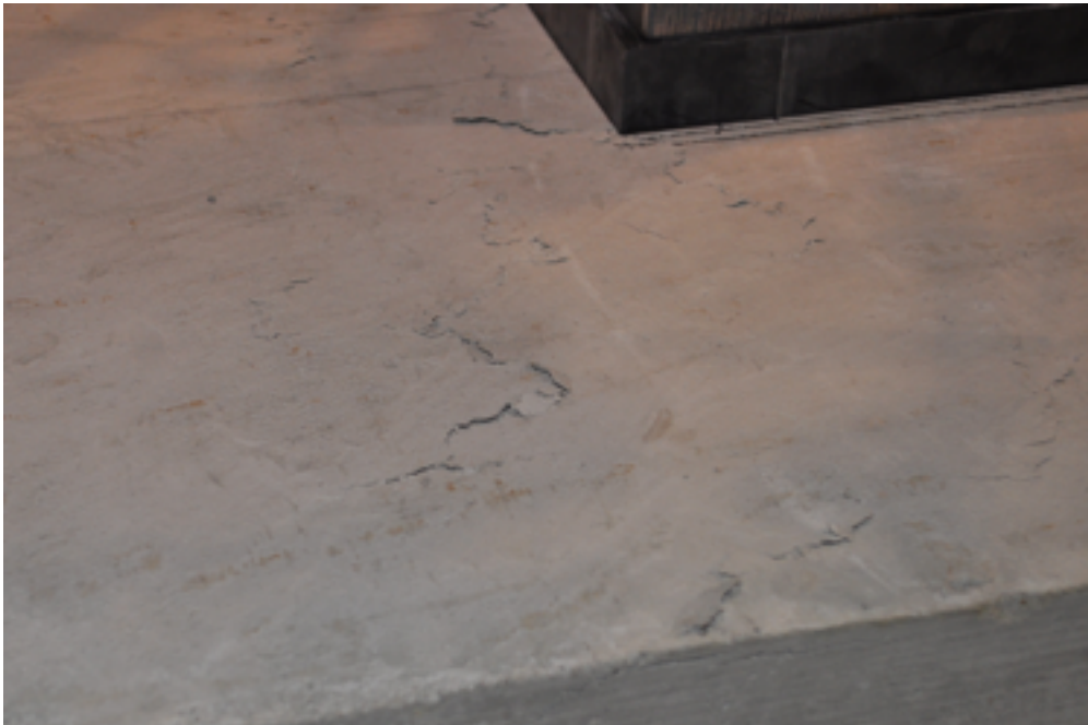
Figure 4.4-11: Crushing of concrete deck for Specimen 4 after failure
