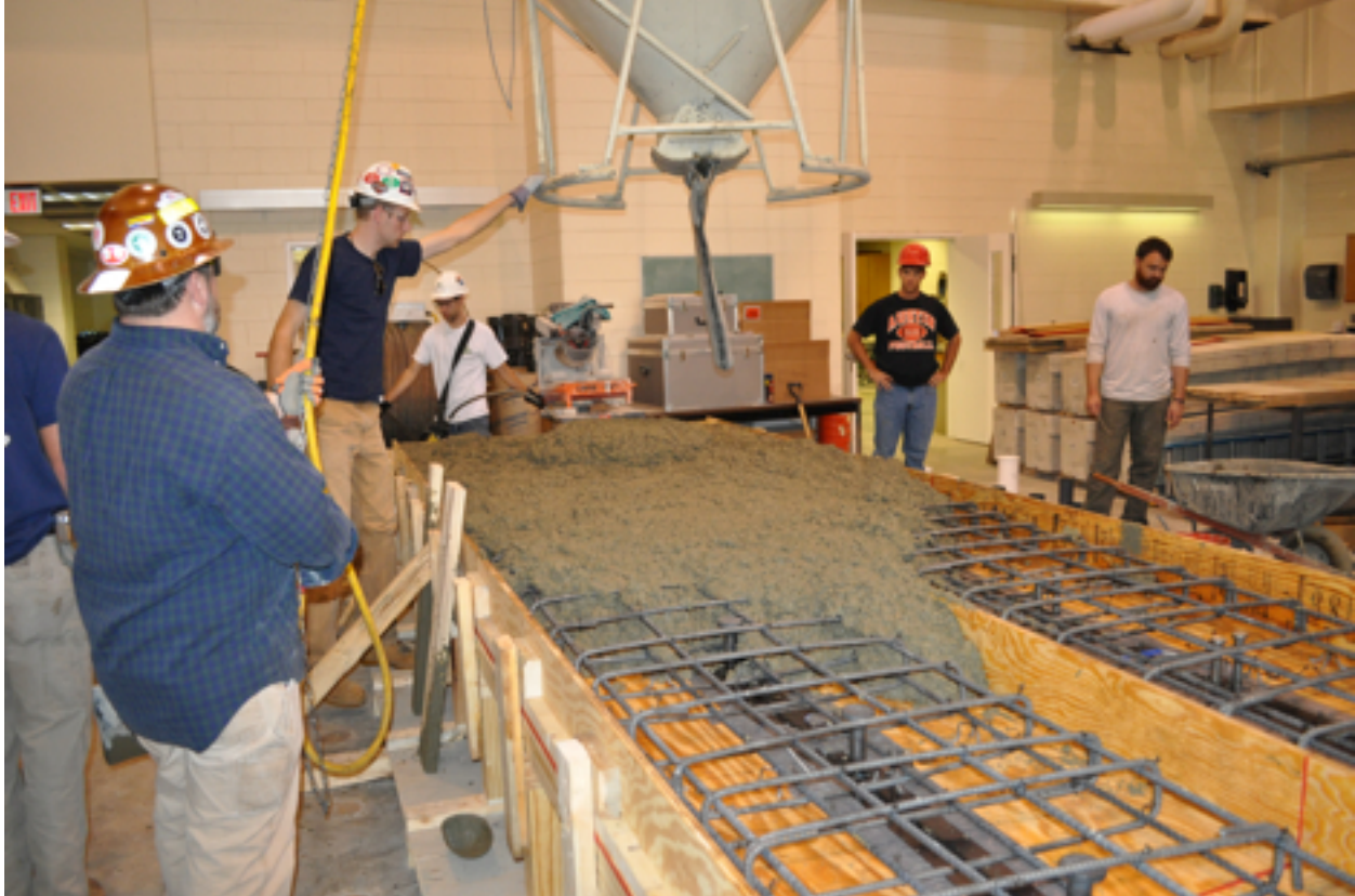
Figure 3.4-4: Casting of concrete deck from overhead hopper
