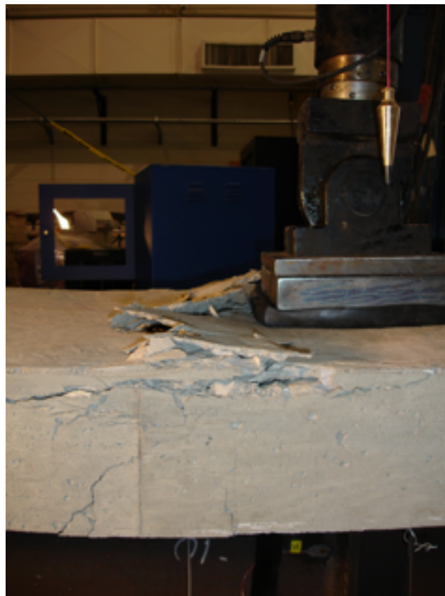
Figure 4.4-6: Crushing at top of deck and cracking at bottom of the deck for Specimen 1
