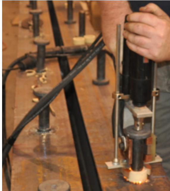
Figure 3.4-1: A stud welding gun with modified cradle welds a large diameter shear stud to the top flange of a test specimen
