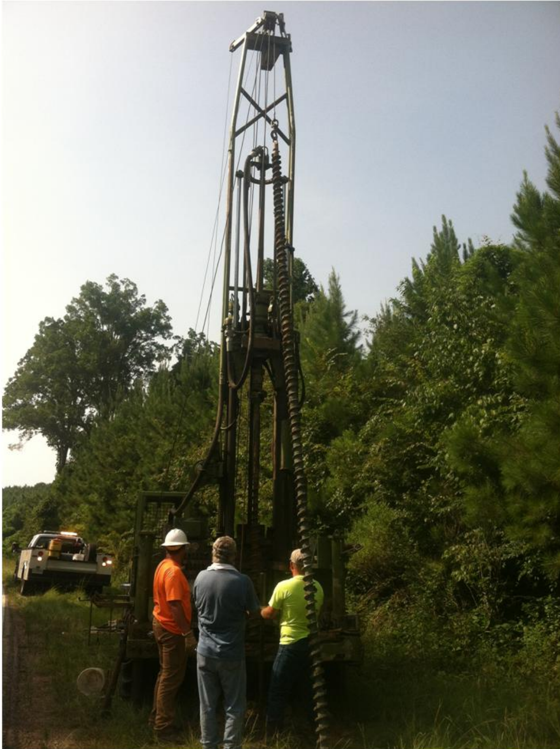
FIG. 3-12. Photograph of ALDOT Drilling for Yazoo Clay.
