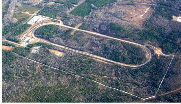
Figure 5.10: NCAT's 1.7 mile long test track where the test vehicle was driven
