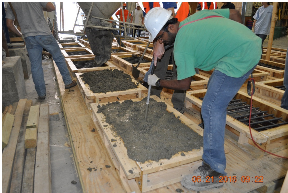
Figure 4.17: Vibrating the Concrete
