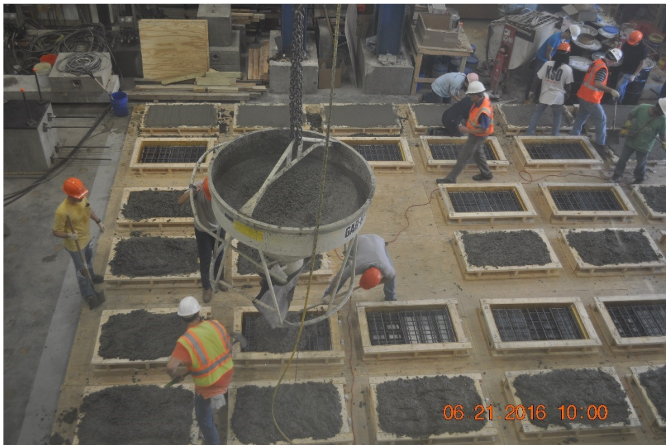
Figure 4.19: Overview of Concrete Placement
