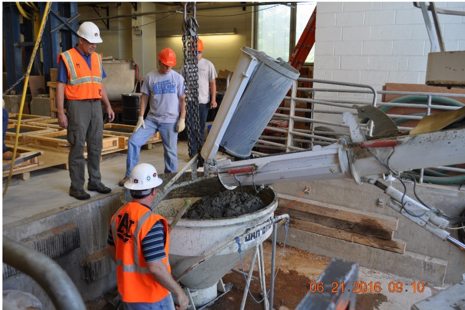
Figure 4.15: Delivery of Ready-Mixed Deck Concrete
