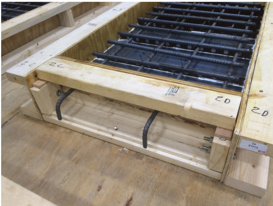
Figure 4.14: Close-up View of Completed Forms
