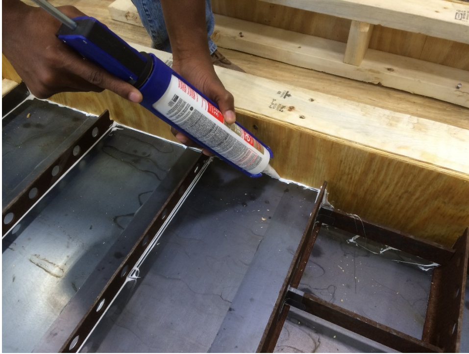
Figure 4.13: Caulking the Forms
