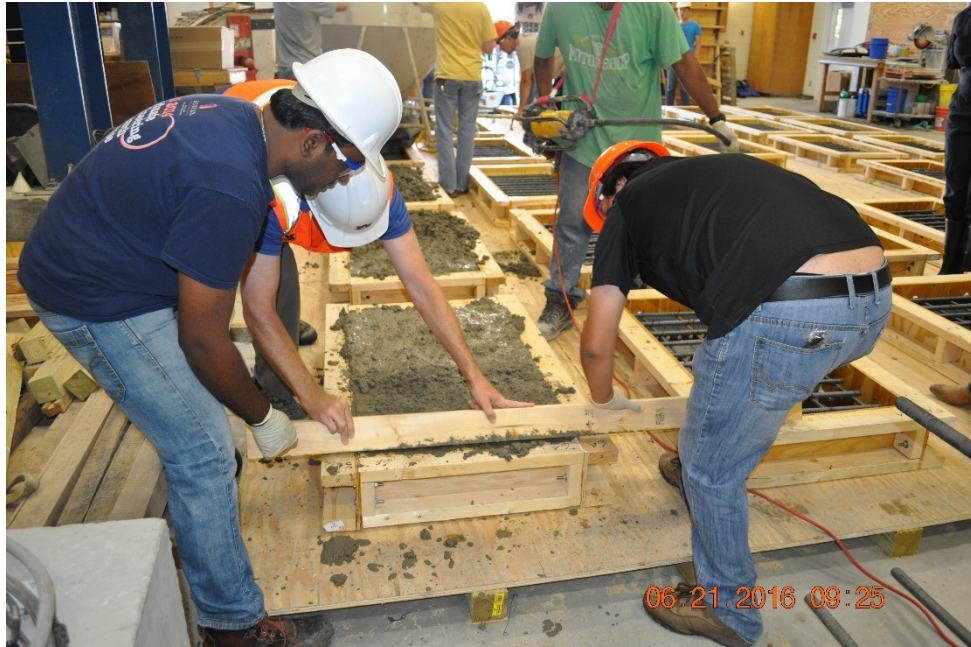
Figure 4.18: Screeding off the Excess Concrete
