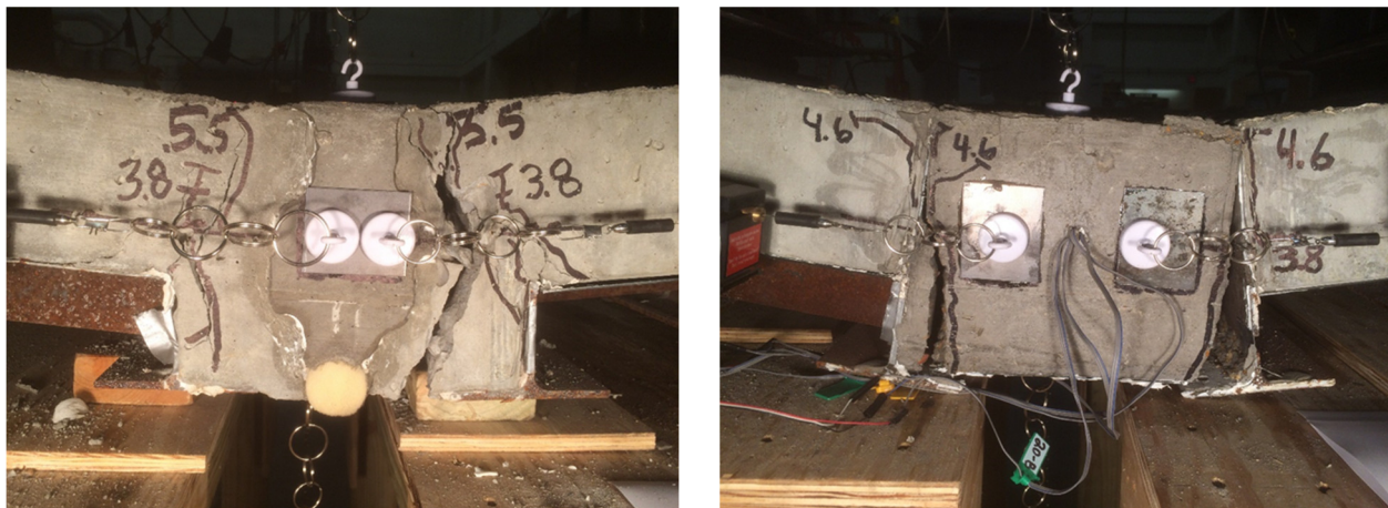
Figure 5.70: Cracking Behavior in the Unreinforced and Reinforced Joints
