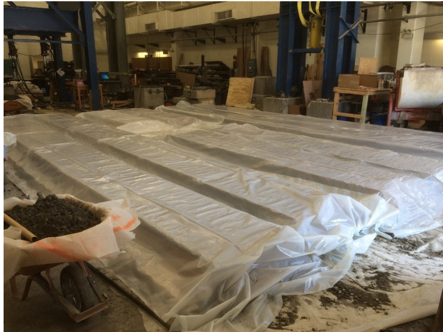
Figure 4.21: Wet Burlap and Plastic Sheeting over Panels
