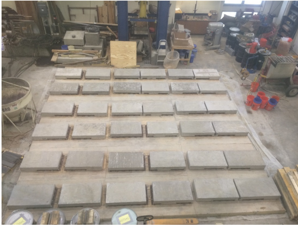
Figure 4.23: Overview of Panels before Grout Pour
