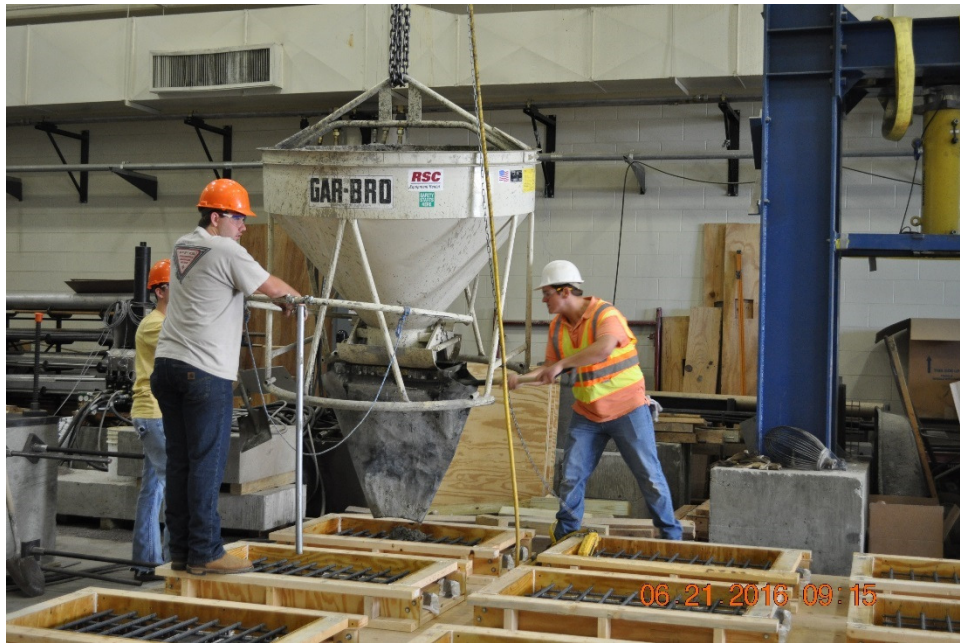
Figure 4.16: Placement of Concrete
