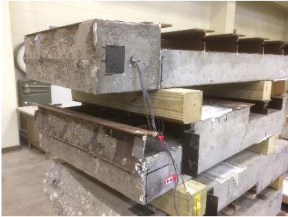
Figure 5.50: Separated Deck Panels (R-NEG-F)
