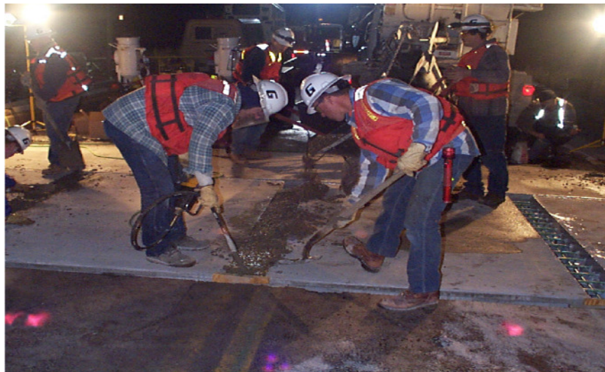
Figure 2.27: Placement of Rapid-Setting Concrete in the Joints of the Longstreet Bridge (Umphrey 2006)
