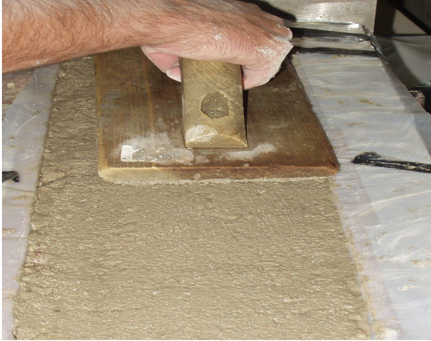
Figure A-18: Finishing of the fresh concrete
