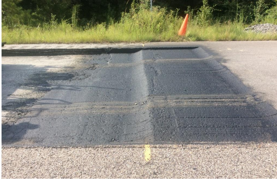
FIGURE 3.10 Tack Application in Transition Zone.
