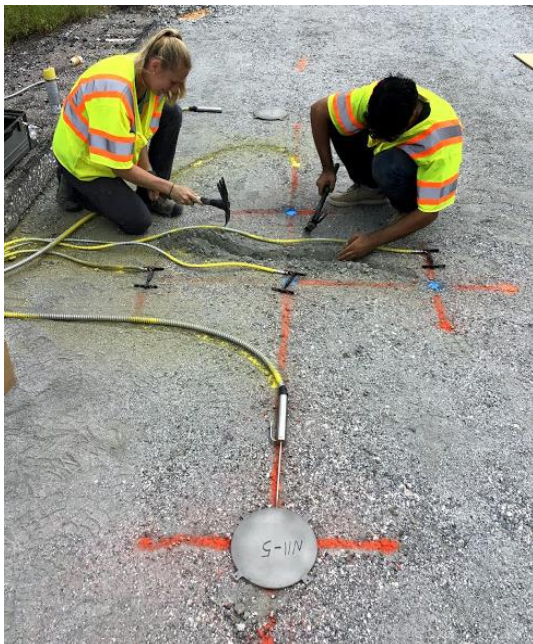
c) Digging Shallow Trenches
