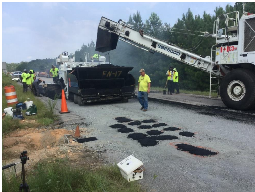
FIGURE 3.11 Paver in Use During S9 Construction.
