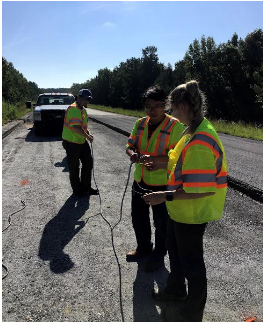
a) Threading Wires in Conduit
