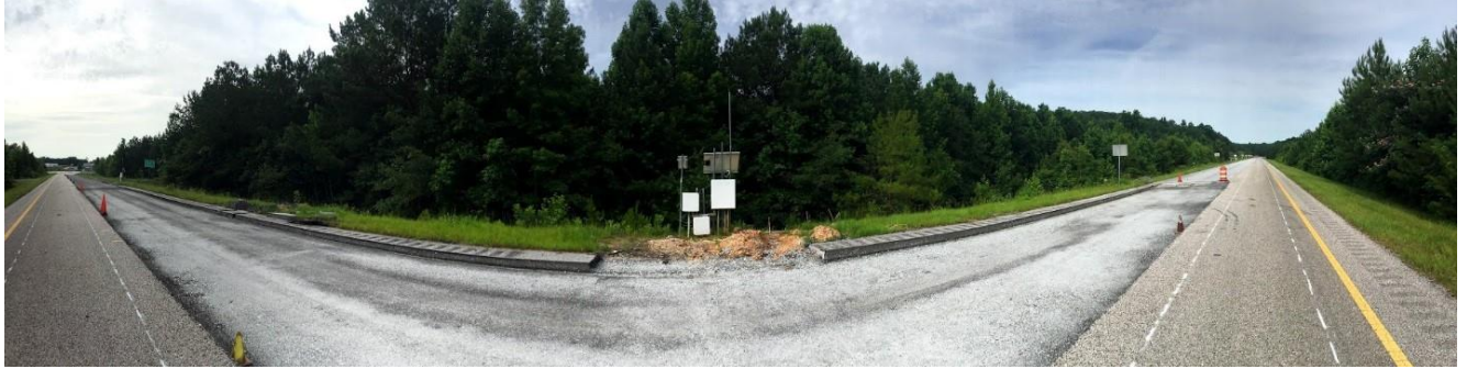
FIGURE 3.8 Section S9 Before Gauge Installation – Granular Base.
