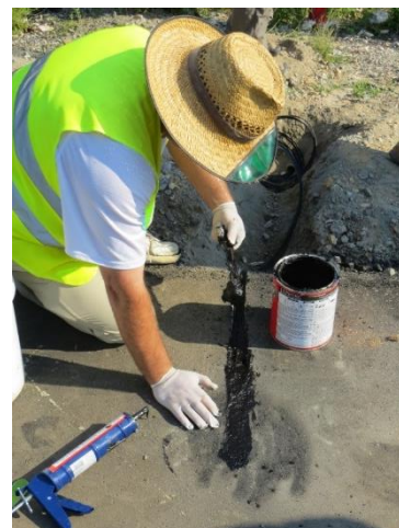
e) Roofing Cement Process
