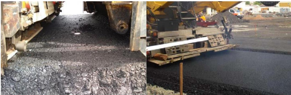
FIGURE 2.3 Thick Lift Pavement During Construction (Tielmann and Böhm, 2016).
