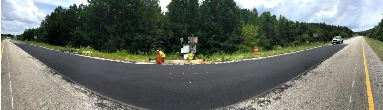
FIGURE 3.13 Section S9 after Paving.
