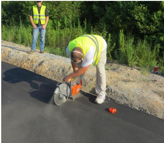
a) Saw Cutting Probe Trench
