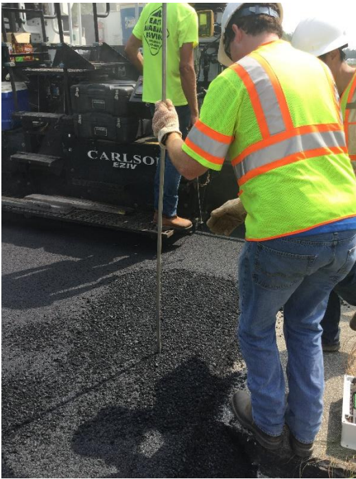
a) Creating Pilot Hole
