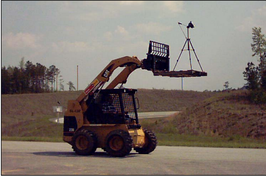
Figure 3.10. Camera Apparatus for Crack Record.
