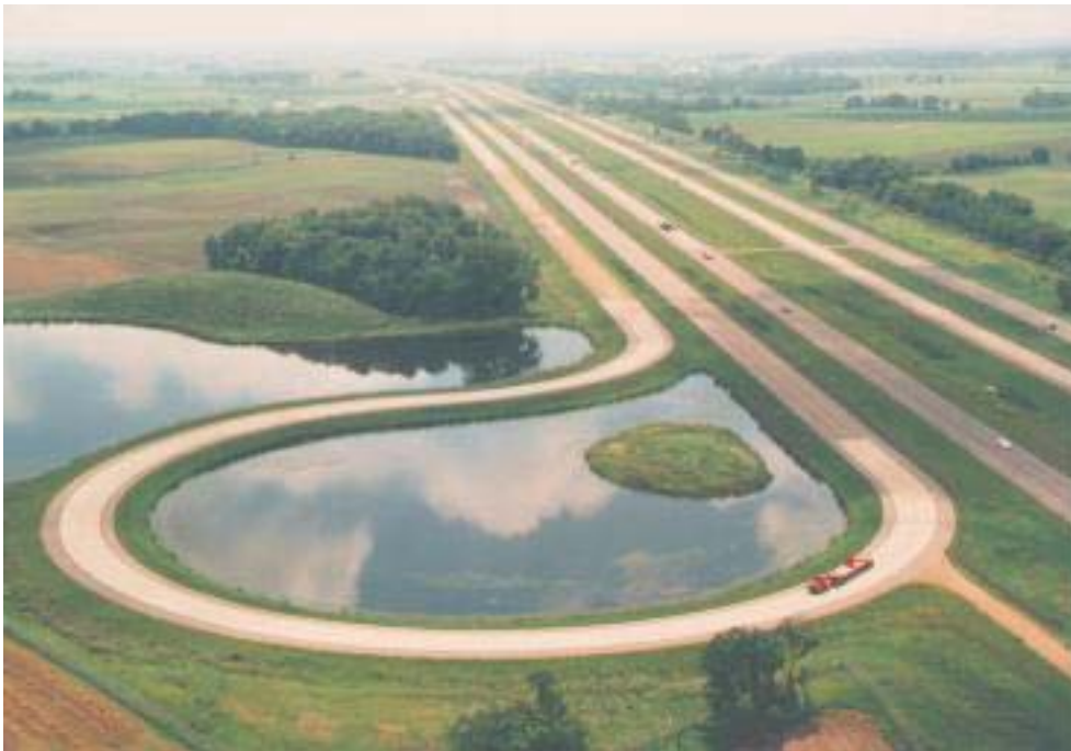
Figure 2.7. Mn/ROAD Facility (“About Minnesota,” 2005).
