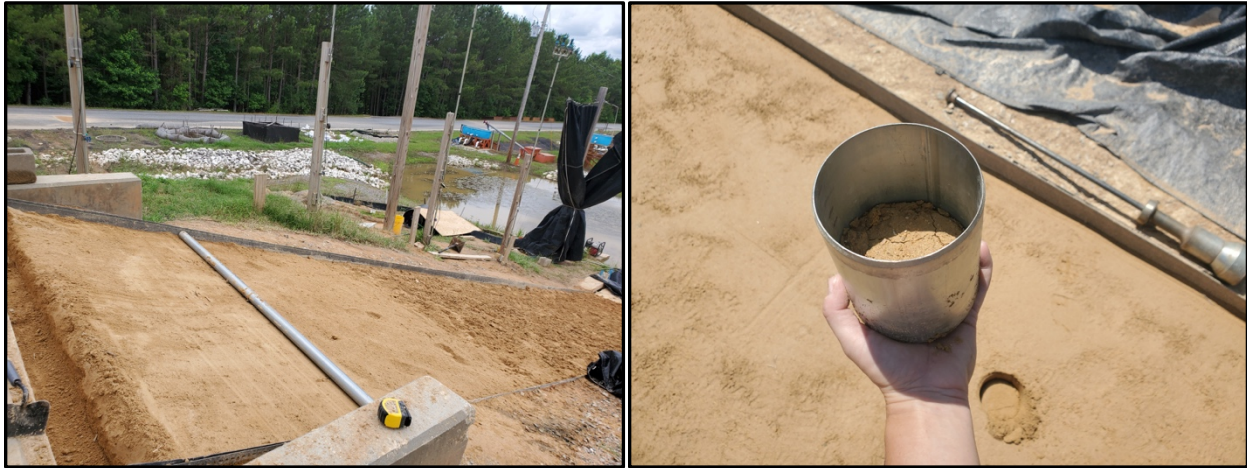
(a) Grading the slope
