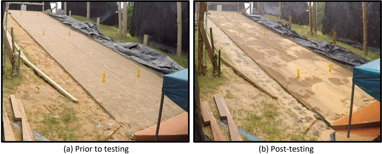
FIGURE 2.15: PAM Test Photos
