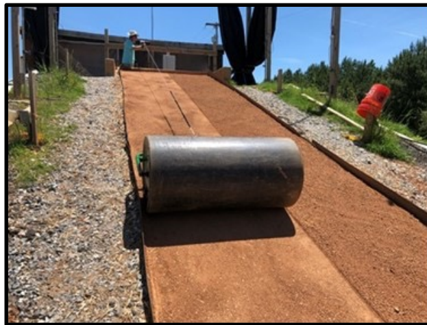
(c) Roller compaction (Faulkner 2020)
