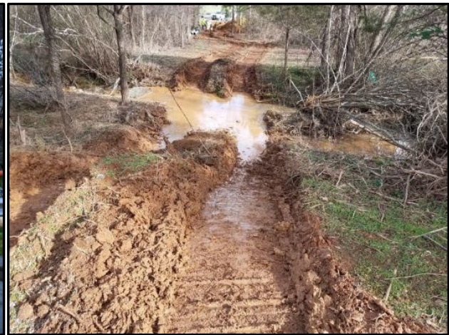
(c) A sediment-laden stream resulting in a $10,000 fine
