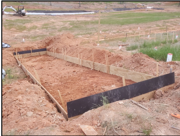
(a) Plot excavated and ready for fill
