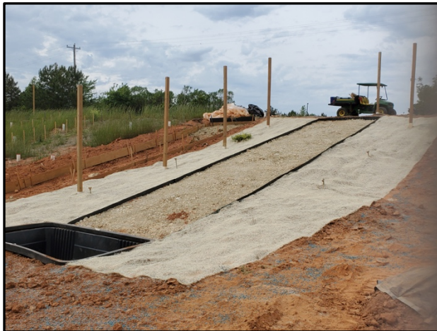
(e) Finished first plot, lower view
