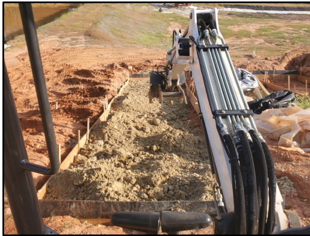
(c) Distributing soil after a lift
