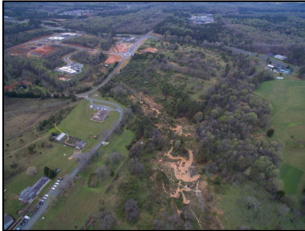
(a) Stormwater runoff from Chatham Park, North Carolina
