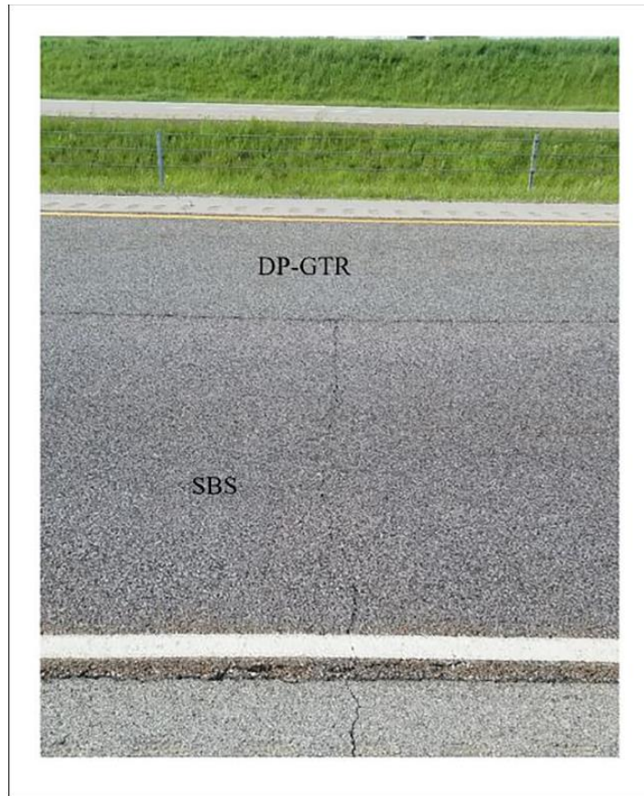
Figure 2.12: Picture of Dry Process GTR and SBS Modified Sections (Rath et al., 2021)
