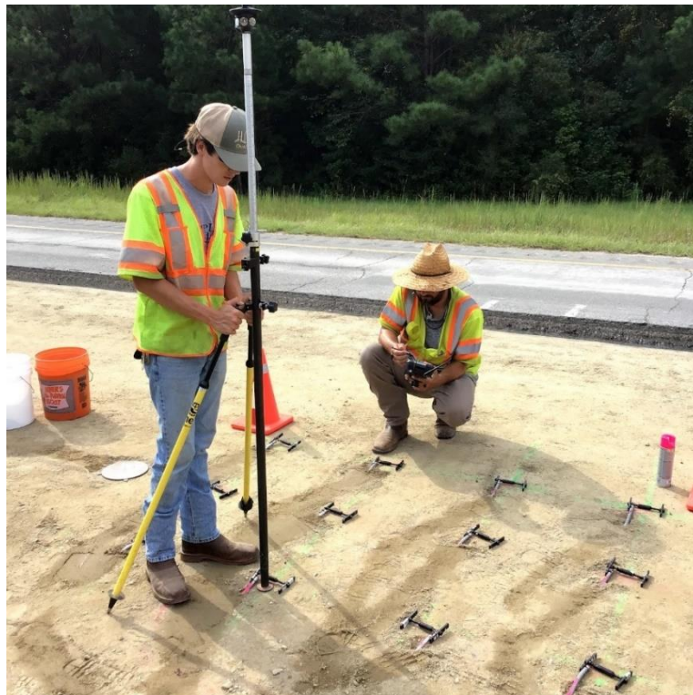
Figure 3.12: Surveying Installed ASGs and Base Layer EPC
