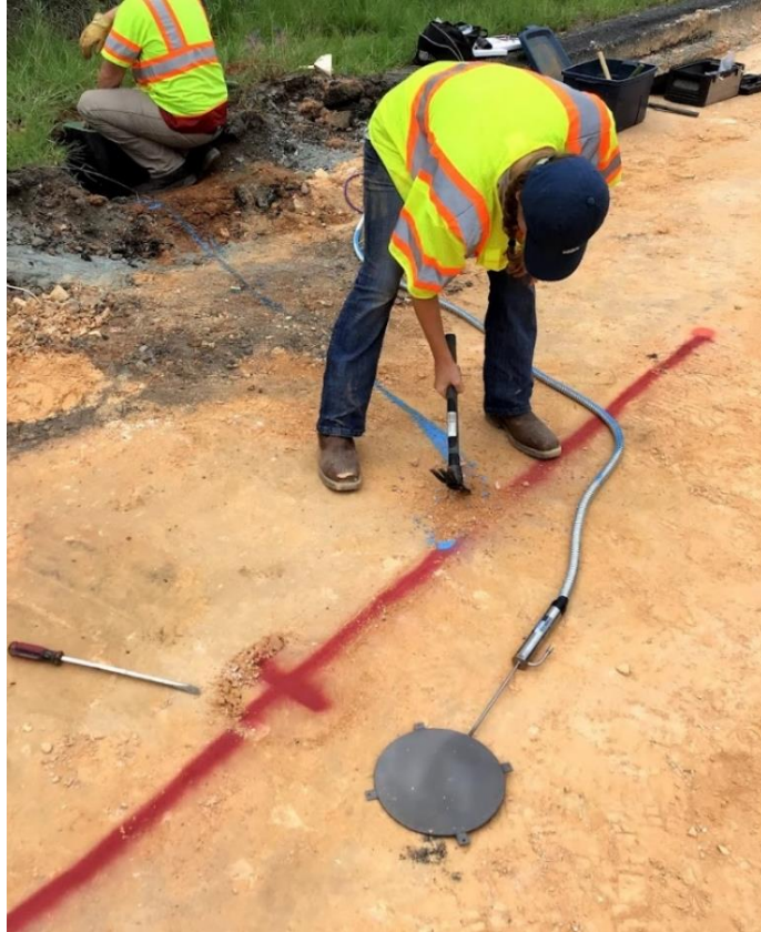
Figure 3.5: Subgrade Trench Digging
