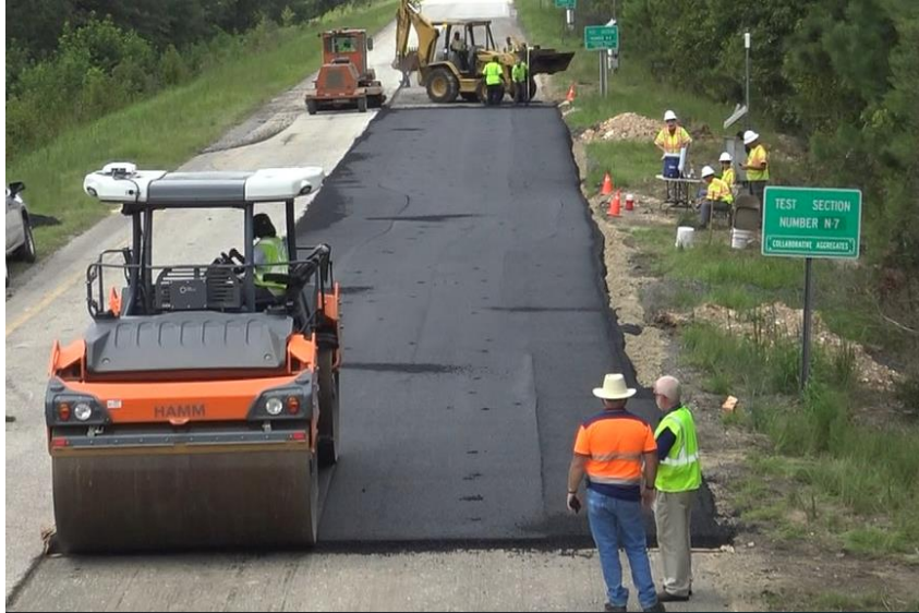
Figure 3.23: Start of Roller Compaction
