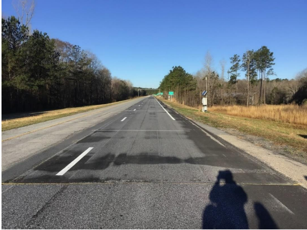
Figure 4.2: N1-GTRDry Section as of March 14, 2022
