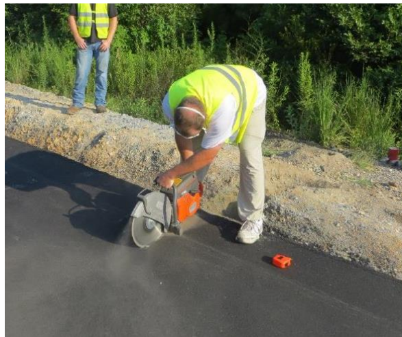
Figure 3.17: Saw Cutting Probe Slot (McCarty, 2020)
