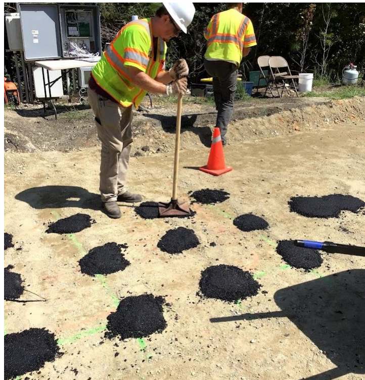
Figure 3.15: Compaction of the Gauge-Covering Mix
