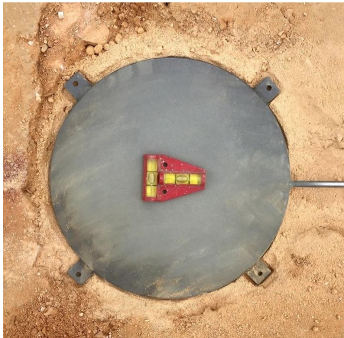
Figure 3.6: Leveled Subgrade EPC
