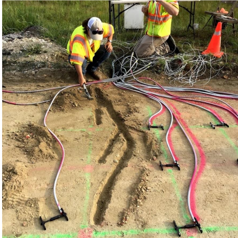
Figure 3.11: Digging Aggregate Base Trenches
