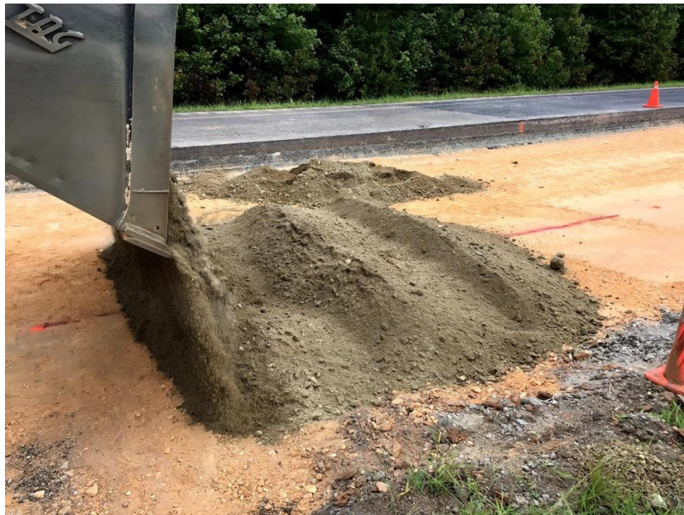
Figure 3.8: Aggregate Base Material Covering the Subgrade EPC
