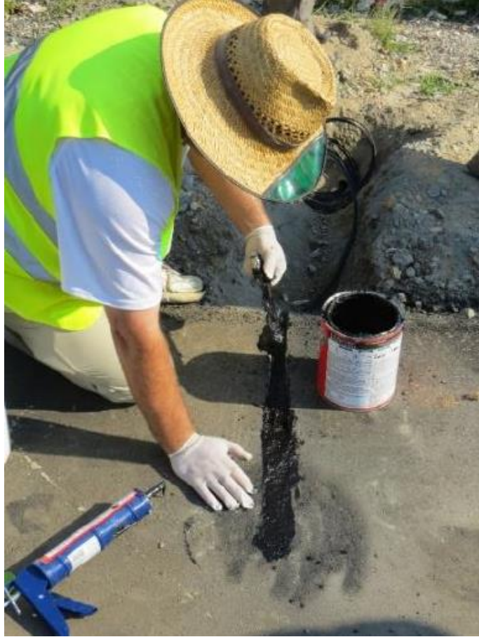
Figure 3.21: Roofing Cement Application Process (McCarty, 2020)
