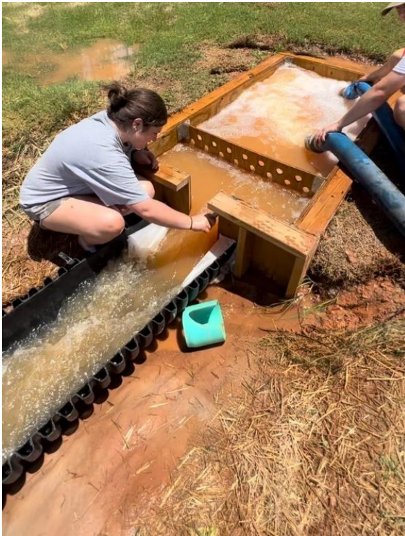
(a) surface weir box water depth measurement
