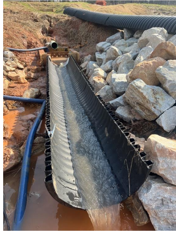
(b) modified swale underdrain weir box test
