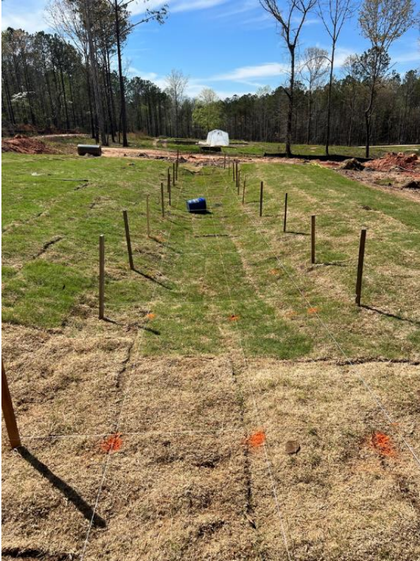
(a) wooden stakes and strings installation
