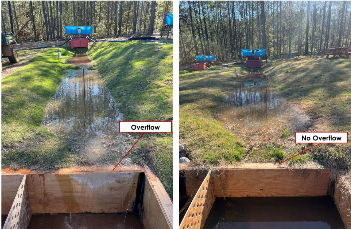
(a) overflow into the weir box
