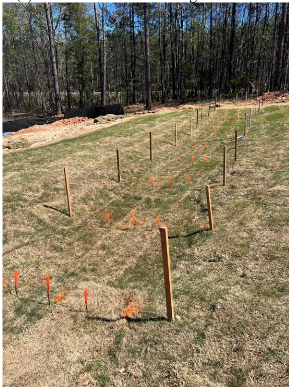
(c) orange steel nail installation
