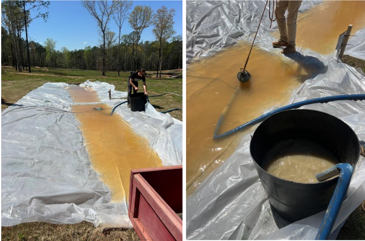
(a) dewatering surface water
