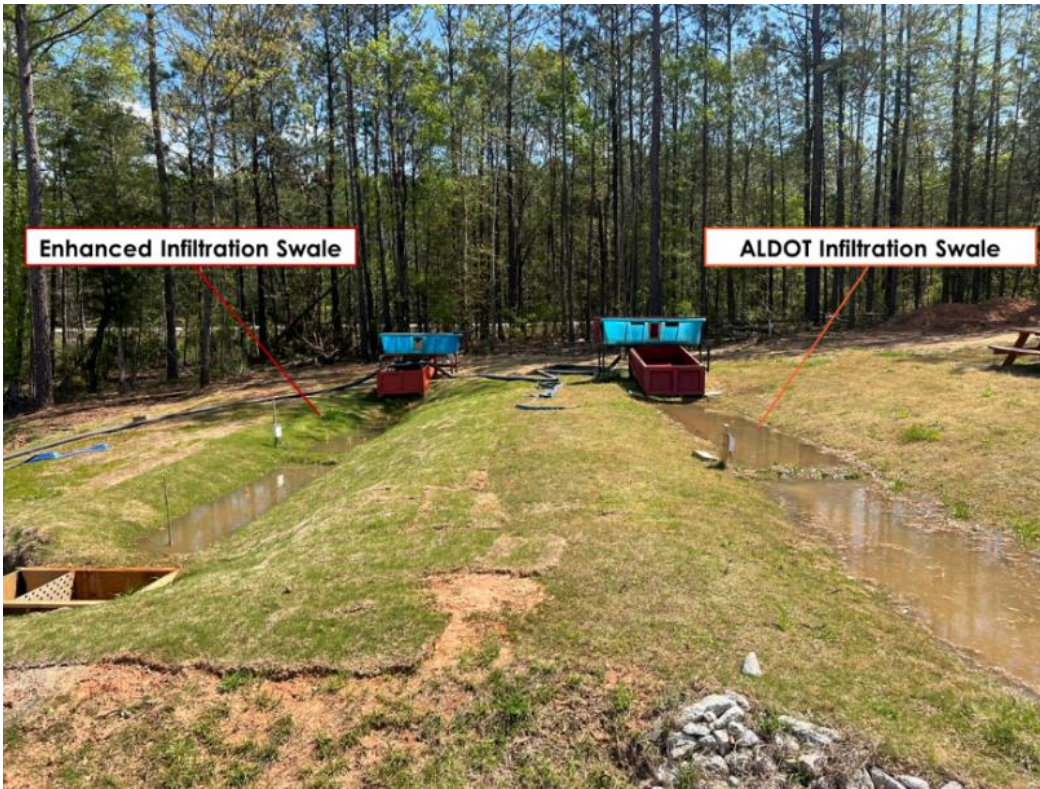
(a) view from the downstream
