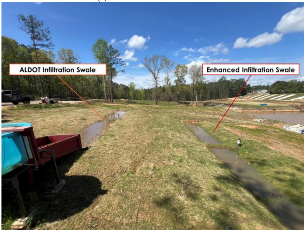
(b) view from the upstream
