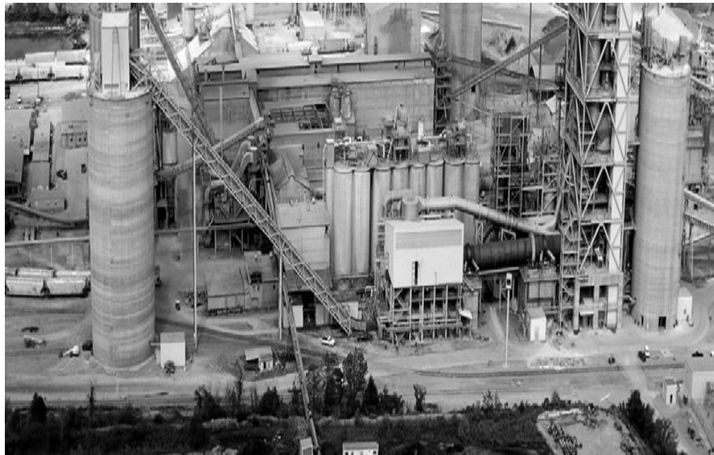
Figure 1.1: Full-scale portland cement production facility (Folta 2010)
