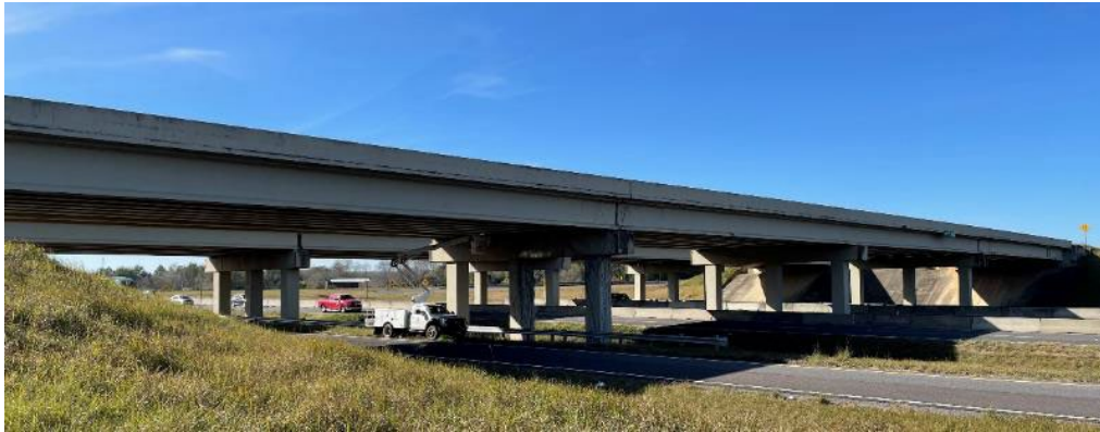
Figure 3-5: Elevation view of the Co Rd 39 bridge over I-10 (MOB-1)
