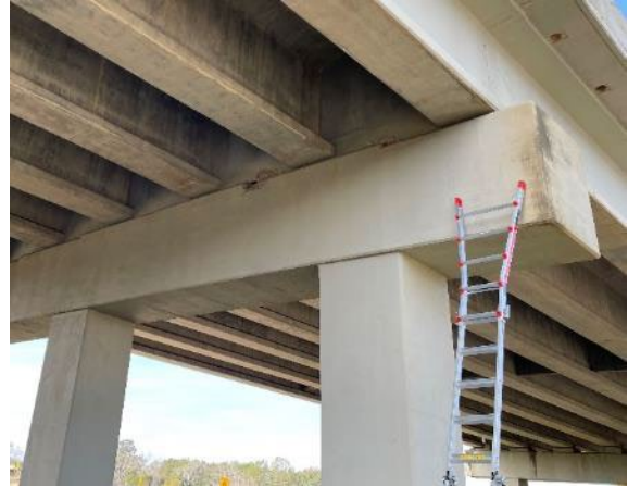
Figure A-5(o): Underside of bridge at Bent 3 (Northbound)
