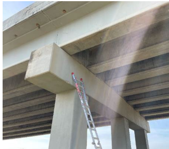
Figure A-5(i): Underside of bridge at Bent 3 (Southbound)
