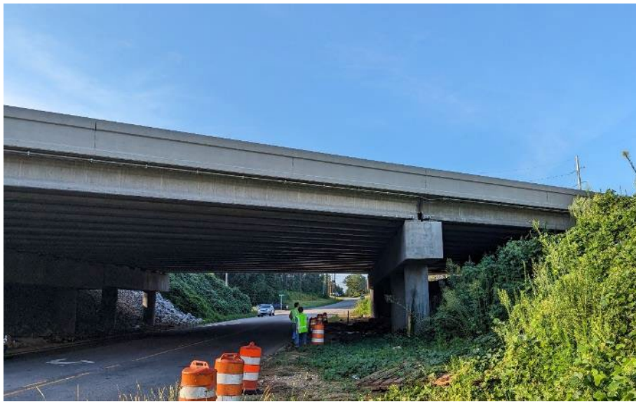
Figure 3-2: Elevation view of I-85 bridge over Co Rd 54 (LEE-1)
