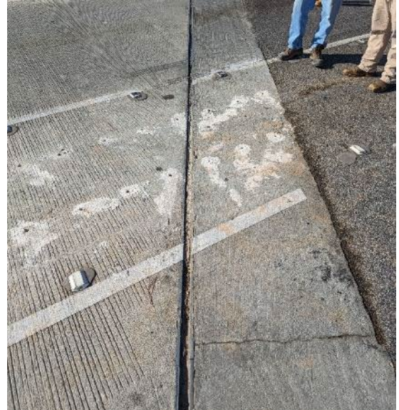
Figure A-1(c): Abutment expansion joint on Bent 1 (Construction Stage I)
