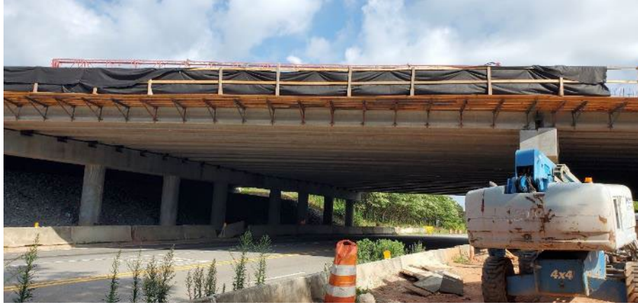
Figure 3-3: Elevation view of the I-85 bridge over SR-51 (LEE-2)
