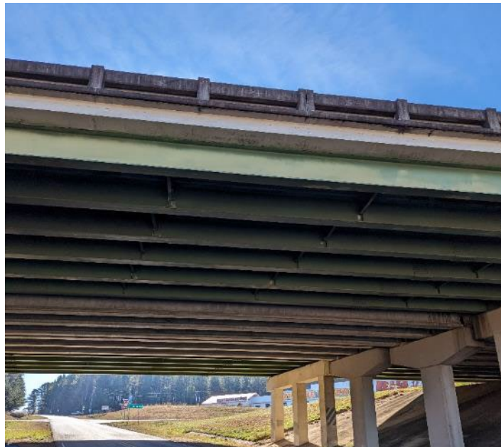
Figure 3-6: Elevation view of the I-20 bridge over Co Rd 49 (CLB-1)
