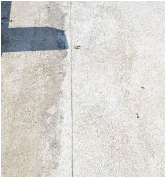
Figure A-2(d): Closed joint at Bent 2 (Construction Stage III)
