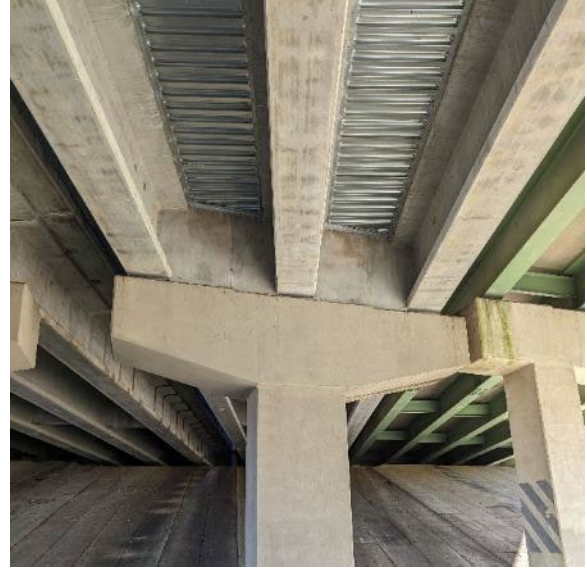
Figure A-4(k): Underside of bridge at Bent 2 (Eastbound)
