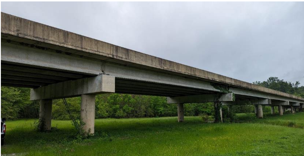
Figure 3-7: Elevation view of the US-11 bridge over Sucarnoochee River (SUM-1)
