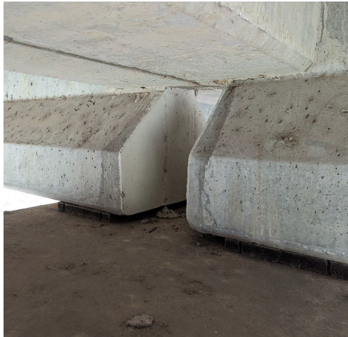
Figure 4-5: Bent 8 girder ends and expansion bearings
