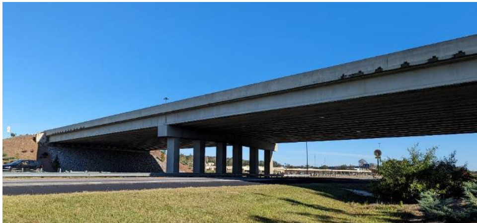
Figure 3-4: Elevation view of the Co Rd 10 bridge over I-85 (LEE-3)
