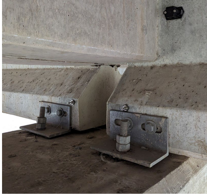
Figure 4-8: Bent 9 girder ends and fixed bearings
