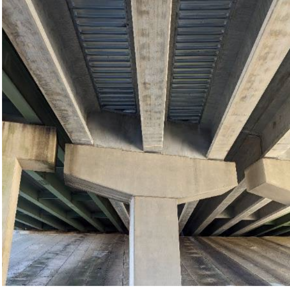
Figure A-4(j): Underside of bridge at Bent 2 (Westbound)
