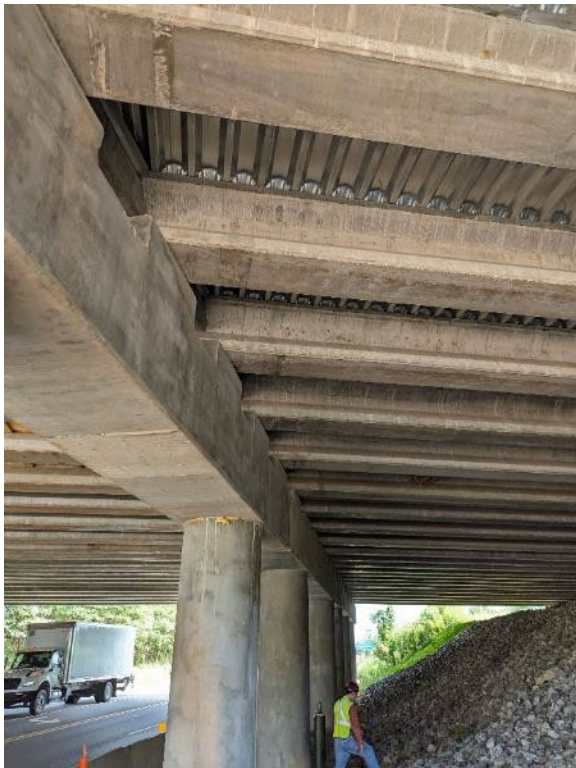
Figure A-2(h): Underside of bridge at Bent 3
