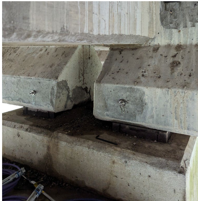
Figure 4-4: Bent 7 girder ends and expansion bearings
