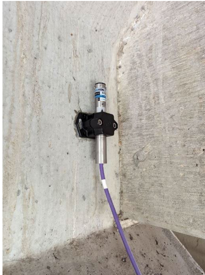
Figure 4-13: Inclinometer installation position (Bent 7 displayed)
