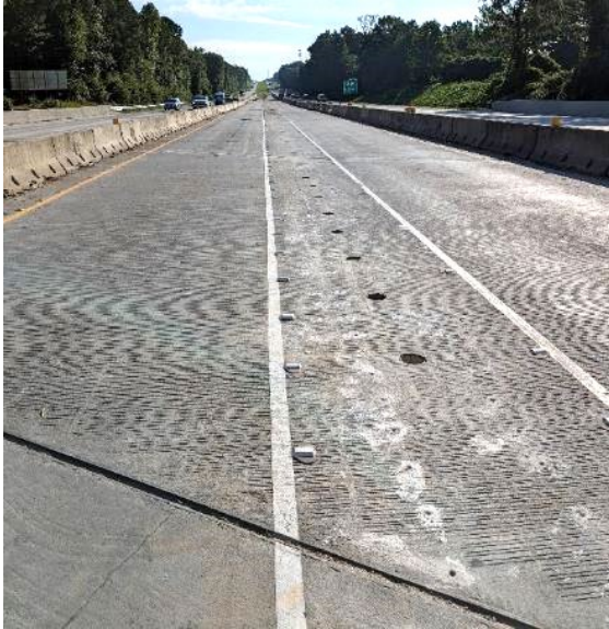
Figure A-1(b): Center portion of deck facing Northbound (Construction Stage I)
