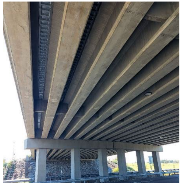
Figure A-3(i): Underside of bridge (facing Eastbound)
