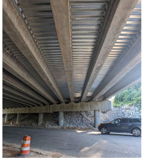
Figure A-1(k): Underside of bridge (facing Northbound)
