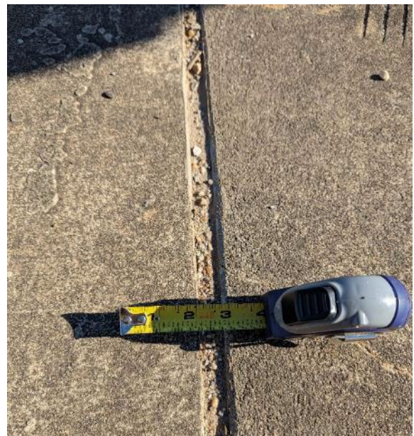
Figure A-3(e): Close-up of closed joint at Bent 2
