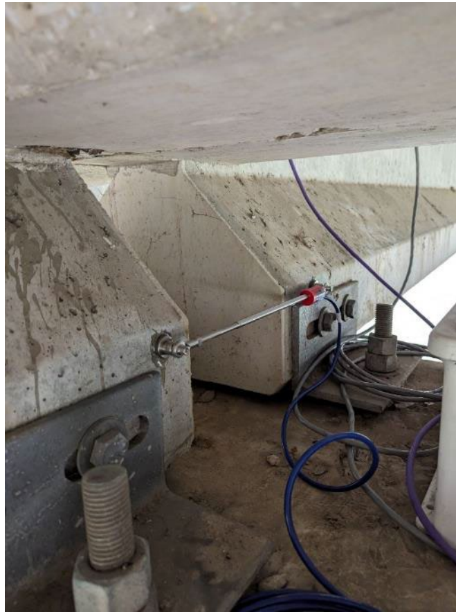
Figure 4-14: Crackmeter installation position (Bent 9 displayed)
