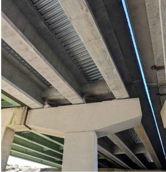
Figure A-4(n): Underside of bridge at Bent 3 (Eastbound)
