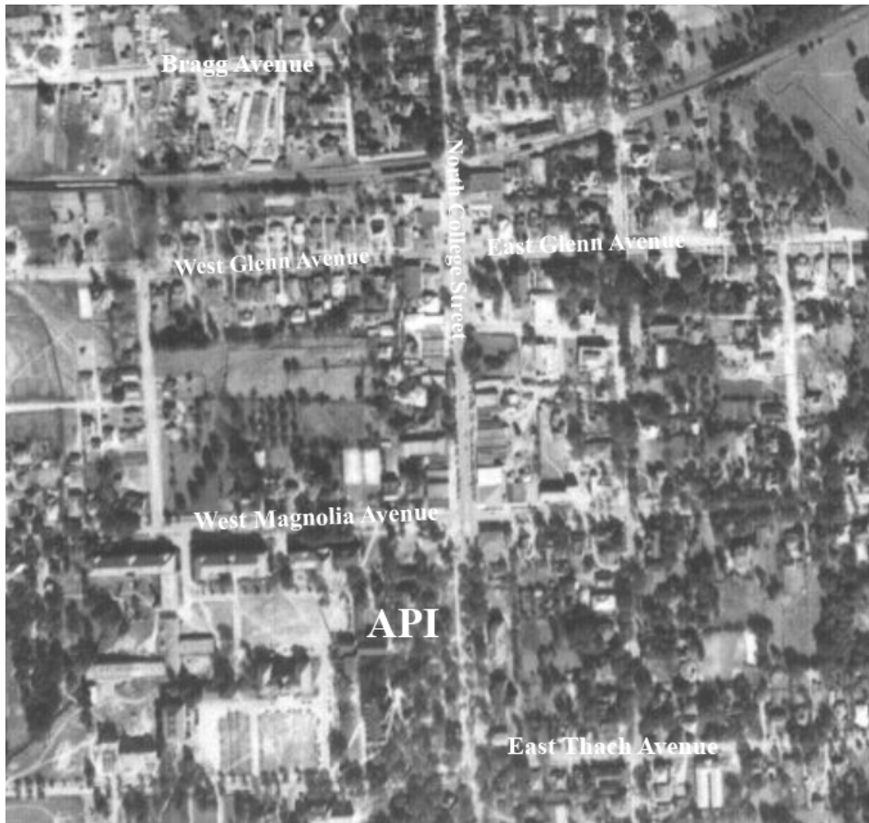
(Figure No. 17) 104 This aerial image depicts downtown Auburn, Alabama and a small portion of API's campus in 1939.
