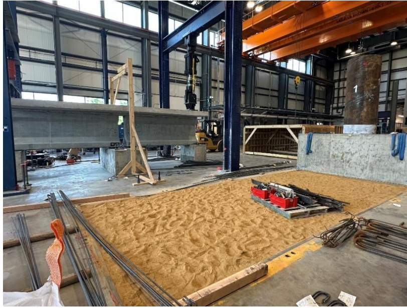
Figure 3-24. Compacted Sand in Geotechnical Chamber.
