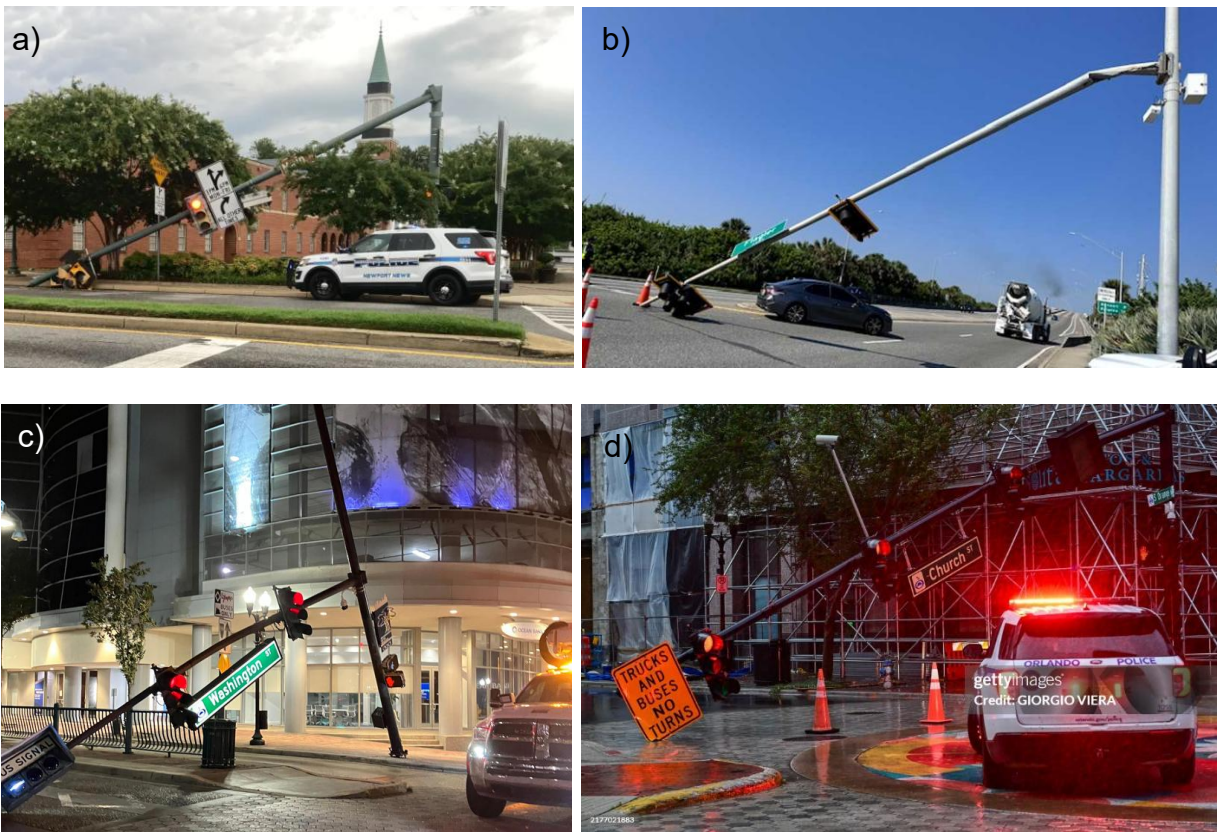
Figure 1-2. Mast Arm Failure in Florida: a) Newport News. Aug. 3, 2024 (The Virginian-Pilot, 2024), b) Flagler Beach, Aug. 14th, 2024 (FlaglerLive, 2024), c) Downtown Orlando, Hurricane Helene 2024 (MSN News, 2024), and d) Downtown Orlando, Hurricane Milton. Oct 10, 2024 (Getty Images, 2024)
