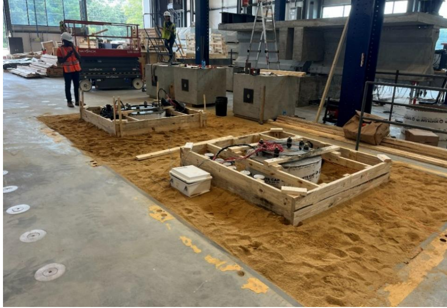
Figure 4-4. Both constructed shafts at the end of construction
