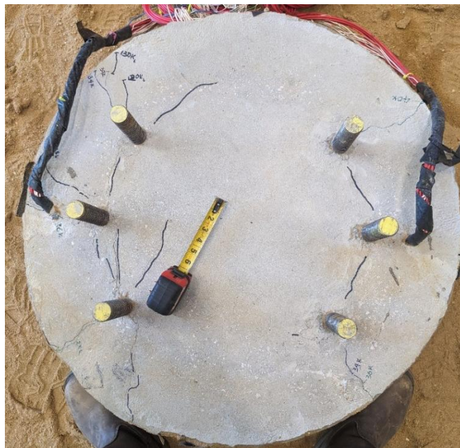
Figure 4-15. Cracks appeared at the surface of the shaft 2
