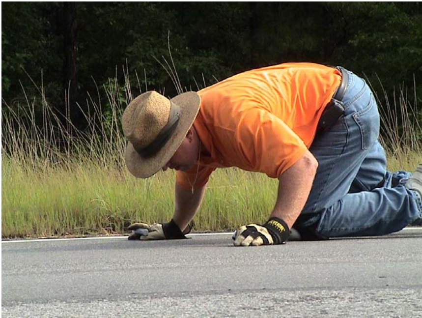
Figure 5-15. Crack Investigation Technique (Priest and Timm, 2006).
