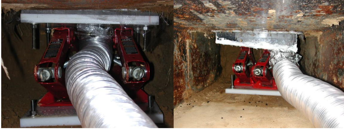
Fig. 4.4. Wick and pan lysimeters installed 50 cm below soil surface
