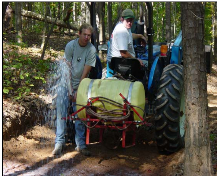
Figure 3.8 – Application of Envirotac II
