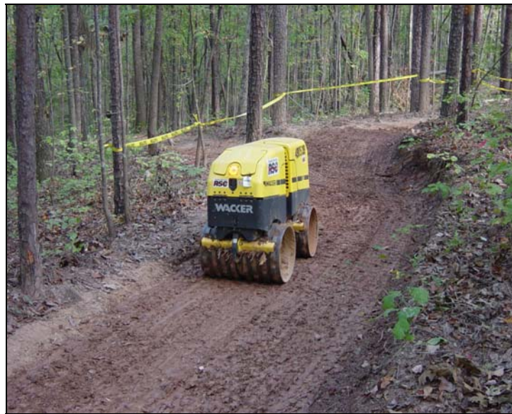
Figure 3.10 – Compaction of treated plot
