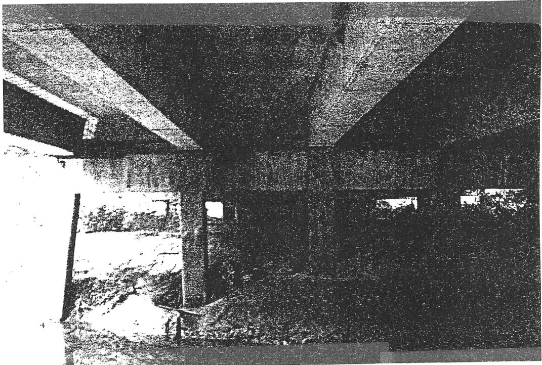
Figure 2.2 One-Story Bridge with Steel H-Pile Encased and Sway-Bracing Omitted
