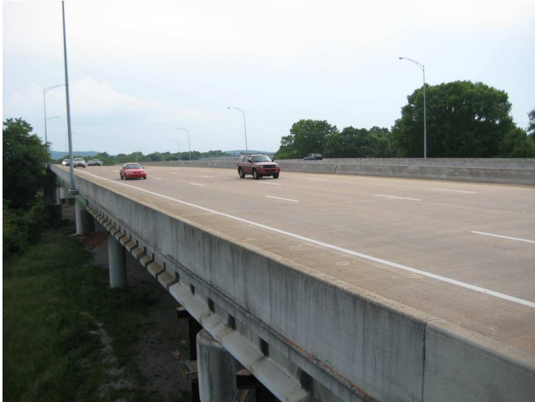
Figure F-1: View of I-565 bridge structure
