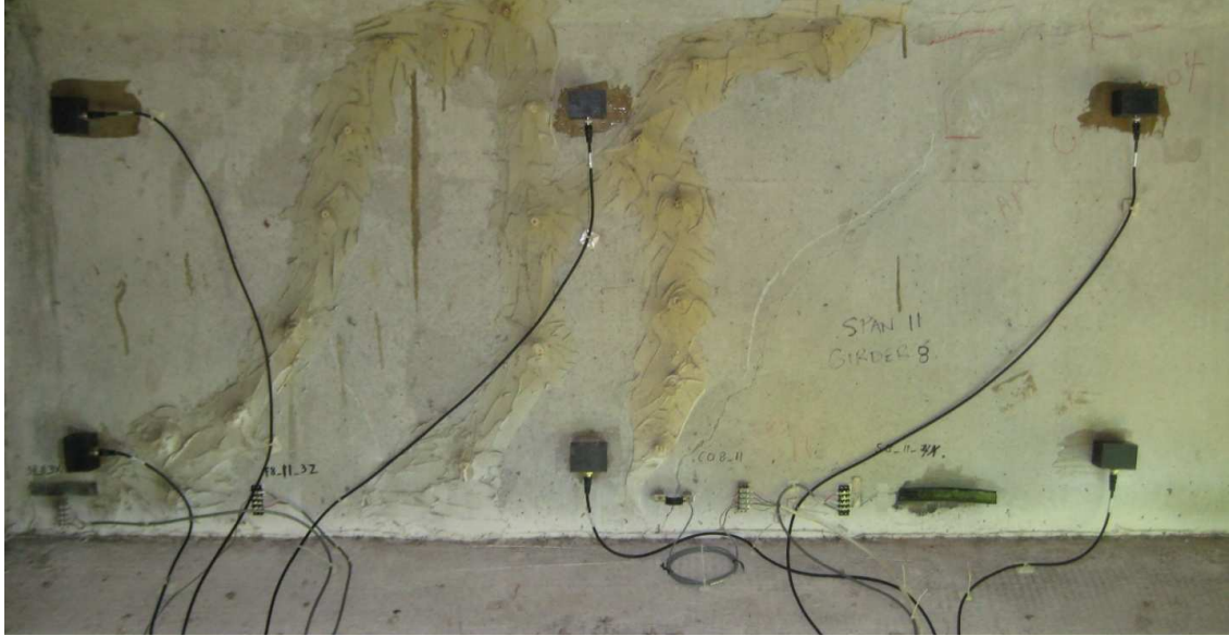
Figure 4-8: Arrangement of Sensors 13-18 on Girder 8
