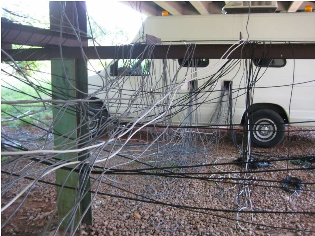
Figure F-5: Cables running from bridge girders to testing van
