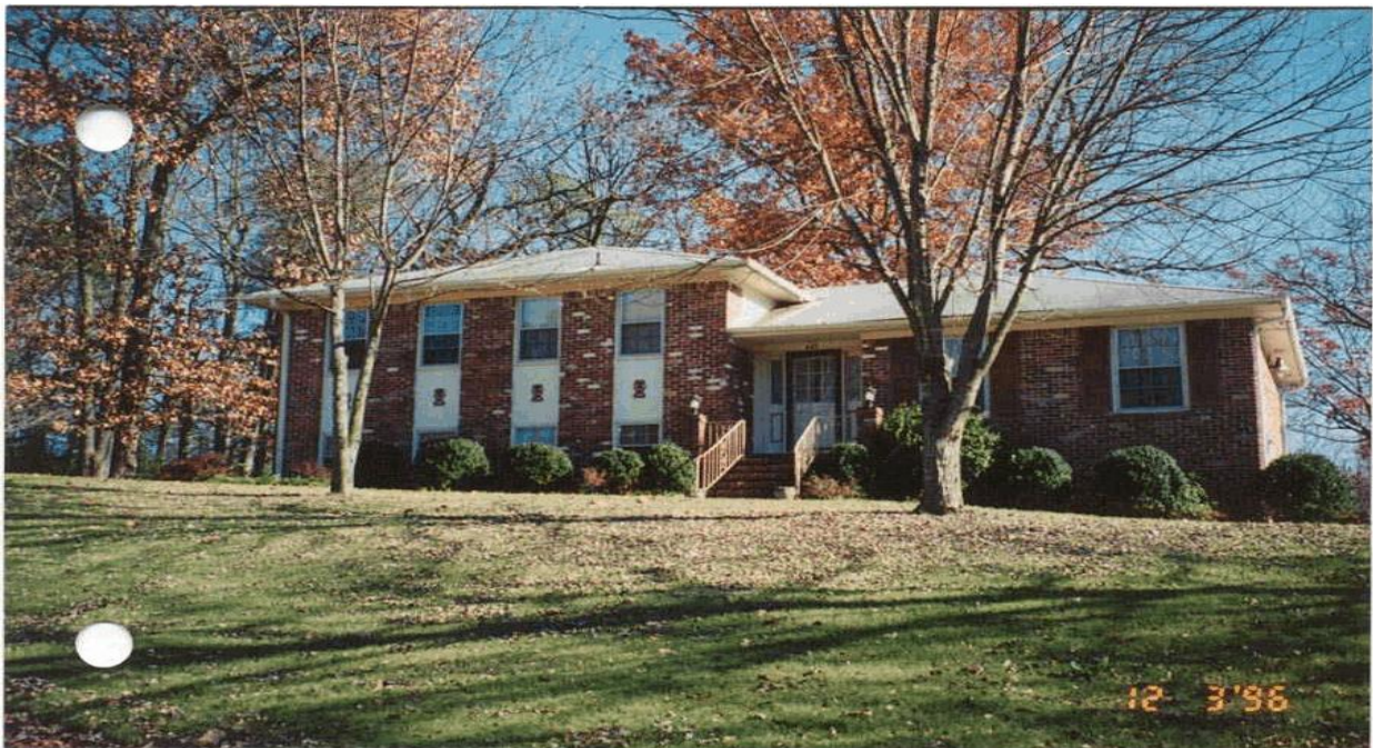
Figure 2—Home of Jack Swann After Renovations
