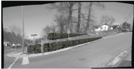
EROSION CONTROL . GABION WALLS - - - - ->
