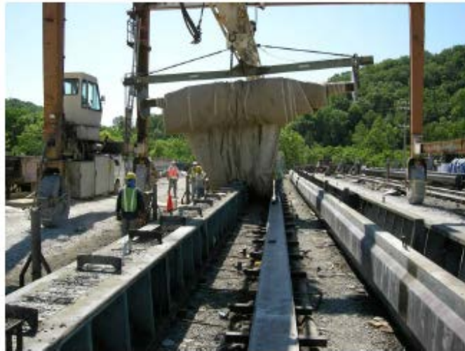
Figure 4-3: Placement of Curing Blankets (Boehm 2008)
