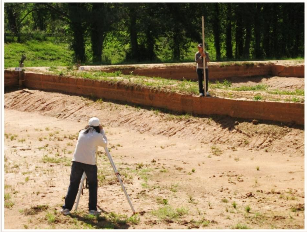
Figure 1. Concrete retaining wall in earthen ponds at the Auburn University E. W. Shell Fisheries Center, Auburn, Alabama.
