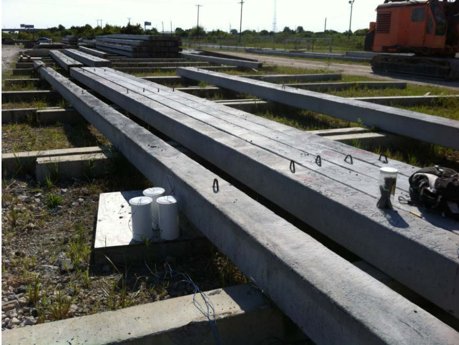
Figure 3.14. Outside storage of piles with temperature cylinders
