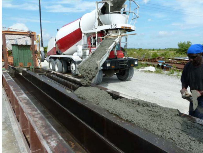
Figure 3.13. Placement of concrete in pile beds
