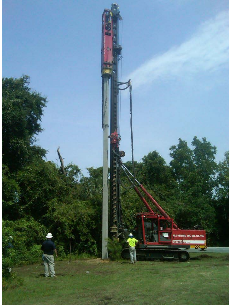
Figure 3.16. Junttan PM16 with HHK 4A pile hammer
