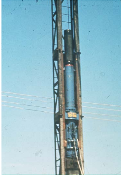
Figure 2.10. Open-ended diesel hammer (Likins 2005)
