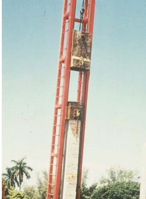
Figure 2.8. Crane hoisted drop hammer (Likins 2005)
