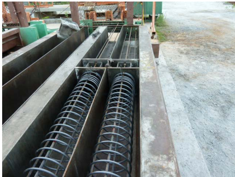
Figure 2.7. Prestressing beds prior to concrete placement
