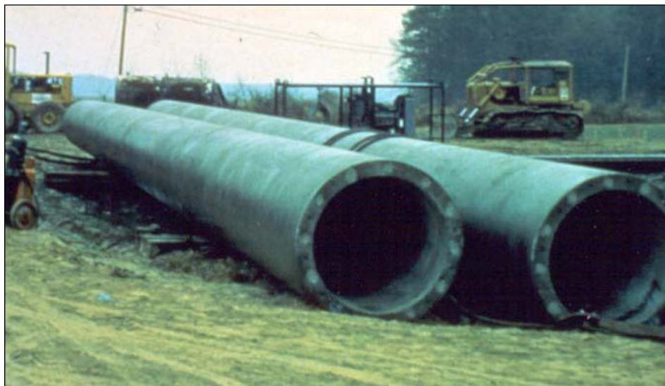
Figure 2.6. Spun-cast PCPS piles (Hannigan et al. 2006)
