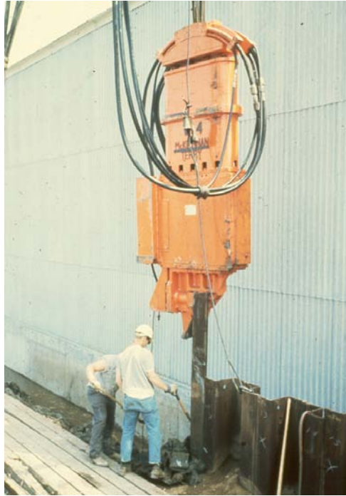
Figure 2.11. Vibratory hammer installing sheet piles (Likins 2005)
