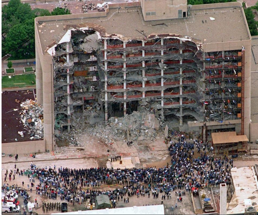
Figure 1.1 Structural Damage of the 1995 Oklahoma Building Bombing (AP Photo, Newman 2013)
