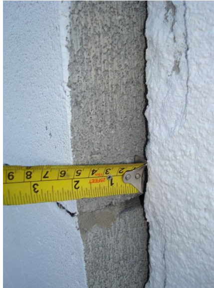
Figure 3.45: Wall 4 Pullout of the Frame
