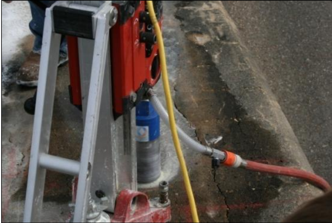
Figure A. 4. Close up of drilling process
