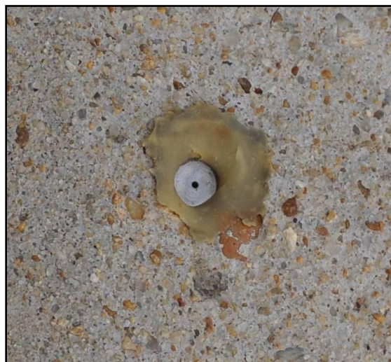
Figure 5.10. DEMEC stud installed in the Bibb Graves Bridge
