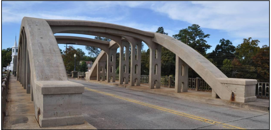
Figure 4.5. Span 5 after water-blasting (Warnock 2012)
