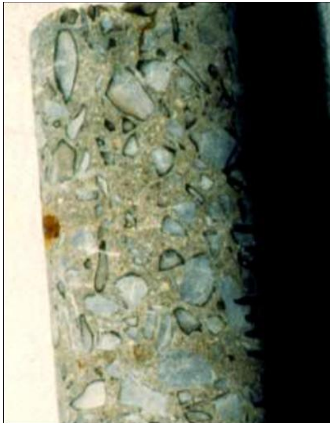
Figure 2.7. Dark rim around the perimeter of reactive aggregate particles
