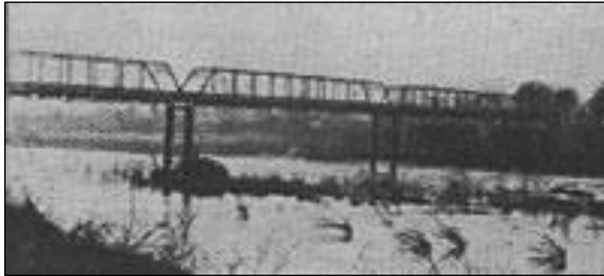
Figure 3.3. Iron bridge built in 1887 (Blackburn 1997)
