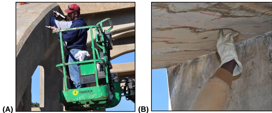
Figure 4.7. (A) Applying flexible sealant and (B) smoothing sealant by hand (Warnock 2012)
