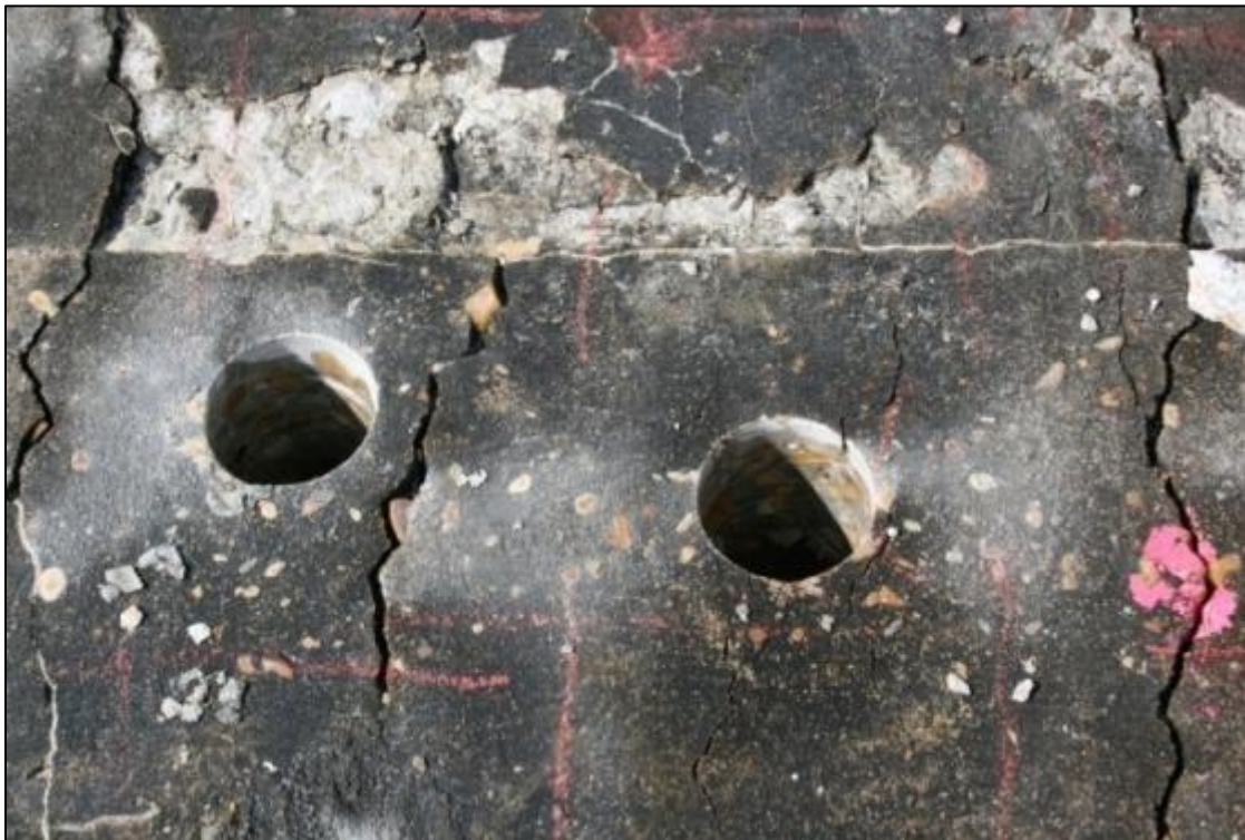
Figure A. 5. Core holes left after drilling
