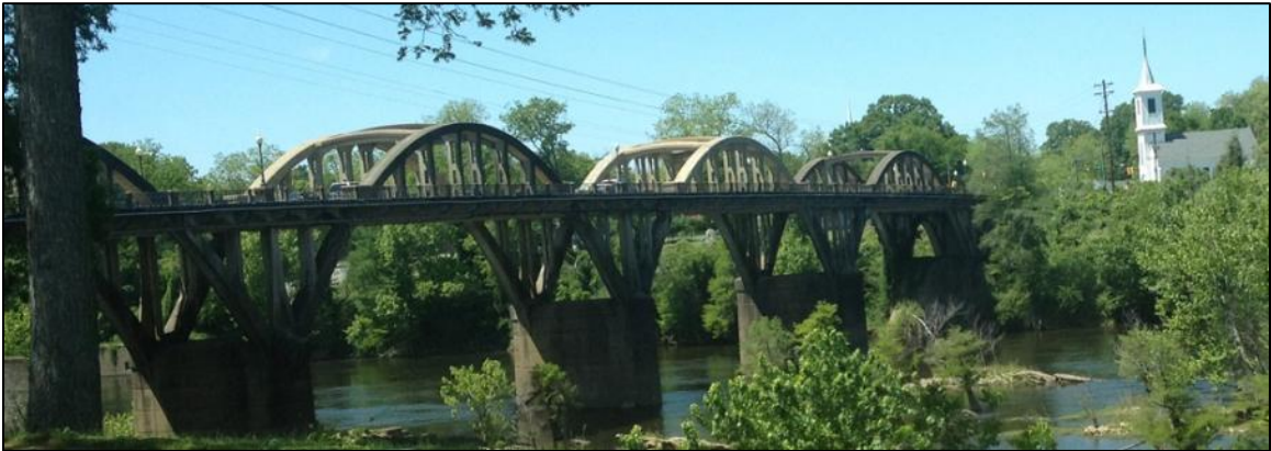
Figure 3.4. Northeast elevation view of the Bibb Graves Bridge
