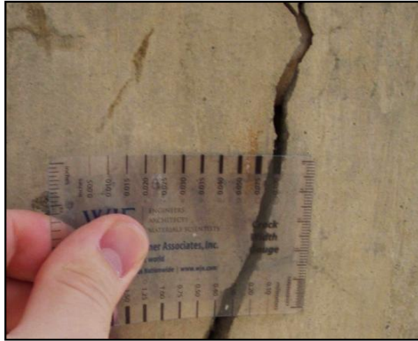
Figure 5.3. Using crack width gauge
