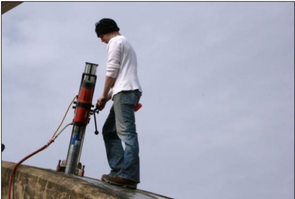
Figure A. 3. Drilling core sample
