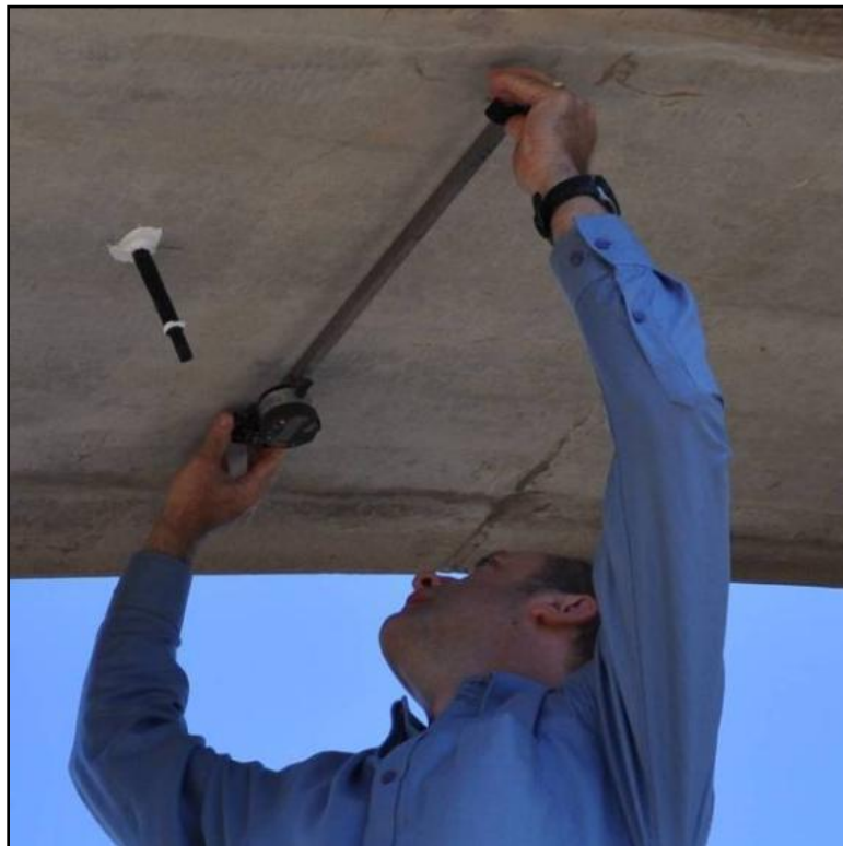
Figure 1.4. Taking a strain reading on the Bibb Graves Bridge (Warnock 2012)
