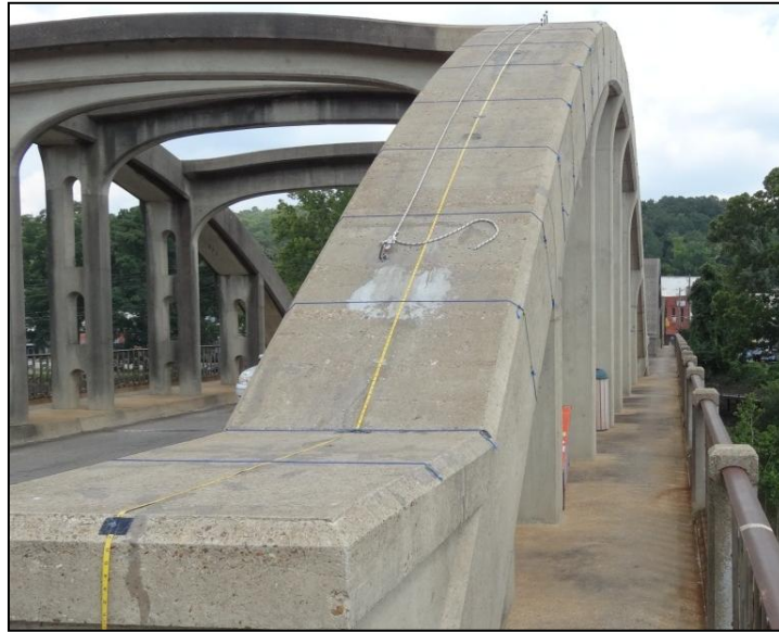
Figure 5.1. Grid for crack survey
