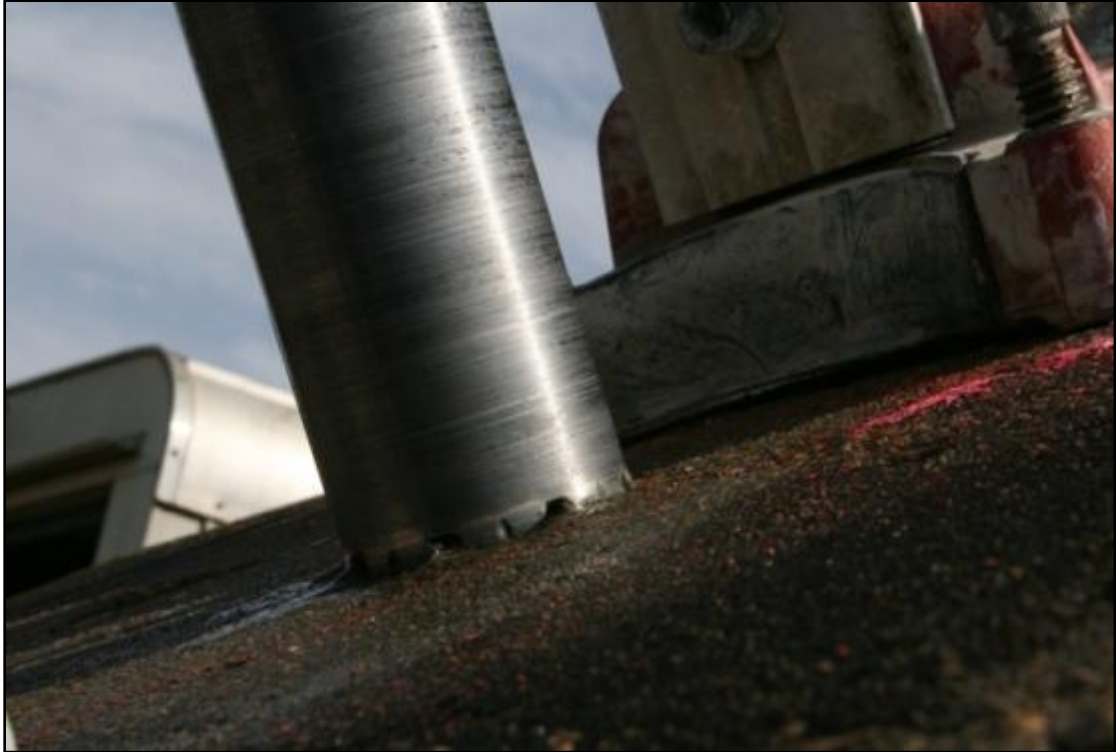
Figure A. 2. Close up of drilling set up
