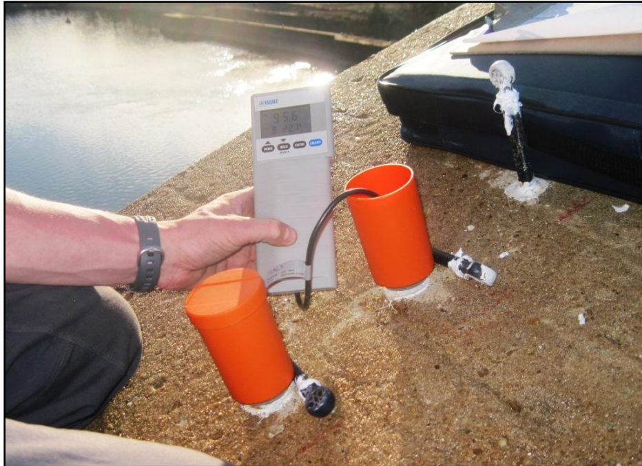
Figure 1.3. Measuring RH in Bibb Graves Bridge (Warnock 2012)
