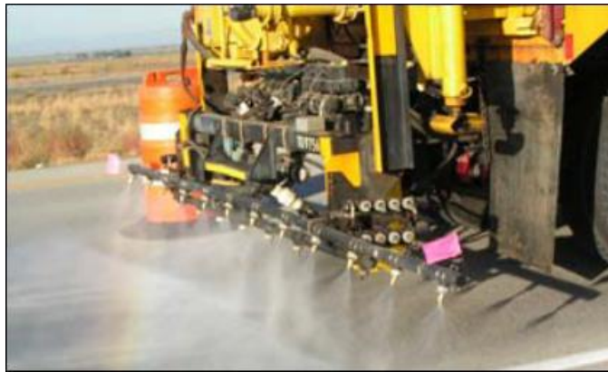
Figure 2.15. Topical application of 30% lithium solution to concrete pavement (Folliard et al. 2009)
