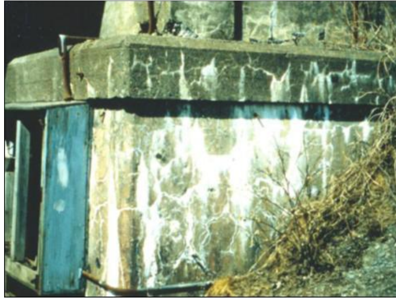
Figure 2.5. Efflorescence and exudations of alkali-silica gel on a foundation (Fournier et al. 2010)
