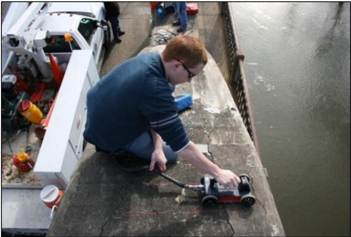
Figure A. 1. Use of ground penetrating radar to locate reinforcement
