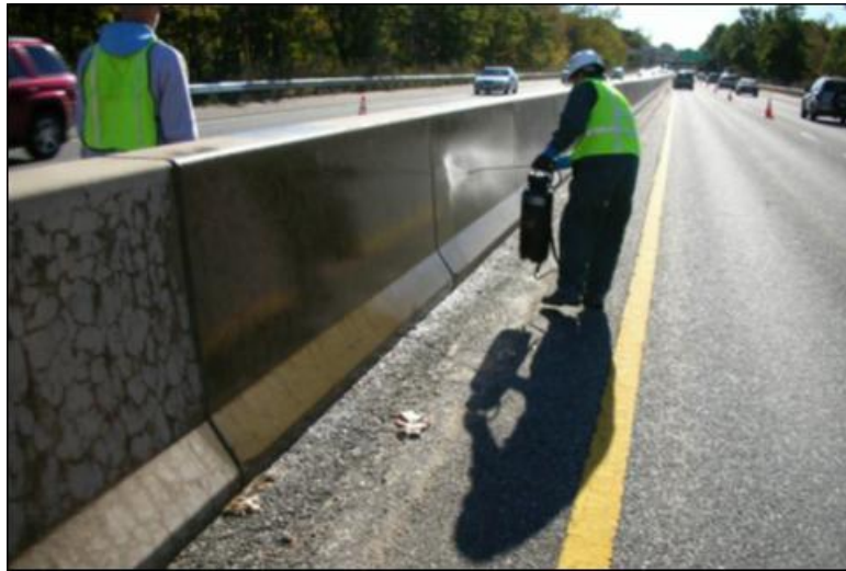
Figure 2.8. Topical application of 40% silane solution to ASR-affected barriers (Fournier et al. 2010)
