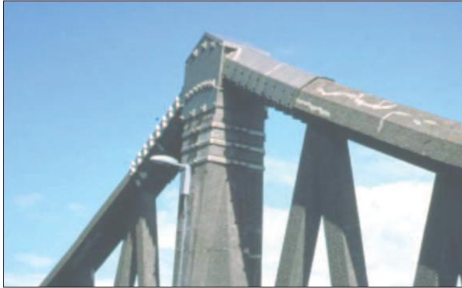
Figure 2.19. Montrose New Bridge repair with confinement and cladding (Fournier et al. 2004)
