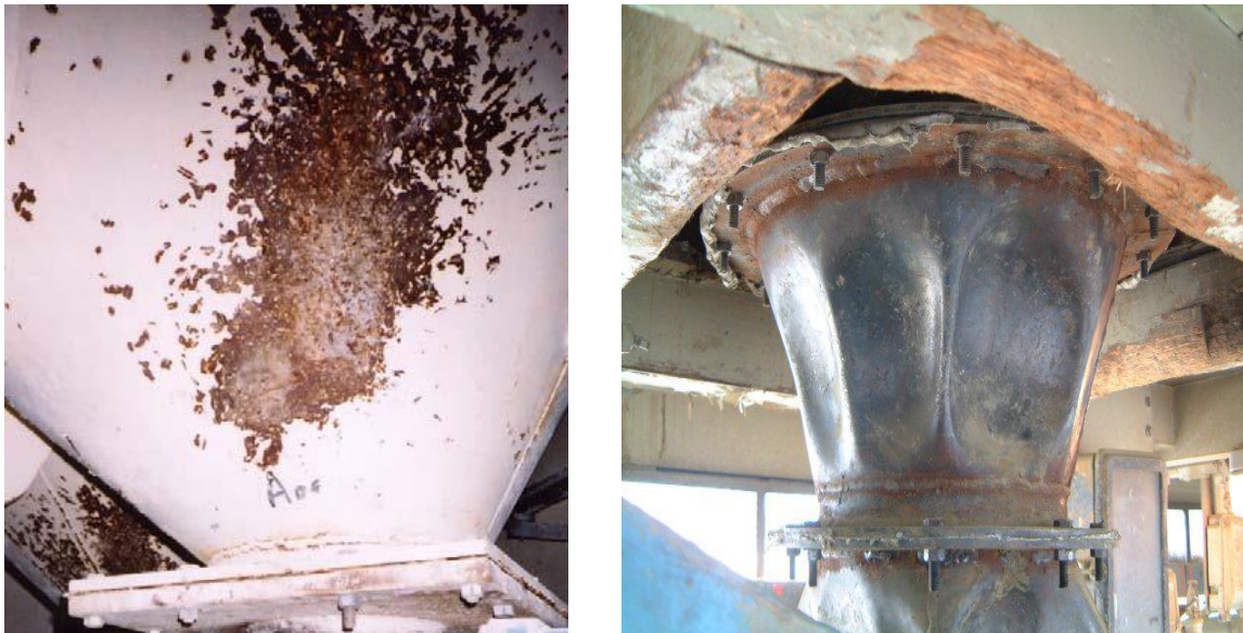
Figure 1.1: Hammer rash on bins with flow problems (Source: Bradley et al., 2011).
