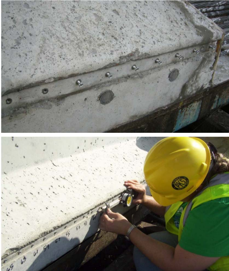
Figure 4.2: DEMEC insert ( top ) installation within DEMEC mounting strips and ( bottom ) measurement using a DEMEC strain gauge
