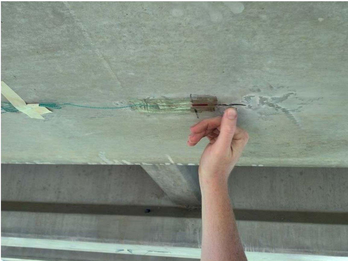
Figure 7.1: Strain gauge applied to bottom surface of girder at midspan
