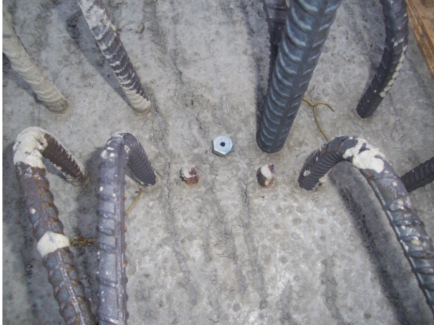
Figure 6.9: Surveying target embedded in top surface of girder
