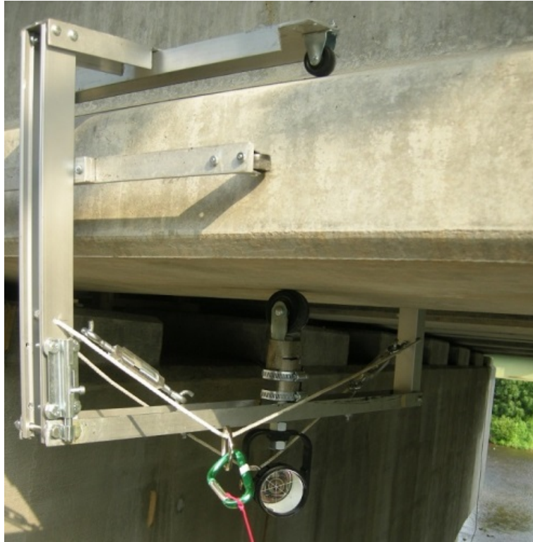
Figure 6.10: Apparatus used to survey underside of girders during construction
