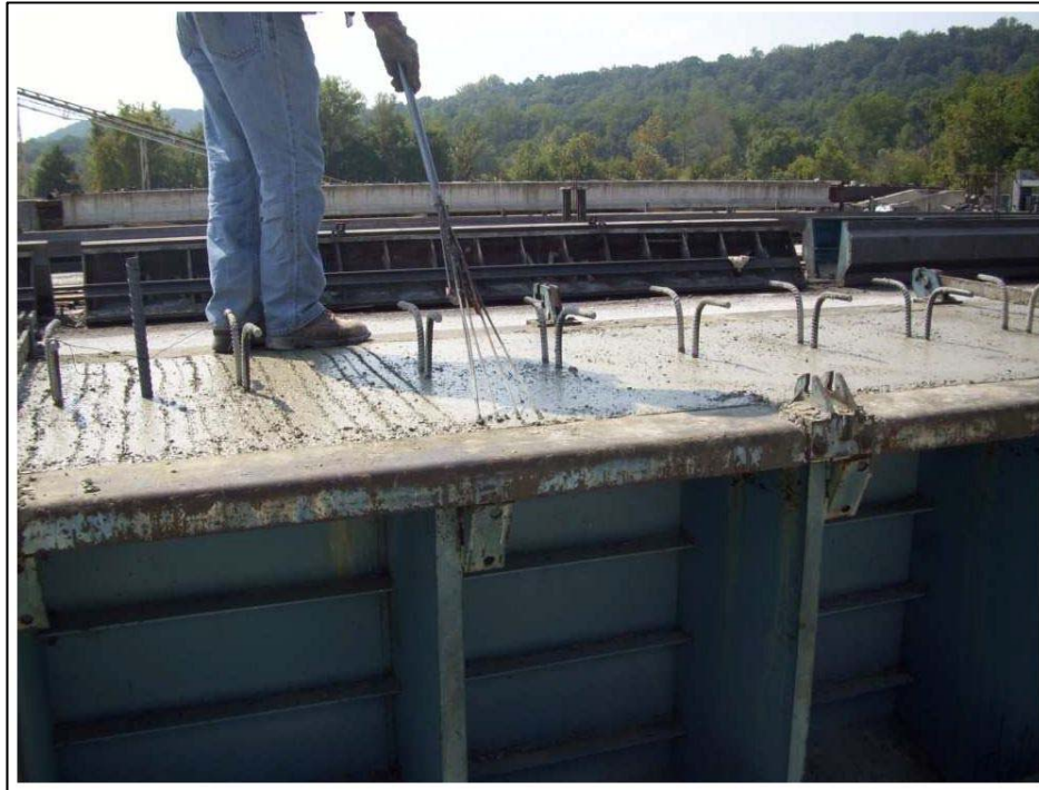
Figure 3.14: Application of transverse, top-surface roughening with a metal rake
