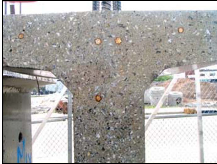
Figure 2.8: Saw-cut cross section of a bulb-tee girder digitally analyzed for hardened concrete constituent distribution (Khan and Kurtis 2010)
