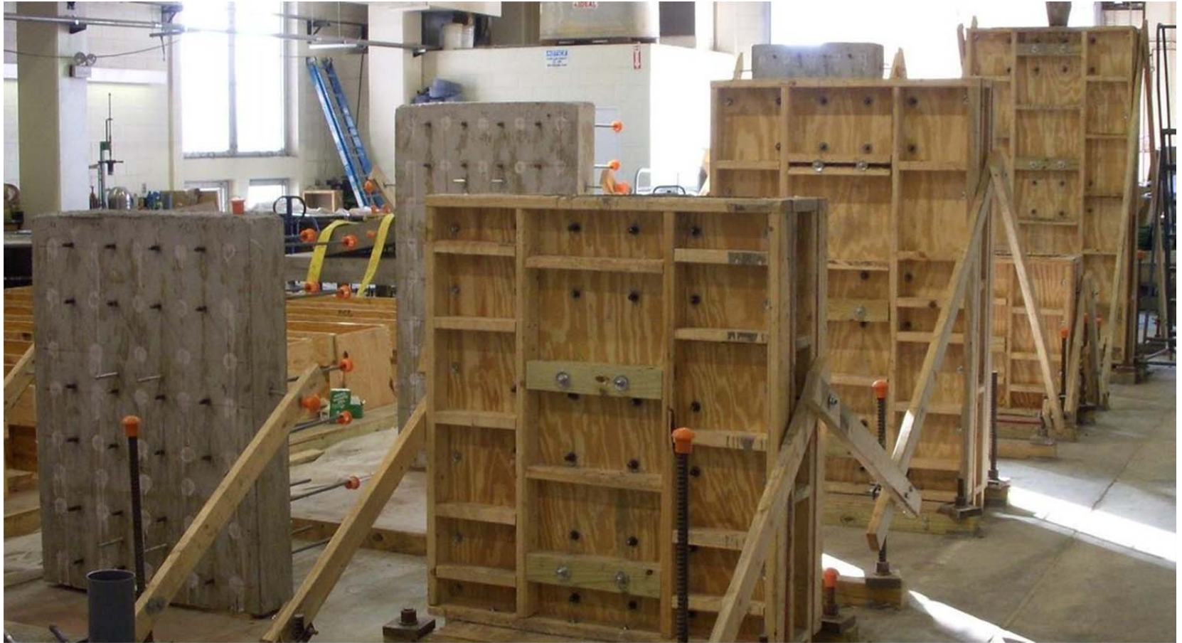
Figure 2.41: Parallel lines of cast walls and formwork
