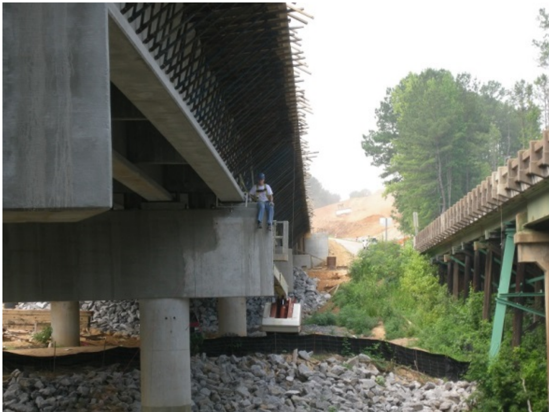
Figure 1.1: AUHRC personnel monitoring girder performance during bridge construction
