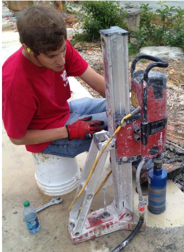
Figure 3-26: Drilling of a Core from the Exterior Region of a Slab
