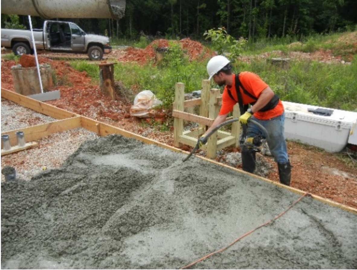
Figure 3-17: Internal Vibration of a Slab
