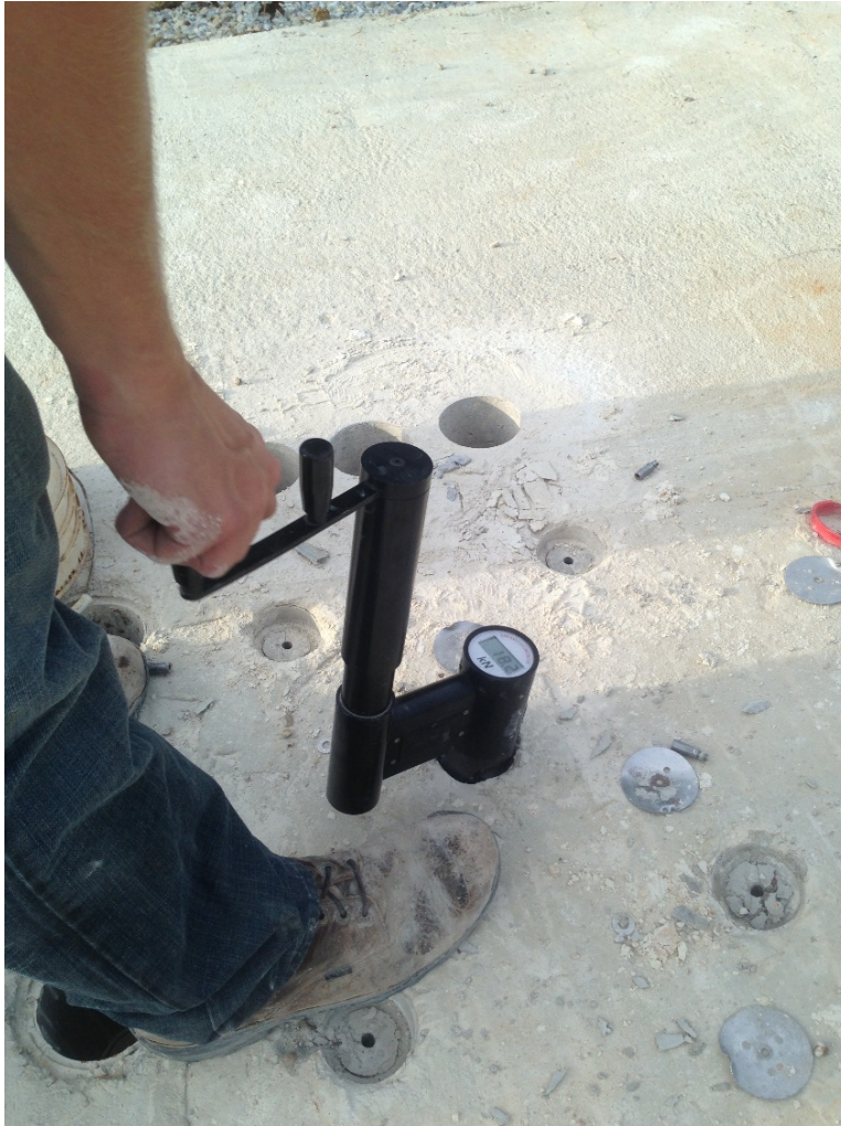
Figure 3-31: Pullout Test Being Performed
