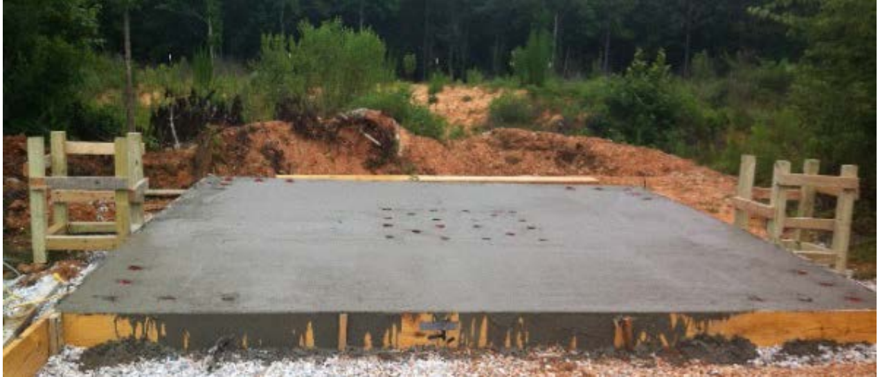
Figure 3-18: A Completed Slab
