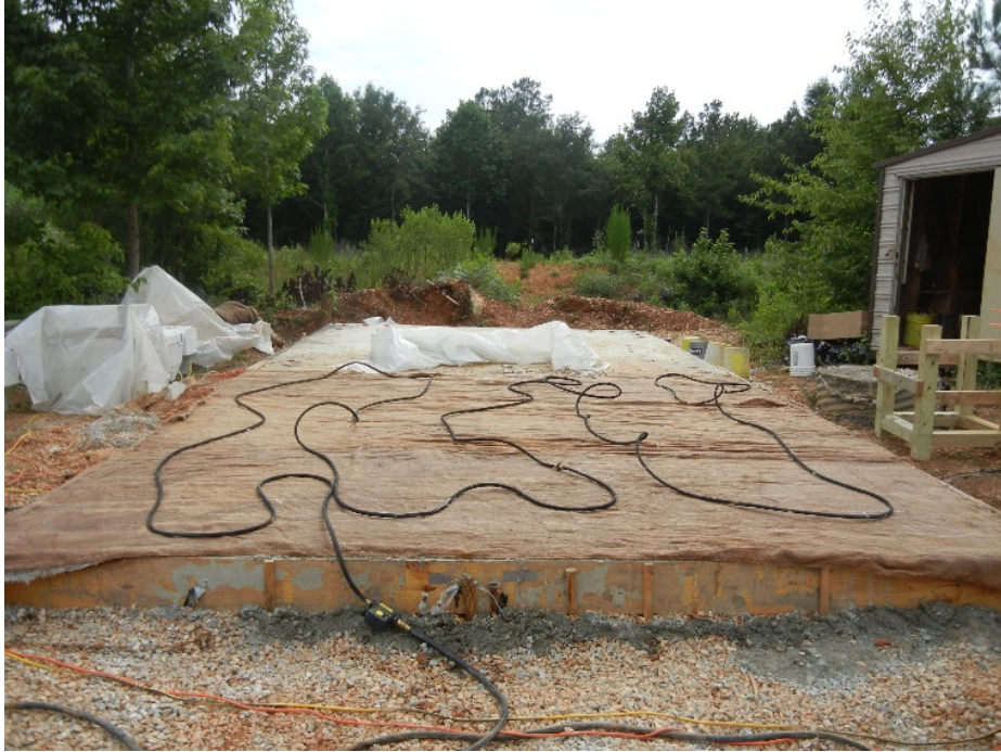
Figure 3-19: Curing Mats and Soaker Hoses
