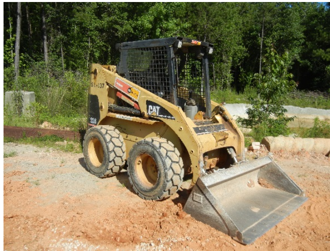
Figure 3-7: Skid-Steer Used for Site Work
