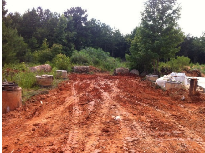
Figure 3-9: Second 15 ft × 60 ft Area After Clearing
