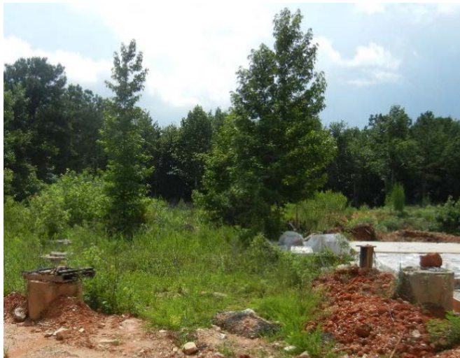
Figure 3-8: Second 15 ft × 60 ft Area Before Clearing
