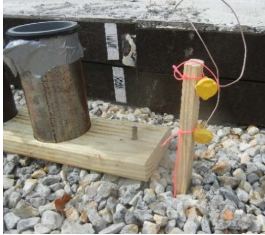
Figure 3-12: Placement of iButton Sensors in a Slab
