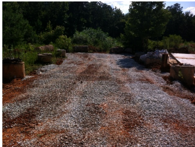
Figure 3-10: Second 15 ft × 60 ft Area After Placement of Sub-Base
