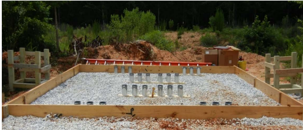
Figure 3-11: Typical Setup before Placement
