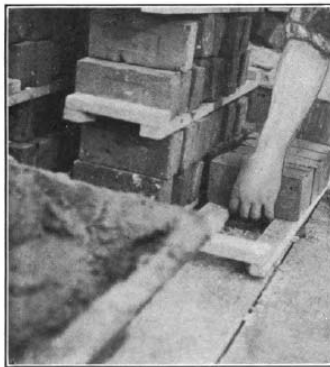
Figure 5.5 Instructed Method of Picking up Brick from Lower Tier (Gilbreth 1911)
