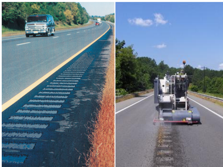
FIGURE 2.5 Milled-in rumble strips
