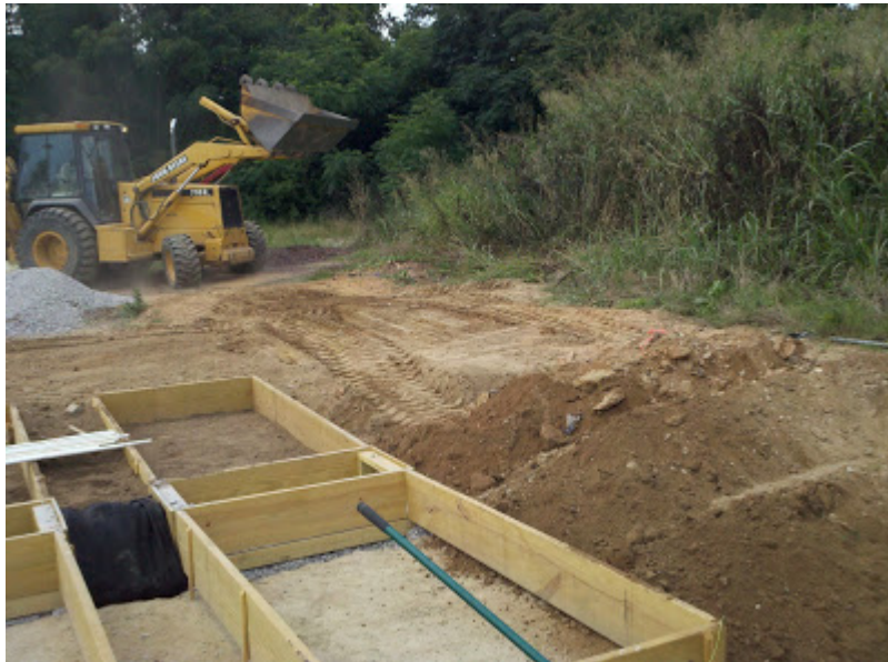
Figure 7. Backfilling in the site
