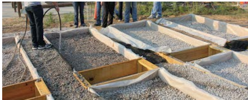
Figure 8. Flushing water to remove fines
