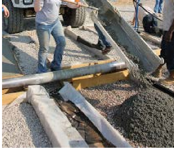
Figure 10. Pouring of pervious concrete
