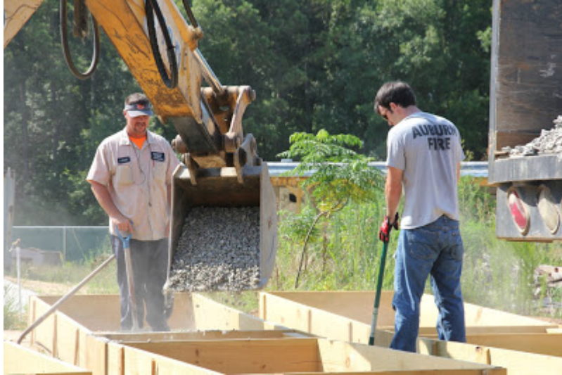
Figure 6. Placing of #57 Stone.
