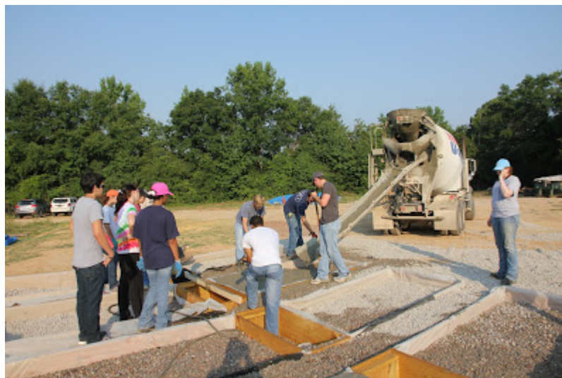
Figure 9. Pouring of traditional concrete
