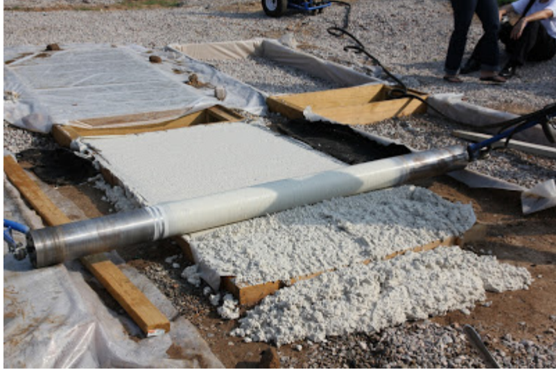
Figure 11. Placing of traditional photocatalytic concrete
