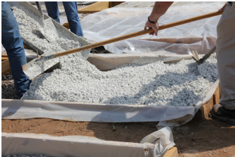
Figure 12. Placing of pervious photocatalytic concrete
