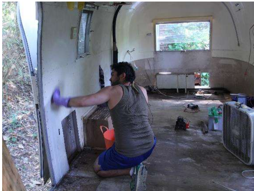
Figure 27: Cleaning Interior Walls
