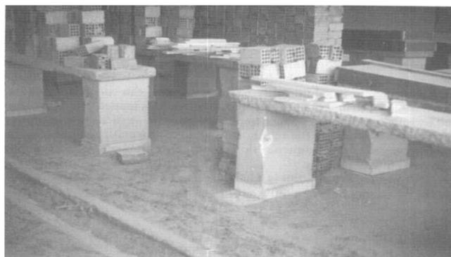
**Figure 2-12: A Bench which has Displaced Horizontally without Friction at the Interface (Papazoglou & Elnashai, 1996)**
