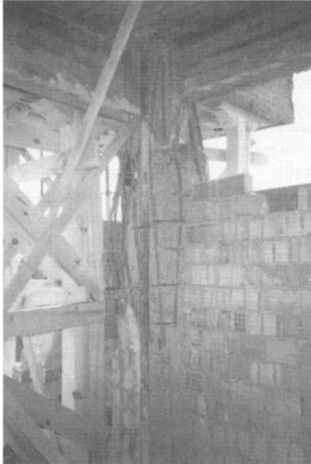
**Figure 2-13: Compressive Column Failure in a Residential Building in Kalamata. (Papazoglou & Elnashai, 1996).**
