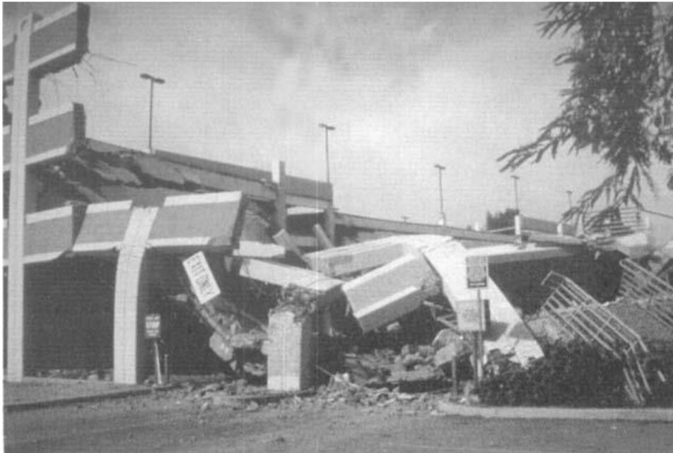
**Figure 2-16: Collapsed CSUN Parking Structure. The Perimeter Frame does not Show Signs of Distress where Gravity System has not Failed. (Papazoglou & Elnashai, 1996).**
