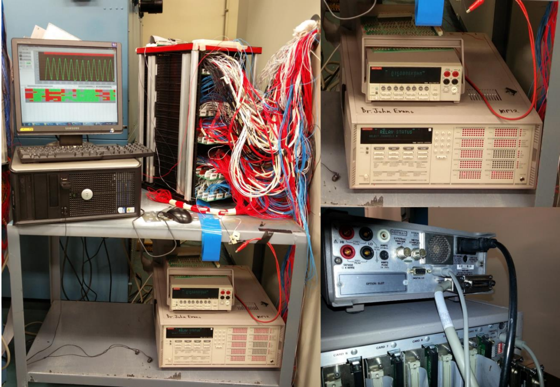
Figure 5.23. Monitoring System for the TC1-SRJ experiment (24A Group, LHS).
