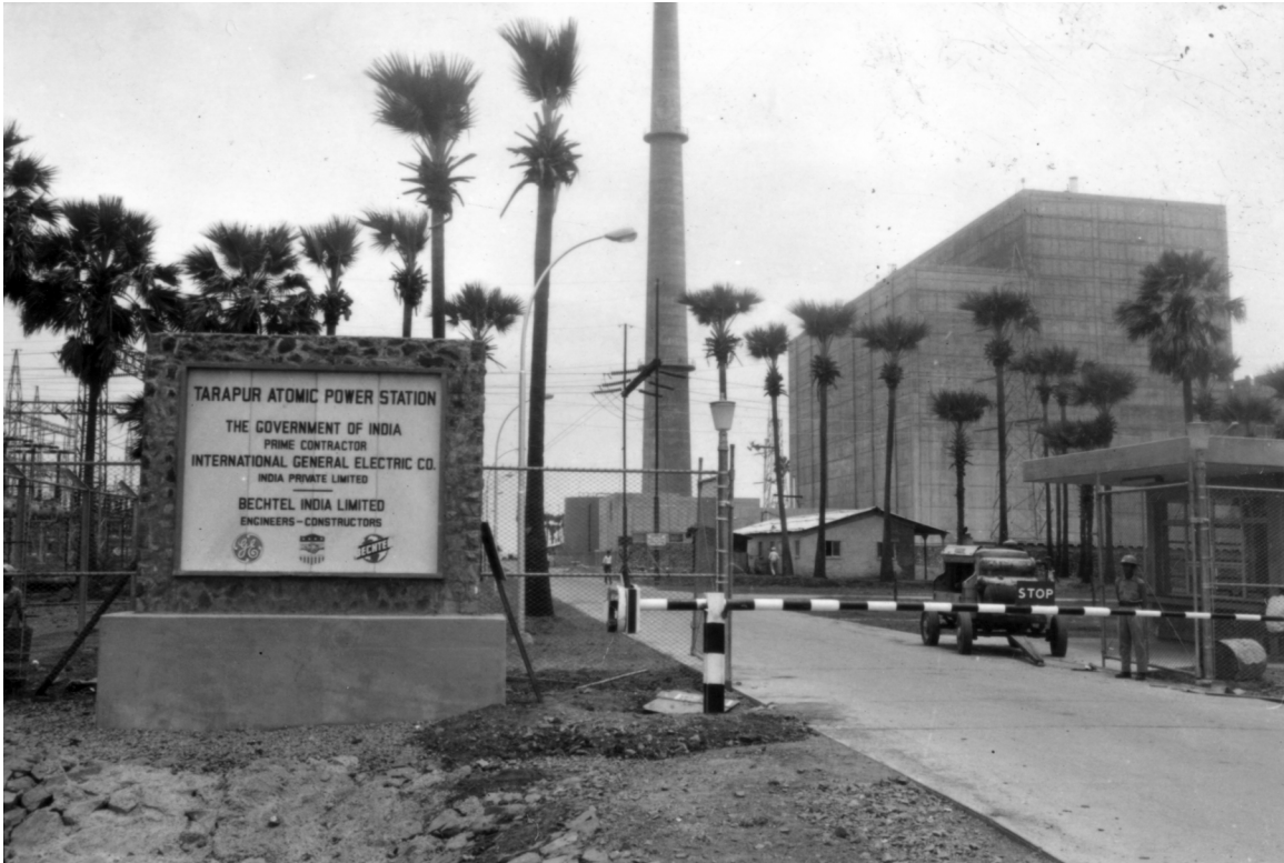
Figure 12. The main gate of the Tarapur Atomic Power Project site, ca. 1969. The ventilation stack and reactor building are visible in the background. (Source: Photographs of Assistance Programs in Foreign Countries, RG 286-CP, NARA.)
