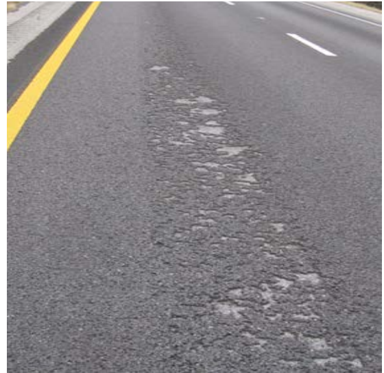
Center of Paver Streak (b)
