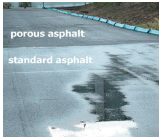
Figure 4 – Illustration of Water Transport on PFC and Dense-Graded Mixes (Porous Pavement)
