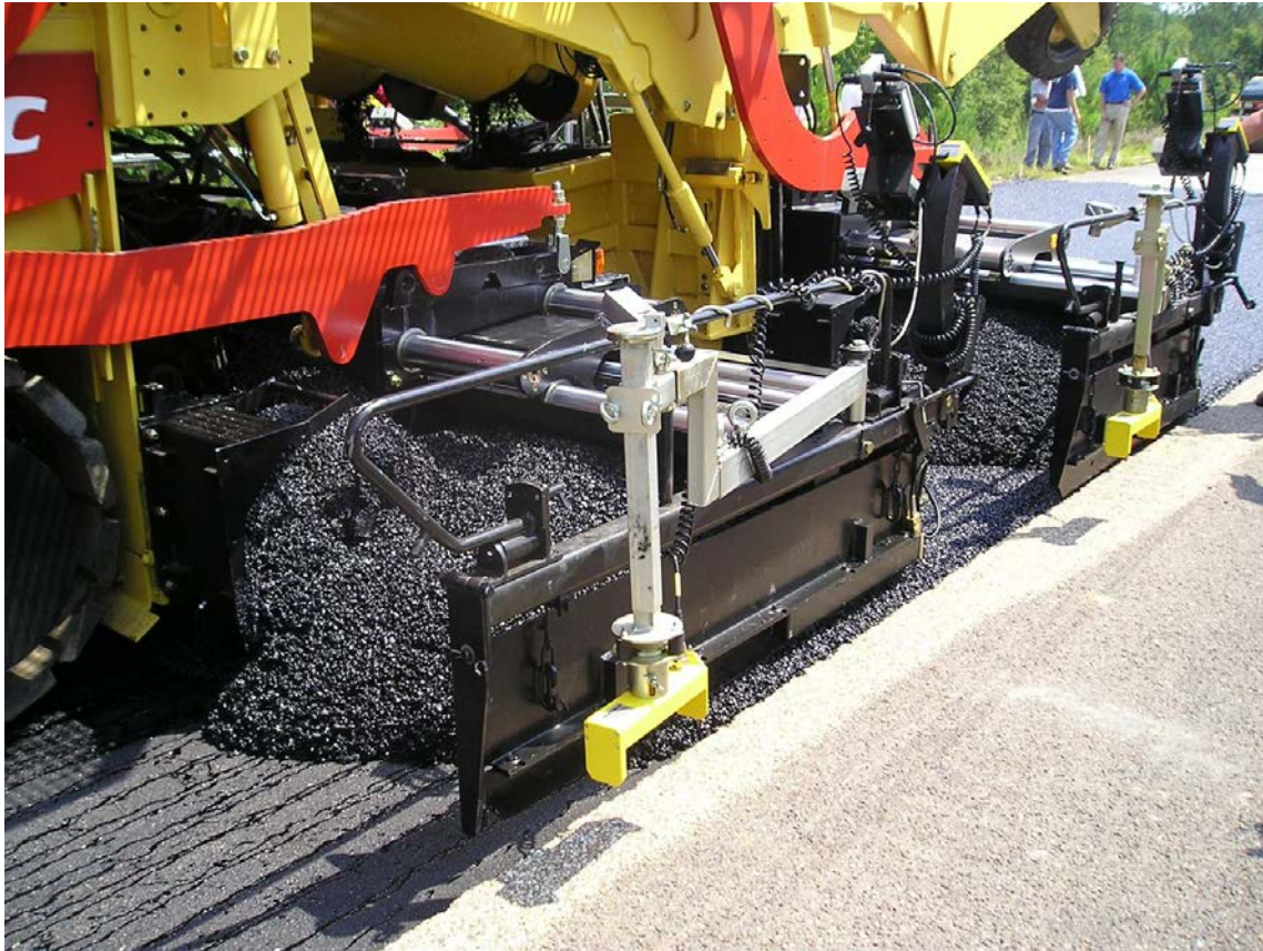
Figure 26 – Imported European Dual Paver for Twinlay PFC at NCAT Test Track
