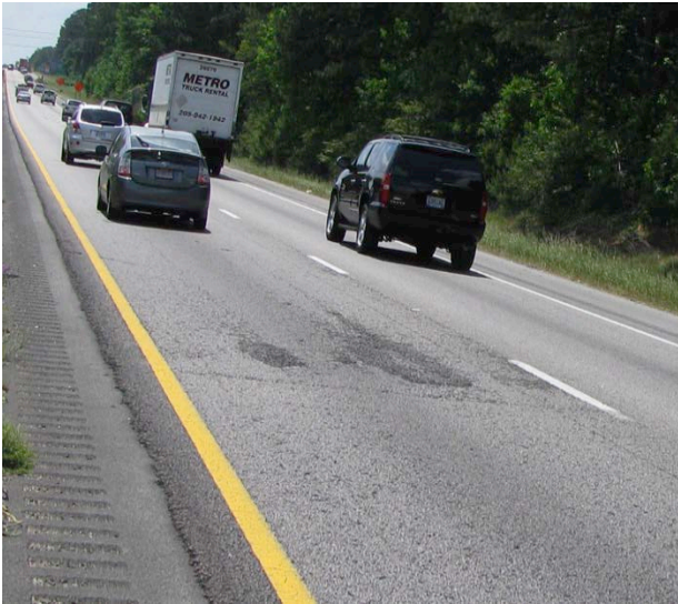
Cold Transverse Joint (a)
