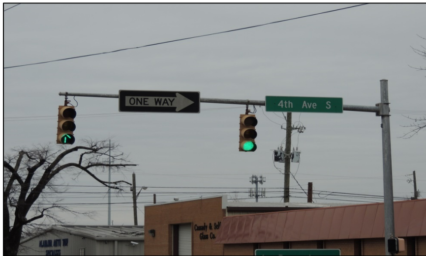
(b) GA + regular turn-prohibition sign, Birmingham AL
