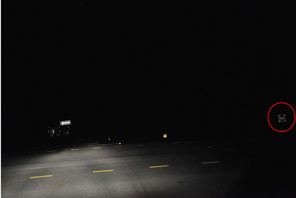
(b) Example of an improperly oriented sign in AL
