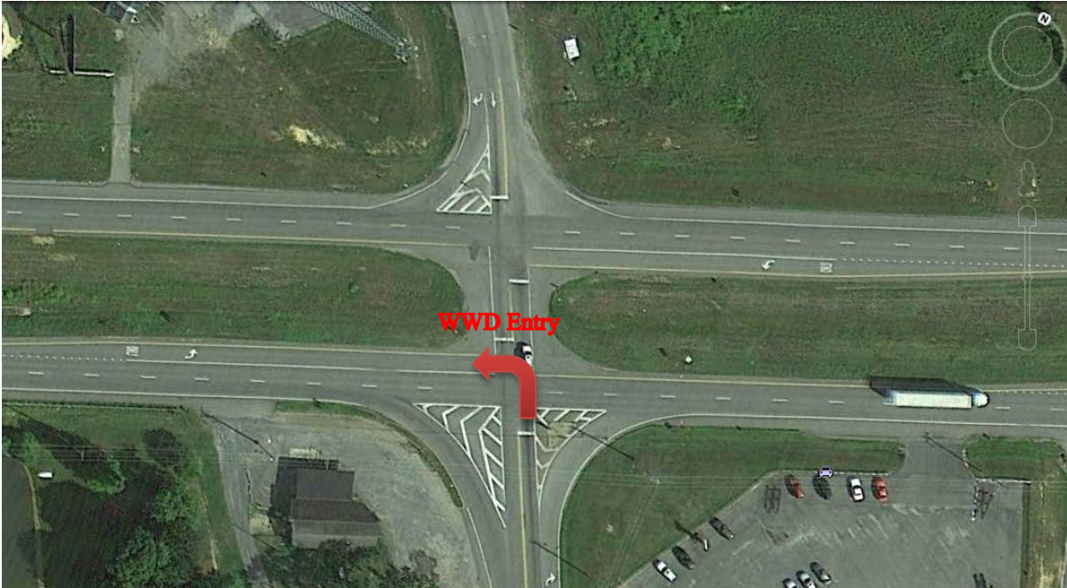
FIGURE 16 Unsignalized Intersection of AL Highway 75 (Divided Highway) and AL Highway 68 (Crossroad) in AL
