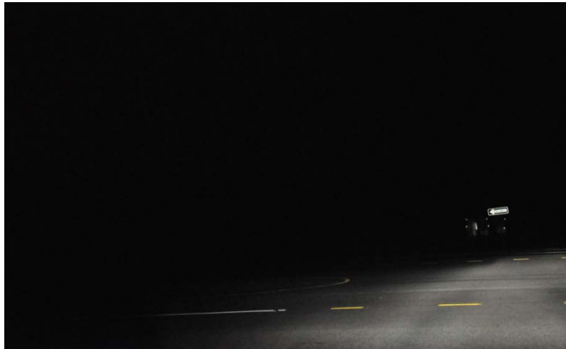
(c) Example of DO NOT ENTER signs placed too far from the nose of the median in AL
