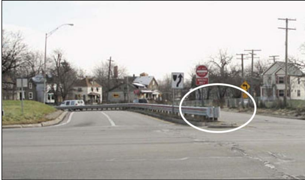
FIGURE 28 Median barrier blocking driver view of the entrance ramp
