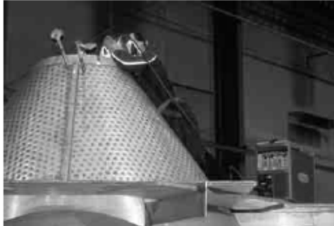
Fig. 19: Portable digital 270 A inverter power source being used in tank construction
