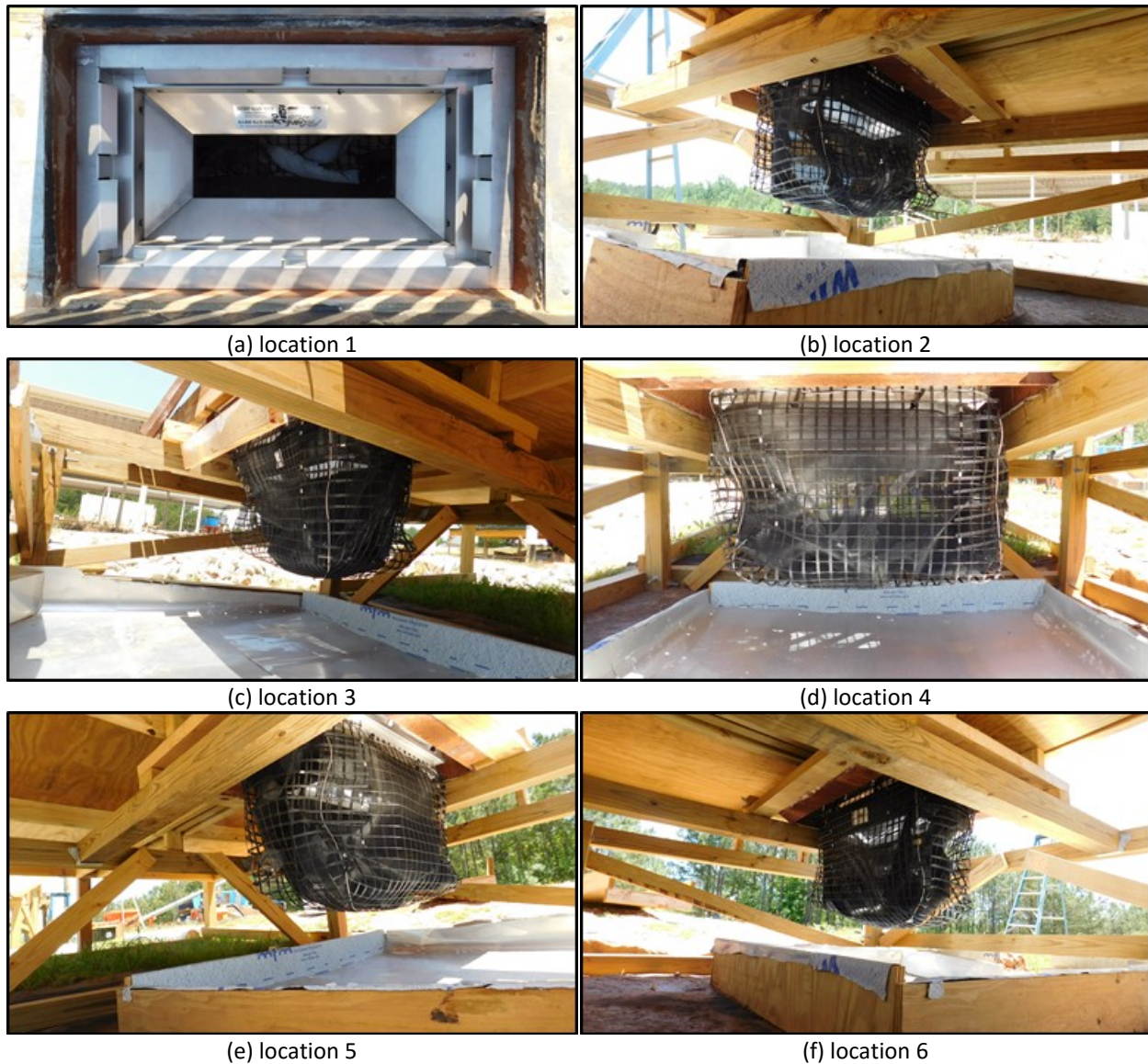
FIGURE 4.8 Pre-test installation for FloGard Plus.
