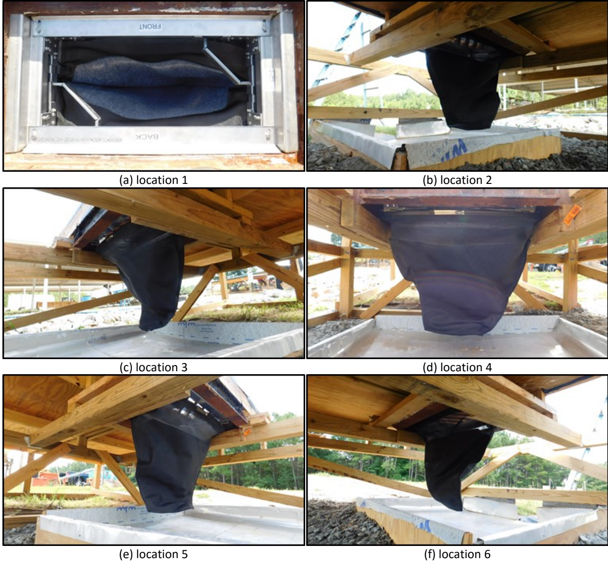
FIGURE 4.6 Pre-test installation for Flexstorm.
